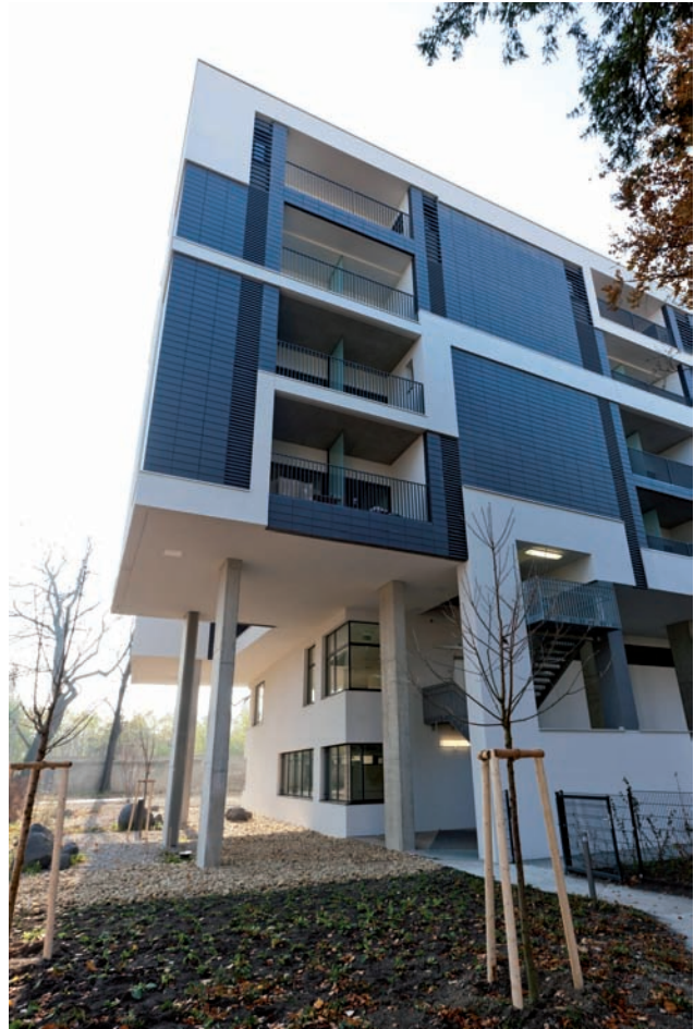
Top Floor Cantilever Image: PORR
