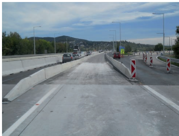
Traffic management in phase 2 – "island" construction site on the Vienna-bound carriageway Image: see below
