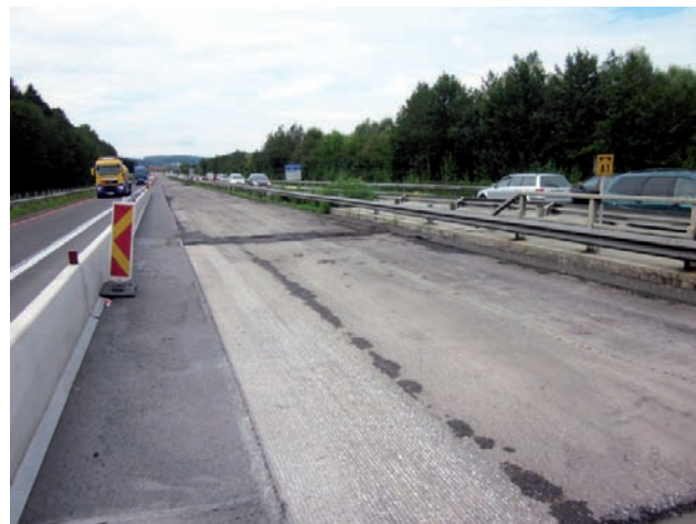
Grinding off of asphalt paving Image: PORR
