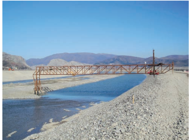
Structure for the bentonite matting "rollout" Image: PORR
