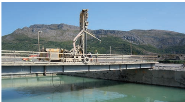
Bridge construction for Gewi piles Image: PORR
