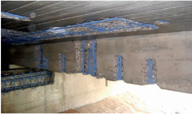
Bridge A1.00C – concrete repairs on the bottom side of the load-bearing structure
