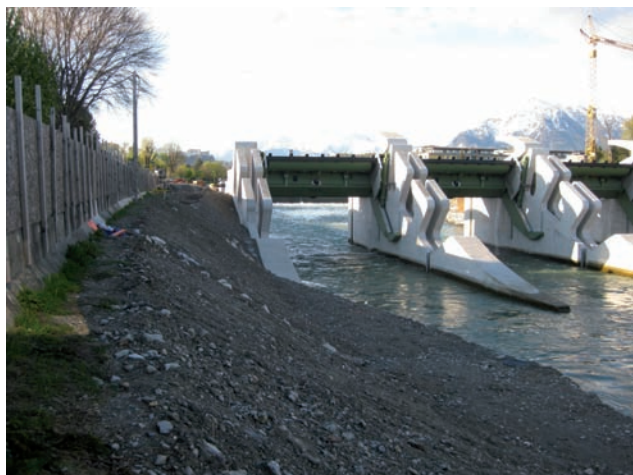
Construction phase 1 – weir gates 2 to 4, April 2012 Image: PORR
