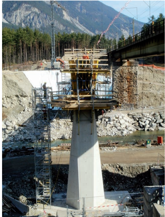
Reinforcement and formwork for pier on Bludenz side Image: PORR
