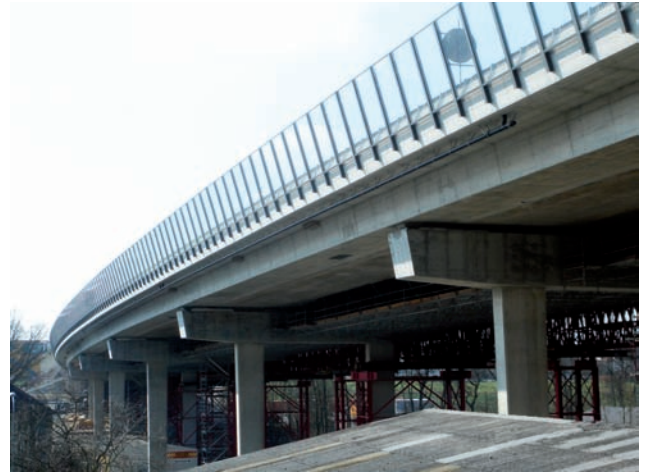
Widened south side with plexiglass noise barrier Image: PORR
