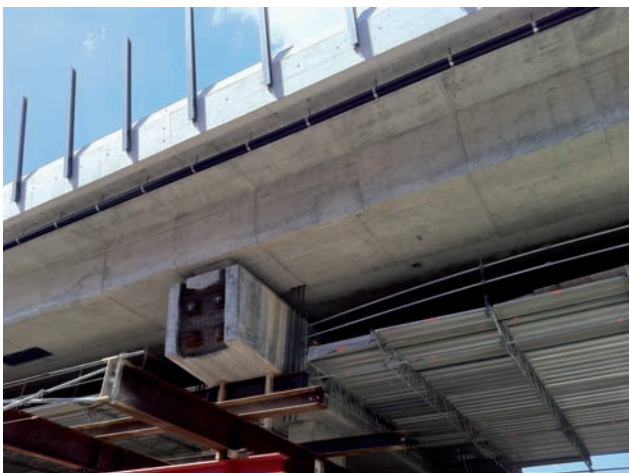
Anti-tilting structure on the transversal beam Image: PORR
