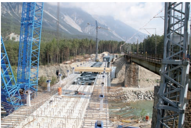
Preparing the steel-concrete composite structure Image: PORR
