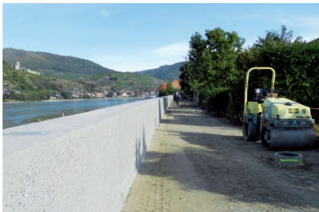
Wall with bush-hammered surface Image: PORR
