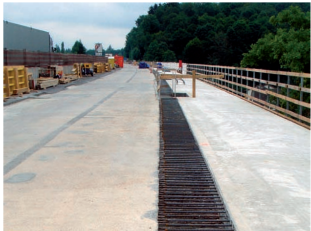
Upper joint gap Image: PORR
