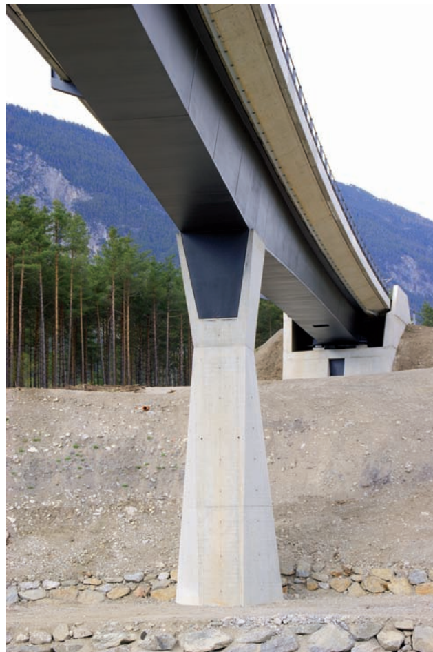
The hollow box girder and one pier seen from below Image: PORR
