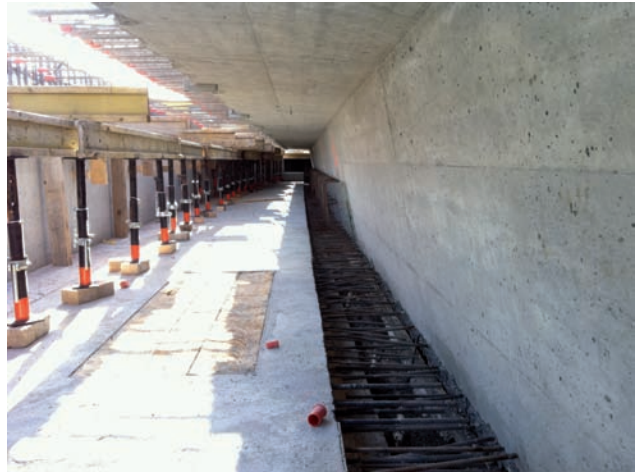
Lower joint gap Image: PORR
