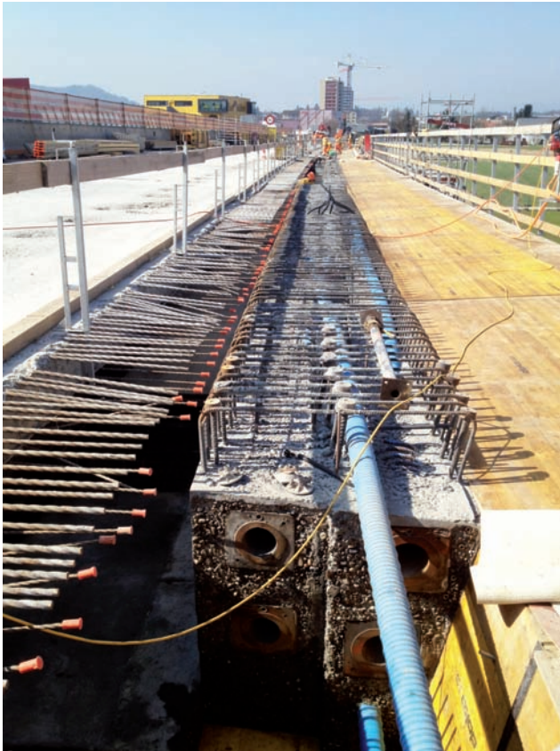
Hollow box girder Image: PORR
