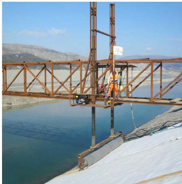
The rollout assembly in action Image: PORR
