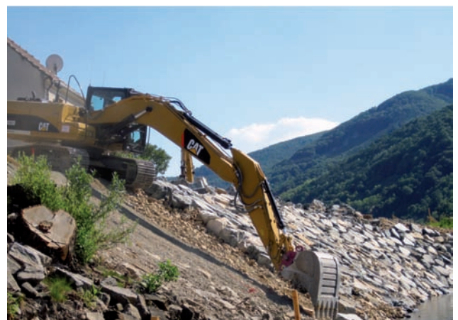
Embankment stabilisation works Image: PORR
