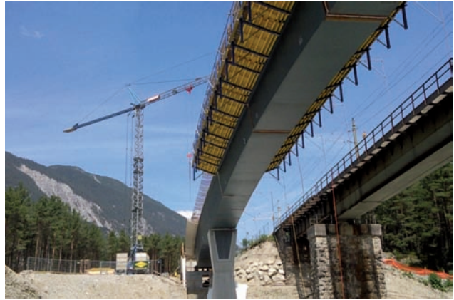
Travelling formwork for the composite structure, central section of the bridge Image: PORR
