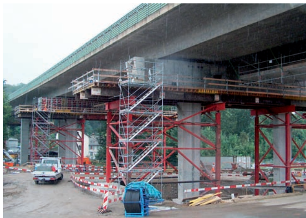
Transversal beams Image: PORR
