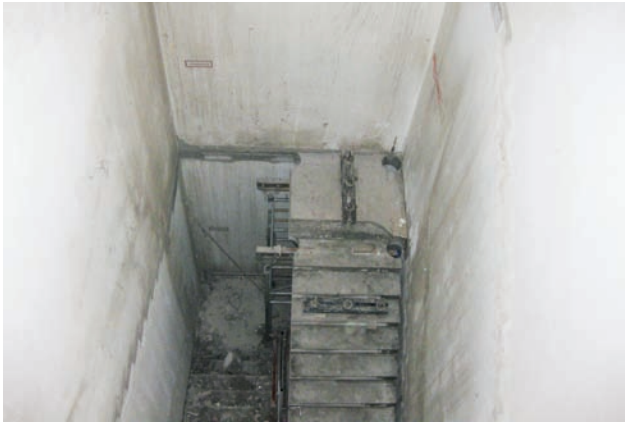
Dismantling of the interior escape staircase Image: PORR
