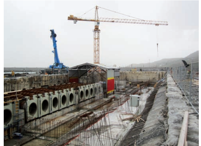
Installation of draft tubes Image: PORR
