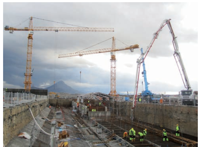
Concreting starts in the dry pit Image: PORR
