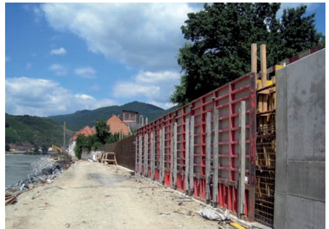
Shuttering at Oberarnsdorf Image: PORR
