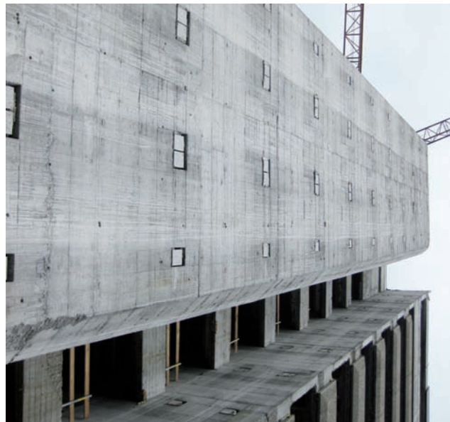
Dismantling of façade panels Image: PORR
