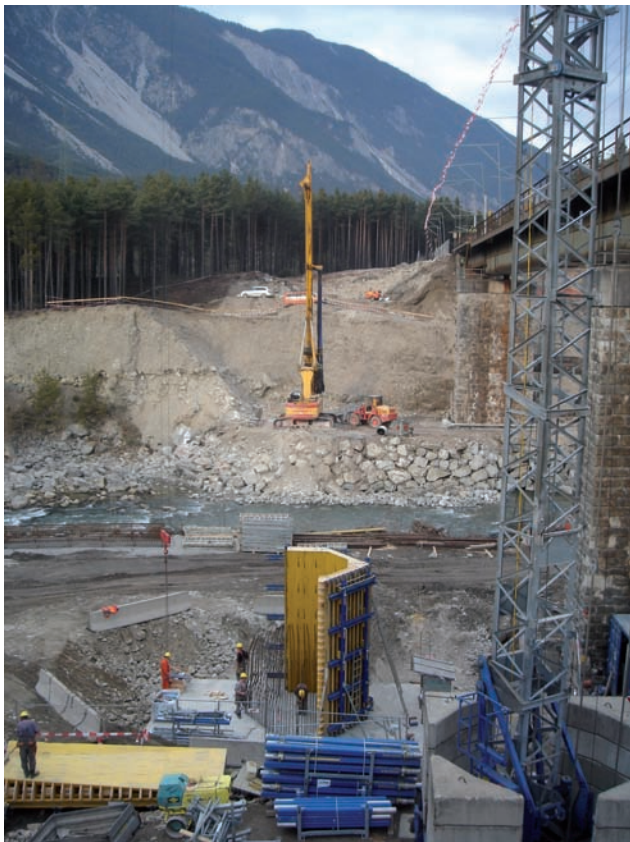
Driving of piles and formwork for pier concreting Image: PORR
