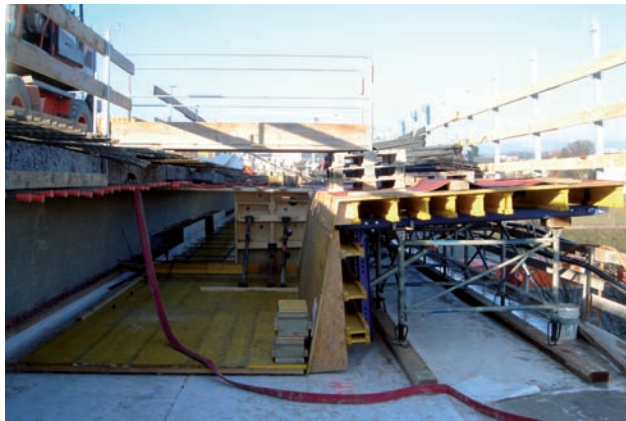
Box girder shuttering on the north side Image: PORR
