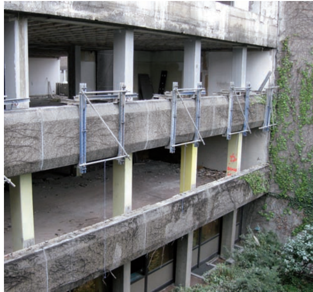
Dismantling of façade panels Image: PORR
