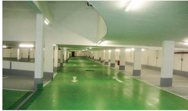
Finished UG level 2 with green surface coating Image: PORR
