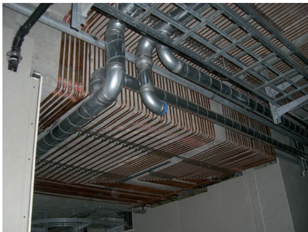
Copper pipes, medical gas supply Image: PORR
