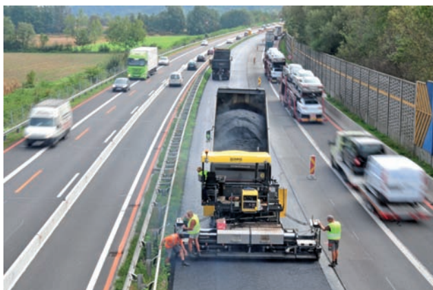
Asphalting in a cramped space Image: PORR
