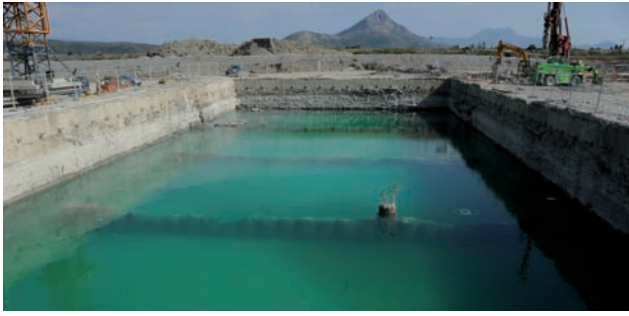
Construction pit before underwater concrete base casting Image: PORR
