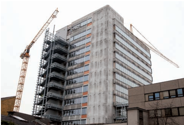
New structural steel fire escape Image: PORR
