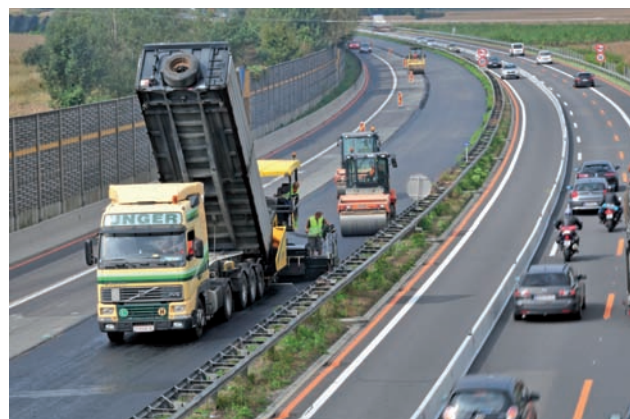
Renewal of asphalt paving Image: PORR
