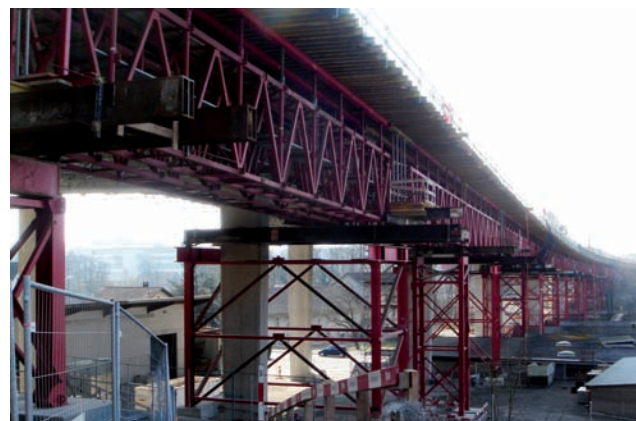
Centring for the box girder, north side Image: PORR
