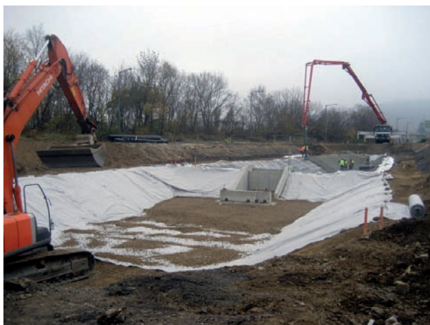
Water protection facility – concreting of settling basin, installation of filter bed Image: see below
