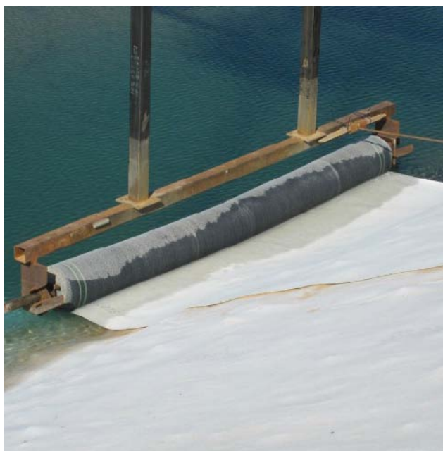
The rollout assembly in action Image: PORR
