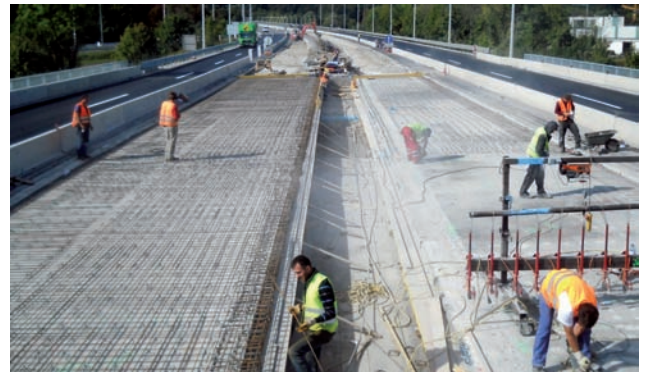
Bridge A1.00C – reinforcing grid for an additional concrete top course Image: see below
