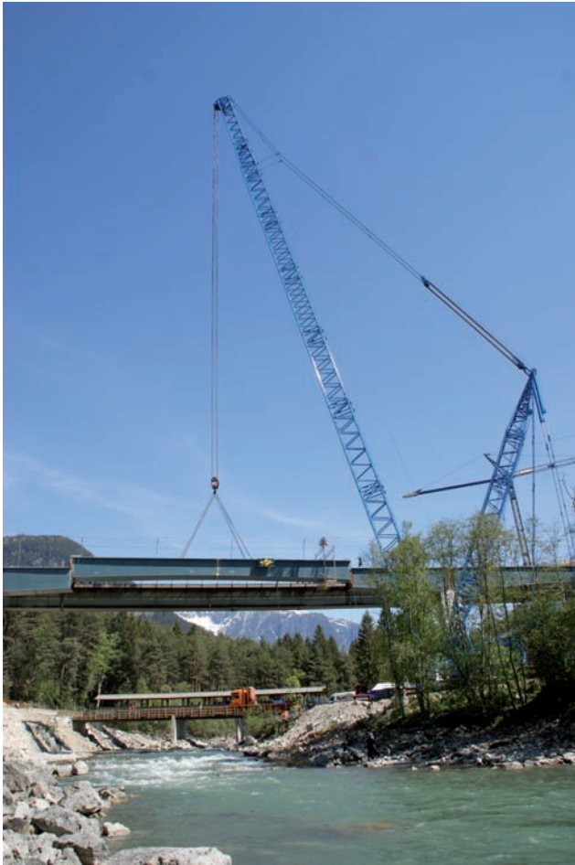
Positioning of the central section of the hollow steel box Image: PORR
