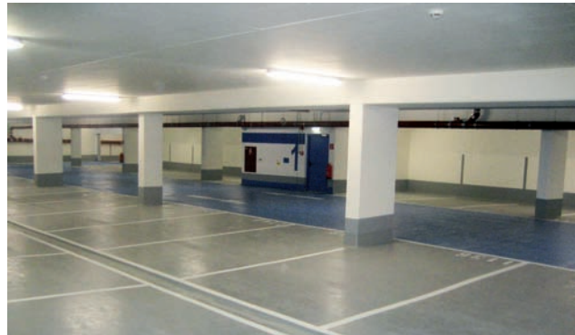
Finished UG level 1 with blue surface coating Image: PORR
