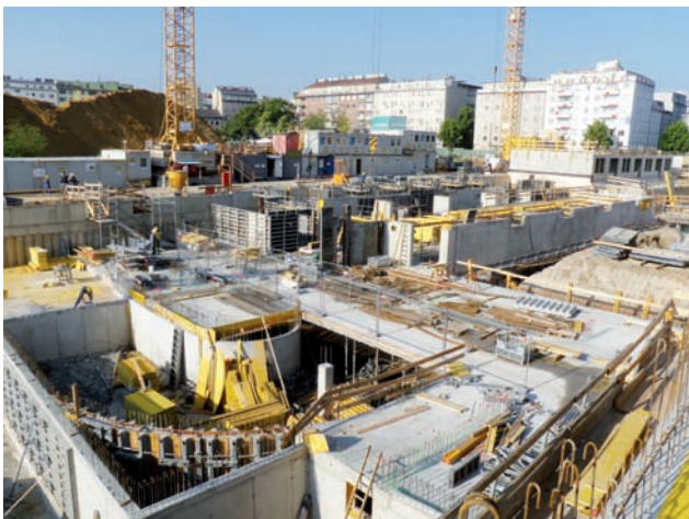
Reinforced concreting works to basement Image: PORR
