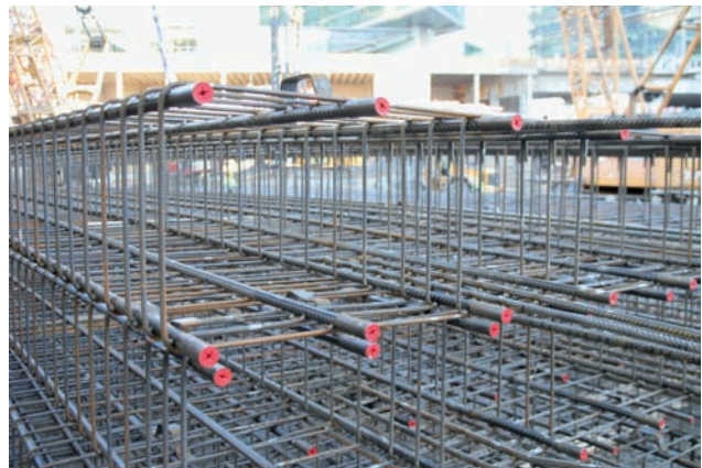
Diaphragm wall cage with threaded sockets Image: PORR
