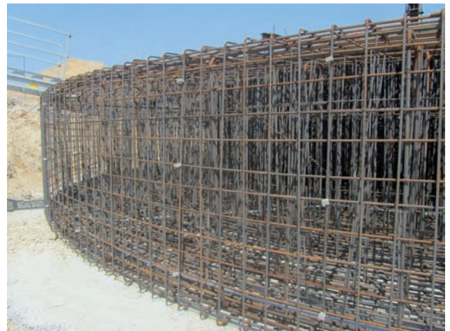
Completion of reinforcement cage Image: PORR
