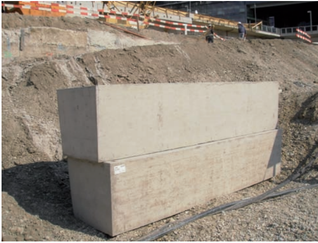
Guide wall extension Image: PORR
