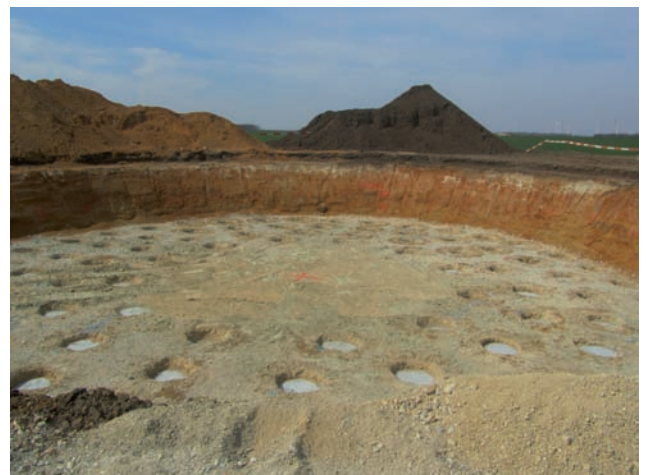
Concrete displacement columns Image: PORR
