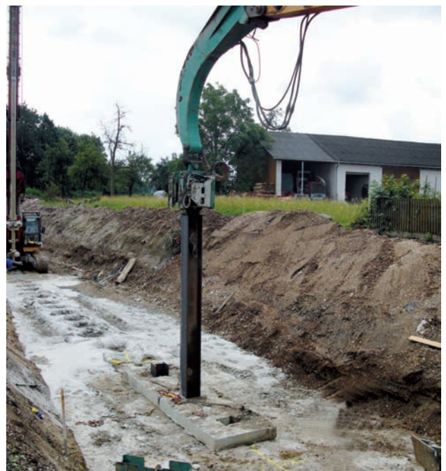
Vibration of rolled girders Image: PORR
