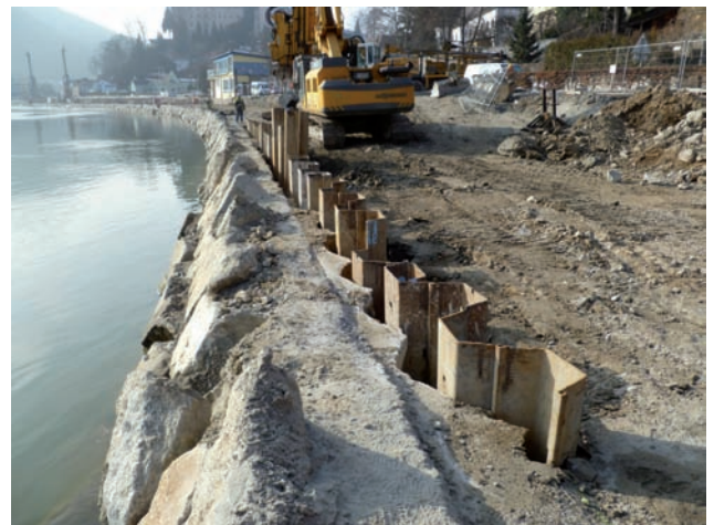
Sheet piling work Image: PORR
