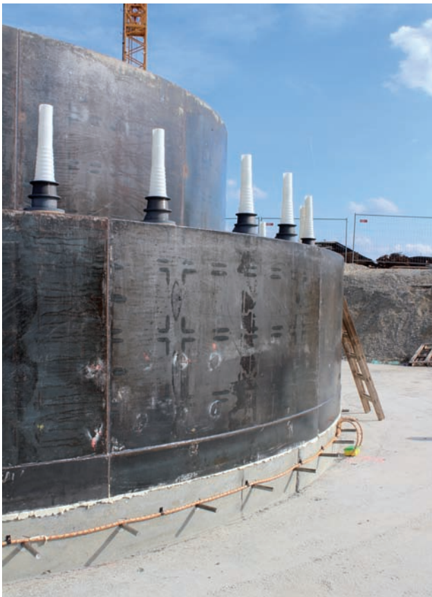
Compression tube around base slab Image: PORR
