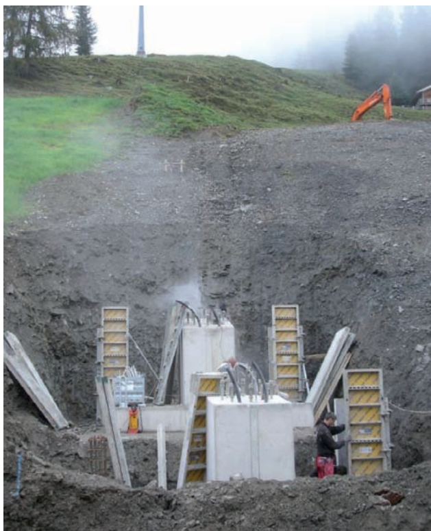
Completion work on support tower foundations near mid station Image: PORR
