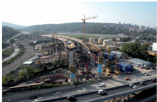
Casting of ICSRR structures with movable scaffolding system in September 2011 Image: PORR
