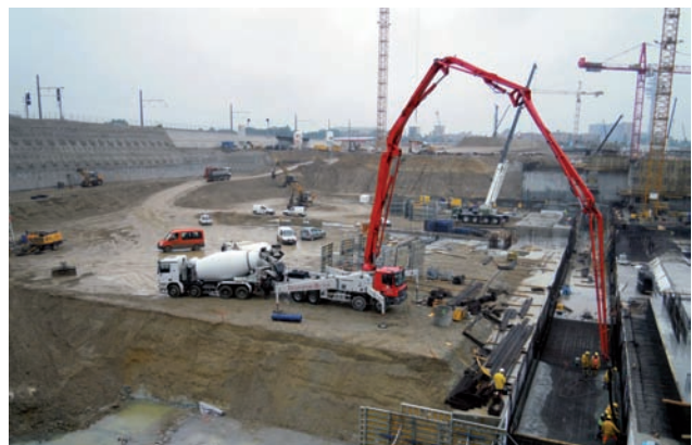
Works to raft foundation and M&E service corridors on third basement level Image: PORR
