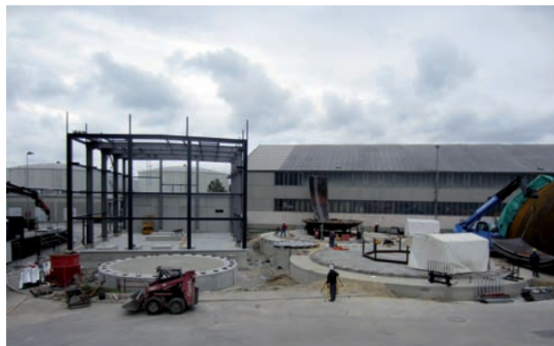
Current state of operations – concrete foundation works and steel construction completed Image: PORR
