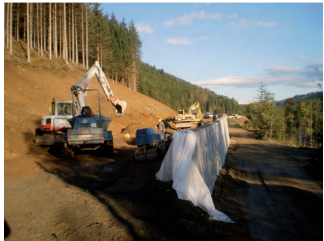
Backfilling of retaining wall and embankment construction Image: PORR
