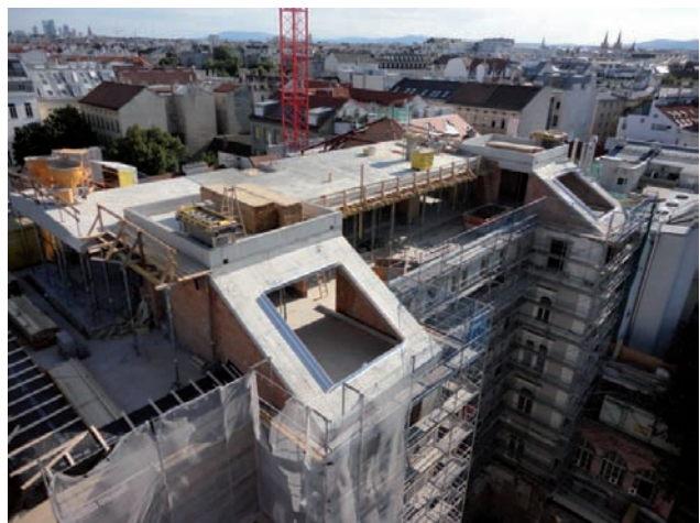
Garden side coffin lid shell construction Image: PORR
