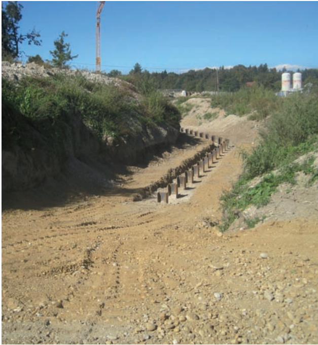
Finished MIP wall with rolled girders Image: PORR
