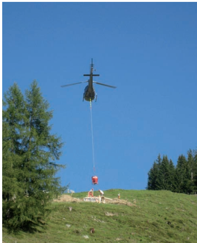
Concreting work on a support tower foundation with the aid of a helicopter Image: PORR
