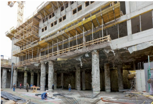
Temporary CFA piles with parts of upper shell already under construction Image: PORR
