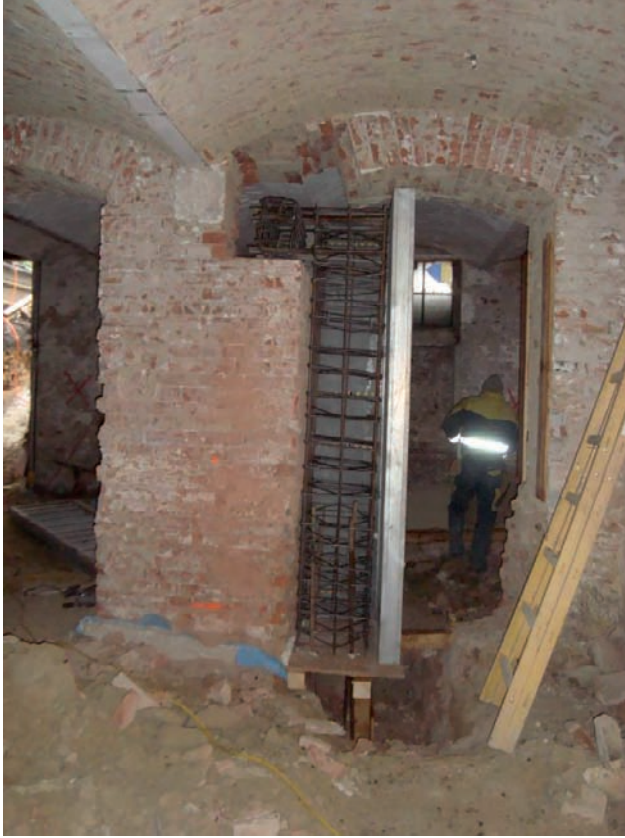
Construction of reinforced concrete columns Image: PORR
