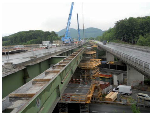
Demolition of existing structure Image: PORR
