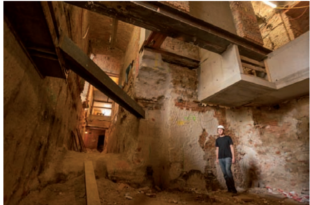
Underpinning structures in basement Image: PORR
