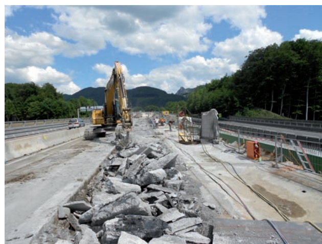
Demolition of bridge superstructure Image: PORR
