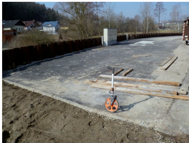
Visible sheet piling Image: PORR
