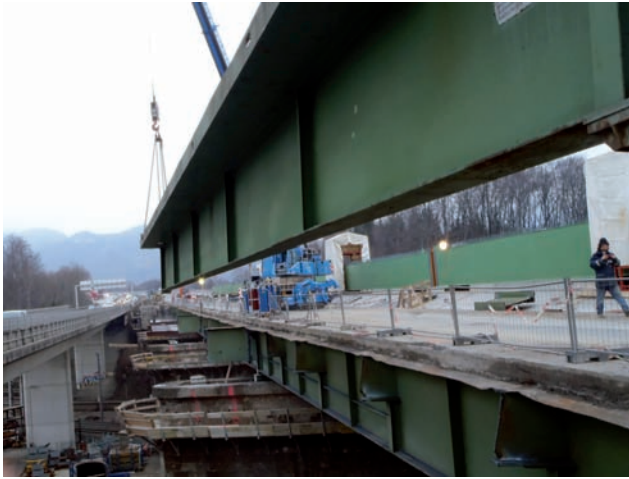
Removal of existing girders Image: PORR
