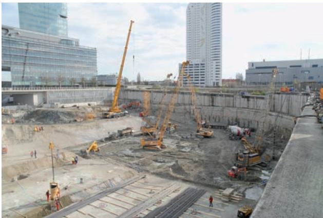
Diaphragm wall construction Image: PORR
