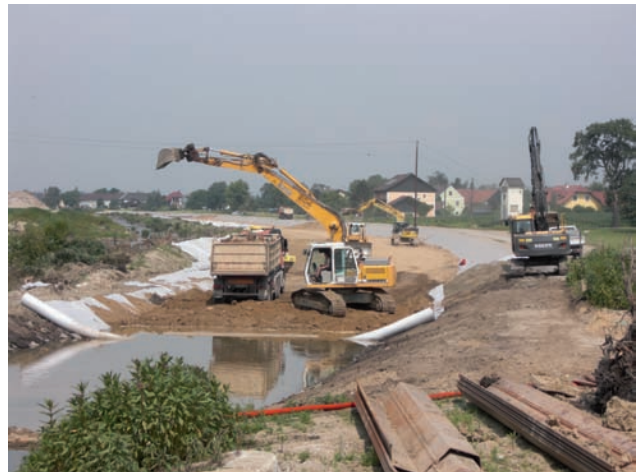
Incorporation of blast debris material Image: PORR
