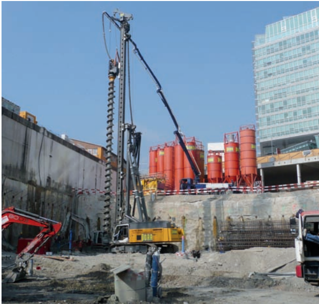
Augered cast-in-place pile Image: PORR
