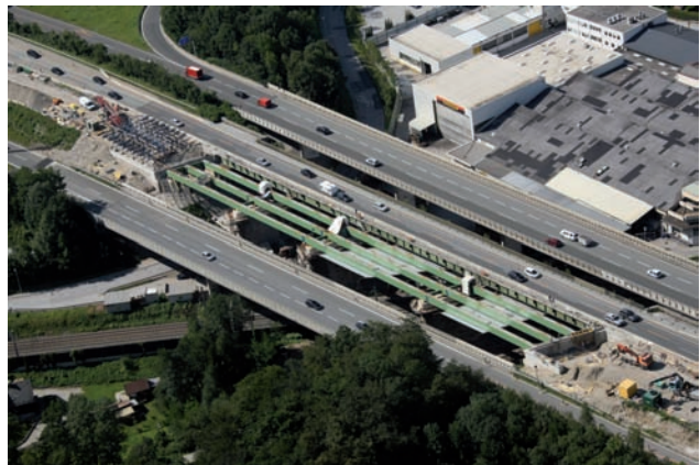
New steel structure for the Vienna-bound carriageway Image: LBS Redl
