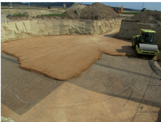
Installation of load-distribution matting Image: PORR
