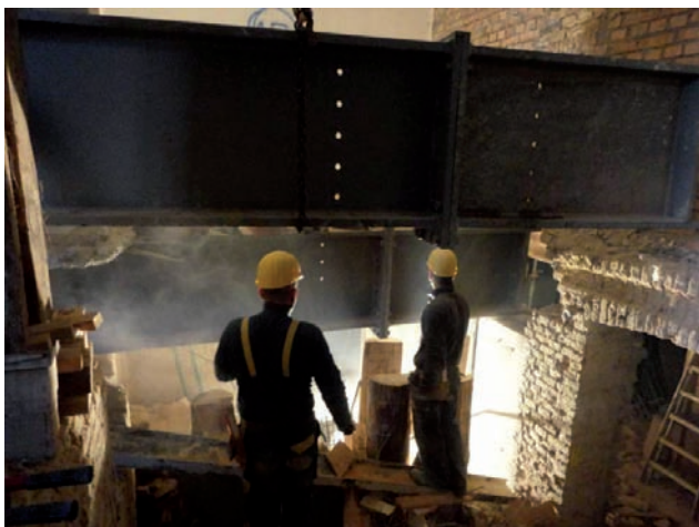
Installation of underpinning structures Image: PORR
