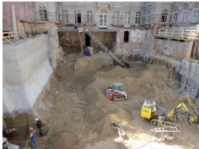
Stabilisation of foundation pit Image: PORR
