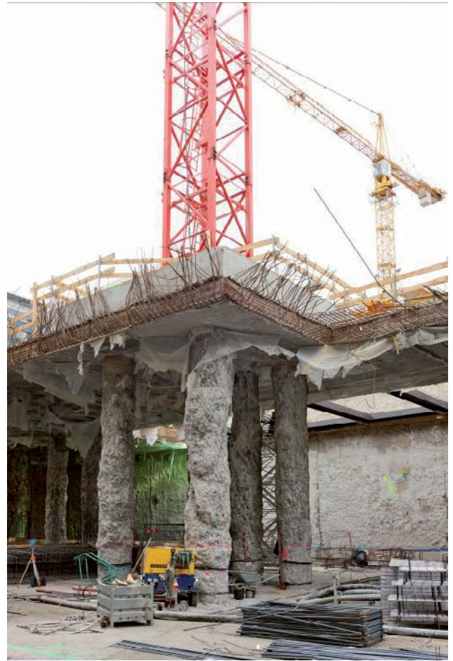
Temporary CFA piles for tower crane Image: PORR
