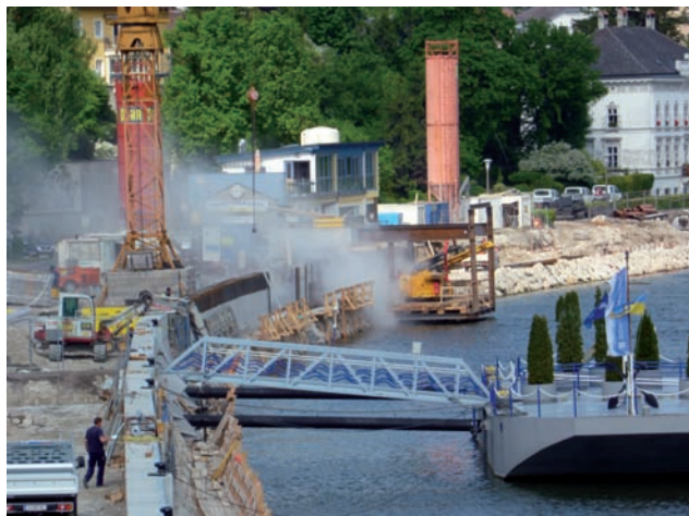
Creation of Gewi anchors with staging as drilling platform Image: PORR
