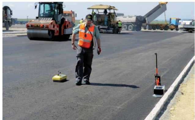
Quality control with nuclear density gauge Image: ASFINAG
