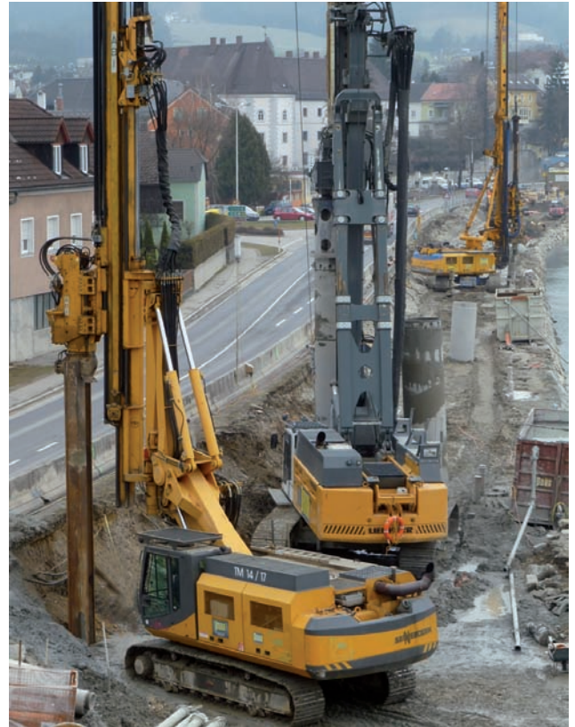
Auger pile and sheet piling work Image: PORR
