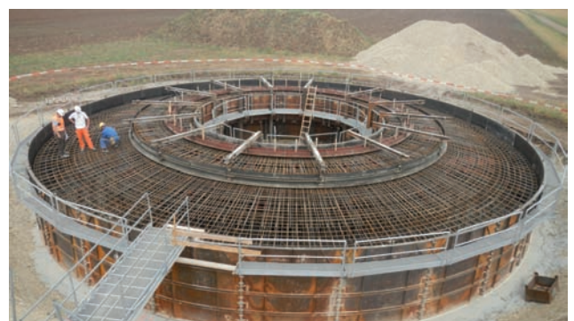
Reinforcement + outer casing completed Image: PORR
