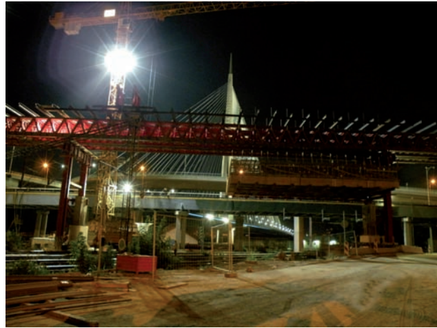
Elevated casting of superstructure above track installation Image: PORR
