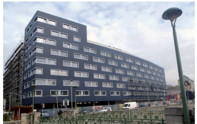
Eternit fibre-cement rainscreen cladding Image: PORR
