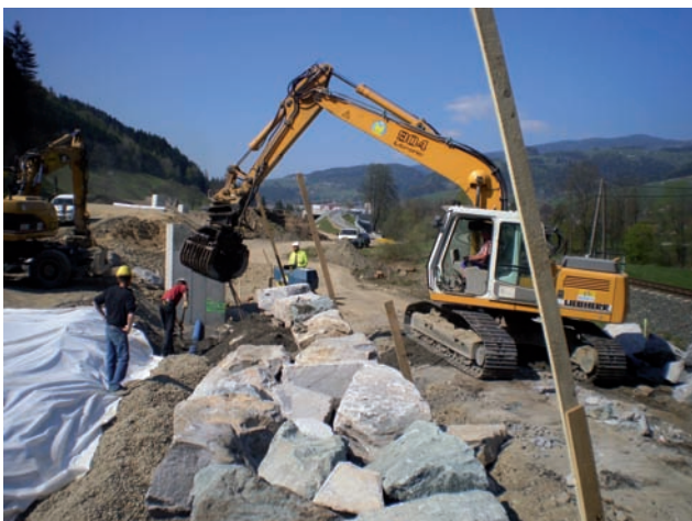
Drainage and channel laying during stone wall construction Image: PORR
