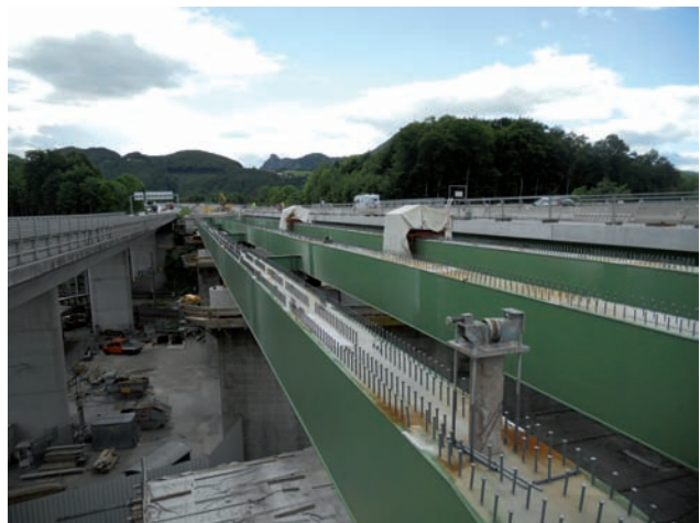
New steel structure for the Munich-bound carriageway Image: PORR
