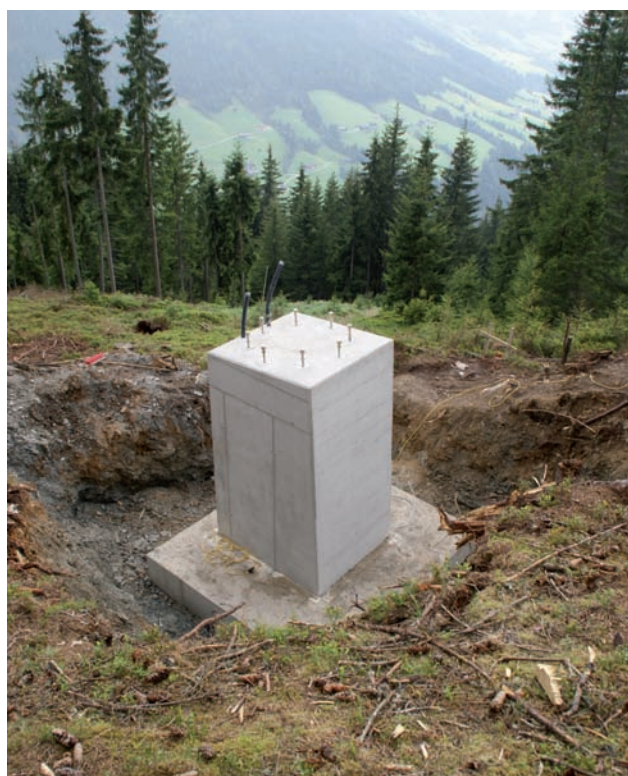
Completion work on support tower foundation no. 16 Image: PORR
