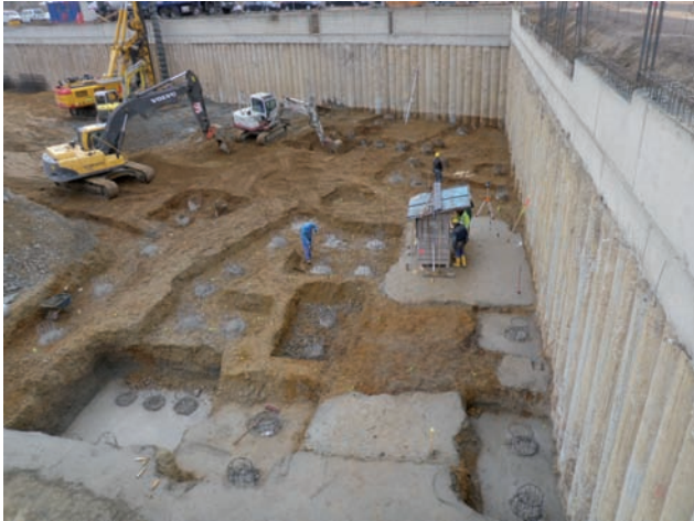
Installation of deep-foundation piles Image: PORR
