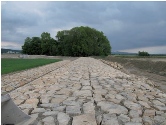
Finished overflow section Image: PORR
