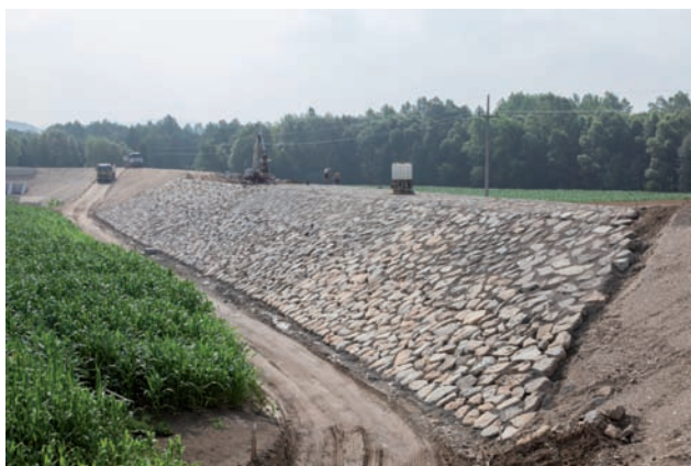
Saxen Süd dam with overflow section Image: PORR
