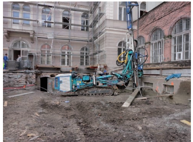
Jet grouting in the garden Image: PORR
