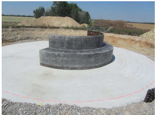
Start of inner formwork assembly Image: PORR
