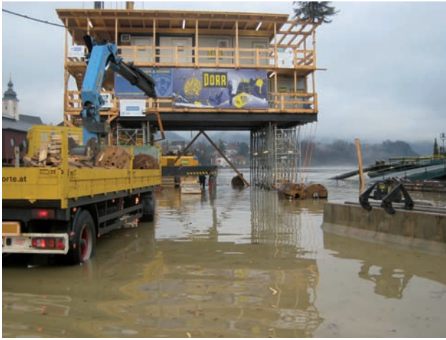
Building site disposition on scaffold towers at high water Image: PORR
