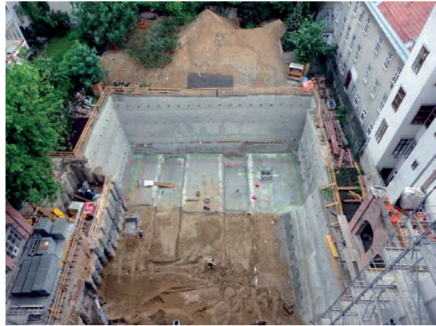
Stabilisation of foundation pit Image: PORR
