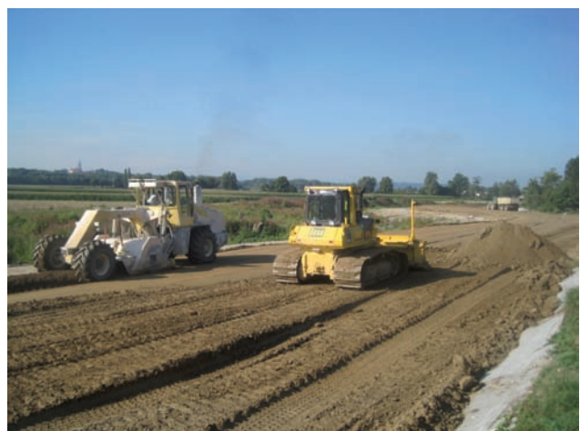
Soil mixing in the mixed in place procedure Image: PORR
