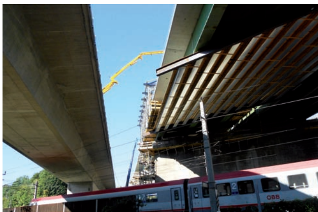
Protective scaffolding over Westbahn railway line Image: PORR
