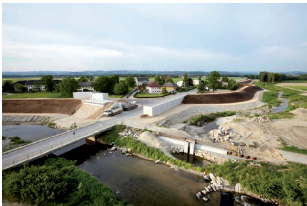
Pumping station 1 with HWP wall, Labing Image: Photo studio Wurst
