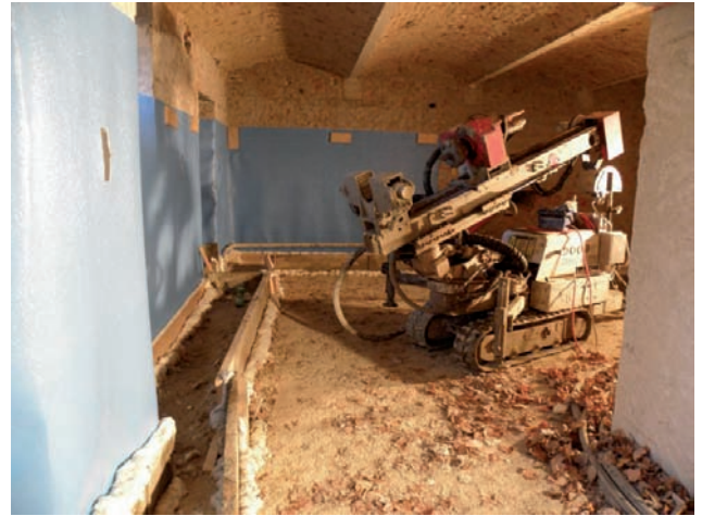
Jet grouting in basement Image: PORR
