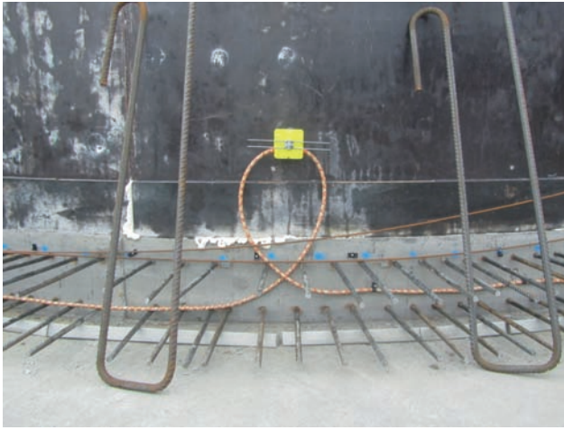
Compression tube - Detail protective box Image: PORR
