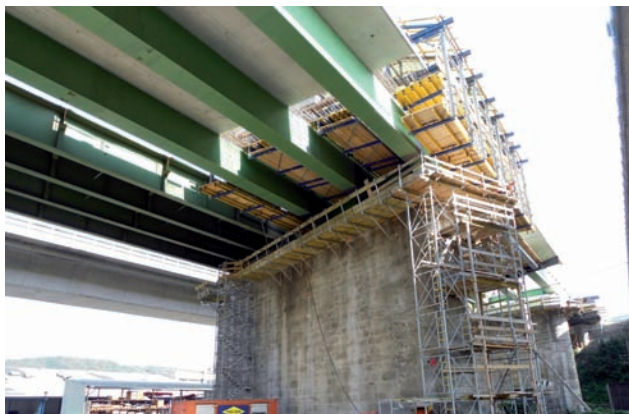
Formwork carriage for the composite structure Image: PORR
