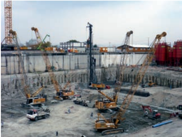
Concentrated machinery deployment for the production of the slotted wall barrette of the Donau-City Tower 1 with up to 40 m depths Image: PORR
