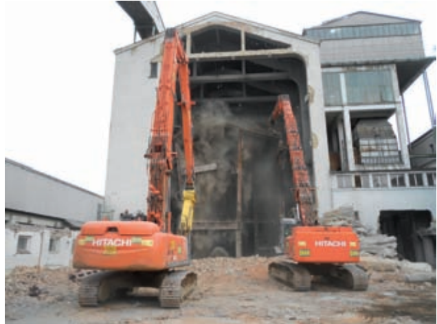
Dismantling the boiler, Boiler House Block 1+2 Image: PORR
