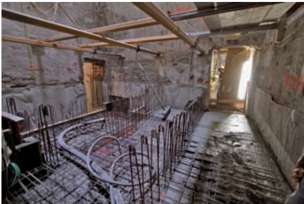
Reinforced concrete work inside building Image: Irene Schanda
