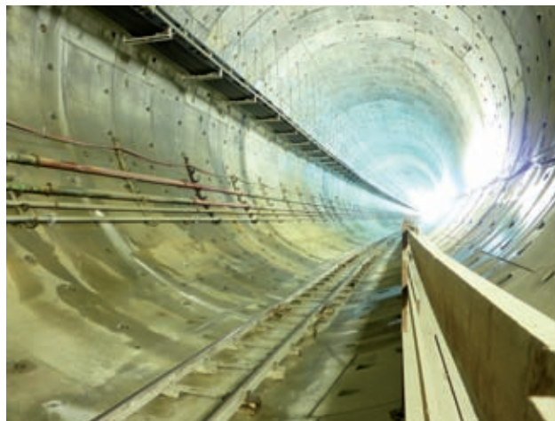
Tunnel tube with segmental lining Image: PORR
