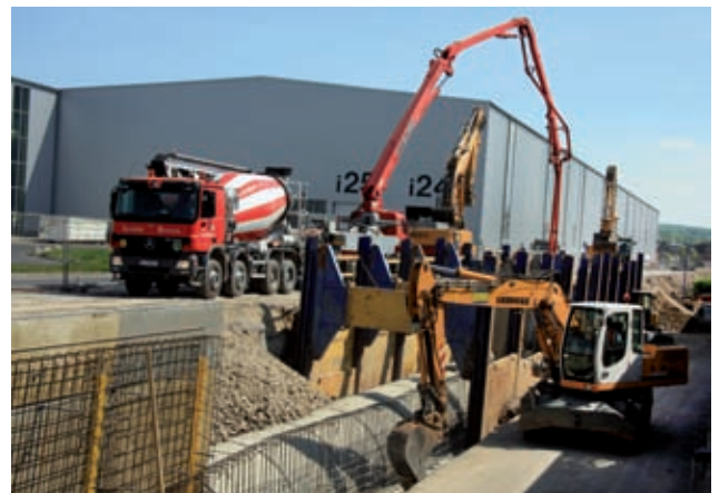
Construction of the mounted retaining wall Image: PORR
