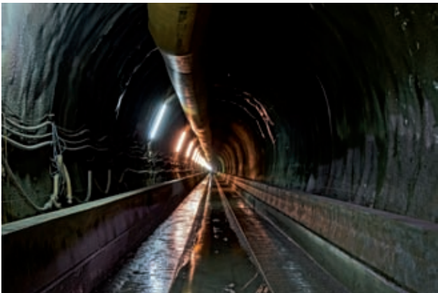
Invert gutter production after four of five working steps Image: PORR
