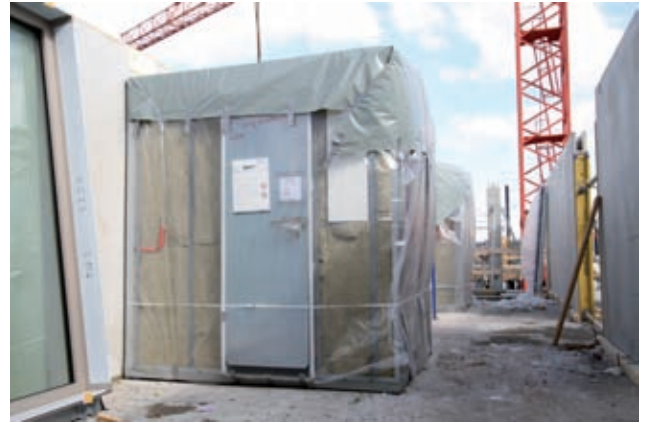
Installation of pre-fabricated bathroom units Image: PORR
