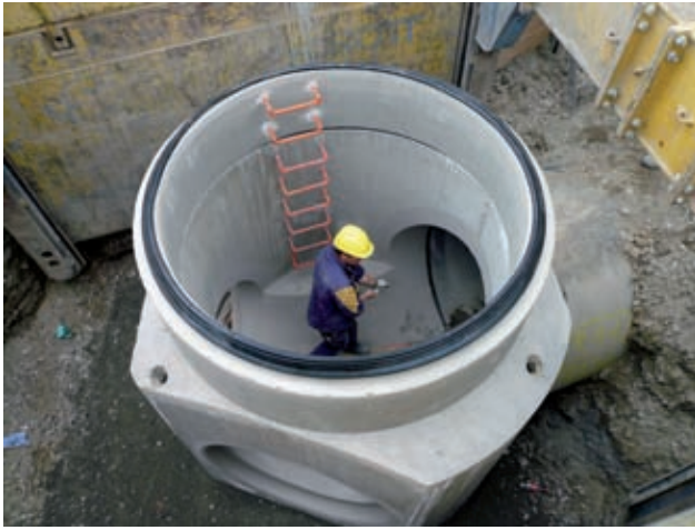
Manhole base DN2000 with DN1600 main channel Image: PORR
