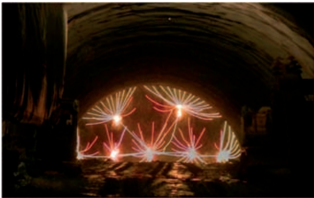
Blasting a heading face Image: PORR
