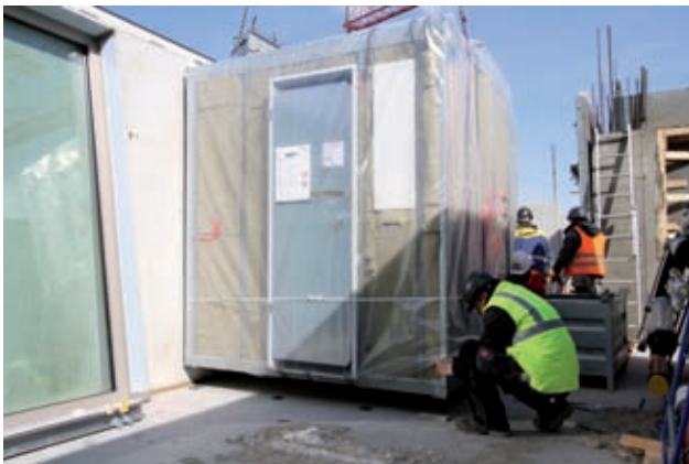
Installation of pre-fabricated bathroom units Image: PORR
