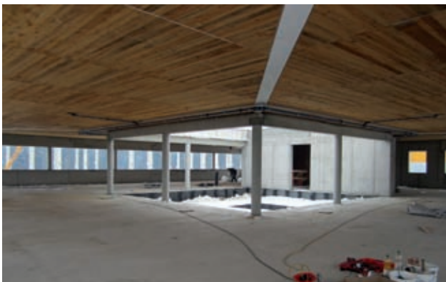
Lightweight timber roof, 2nd floor Image: PORR
