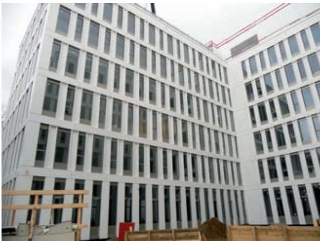
Office component, modular and sheet metal façade Image: Alu-Sommer
