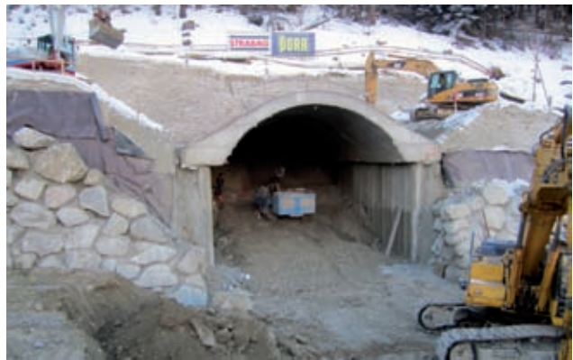
Cut-and-cover method and bore piles at the Ampass portal Image: PORR
