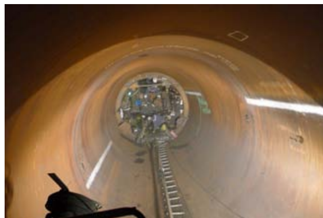
Illustration 10: Penstock construction, inner lining with armoured steel Image: PORR
