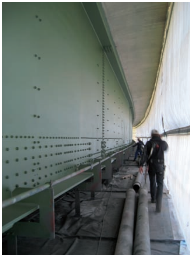
Coating system 3 after the last deck-layer Image: PORR
