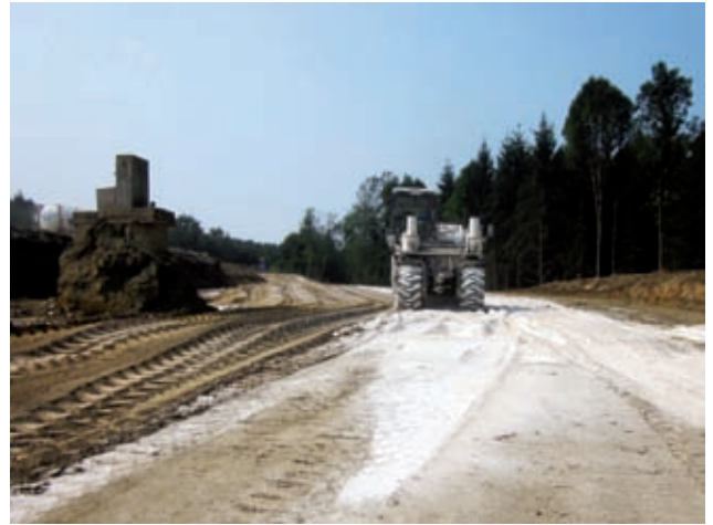
Soil stabilisation Image: PORR
