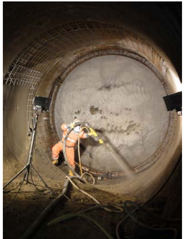
Shotcrete strengthening – cross heading under icing Image: PORR
