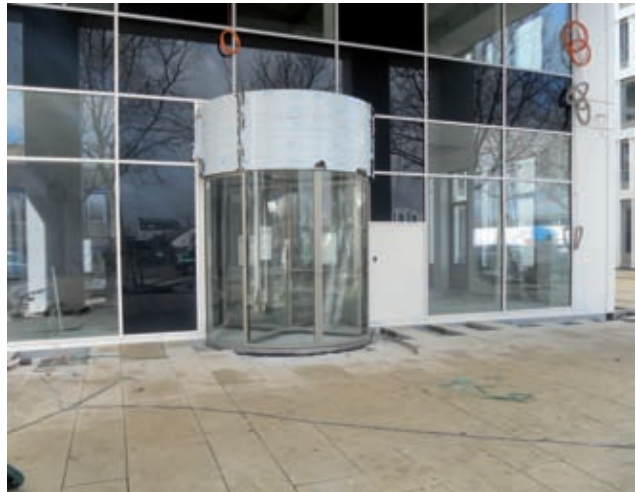
Post and beam façade with revolving door Image: Alu-Sommer
