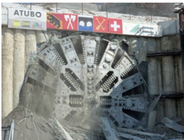
Breakthrough of Längholz tunnel tube, east Image: PORR
