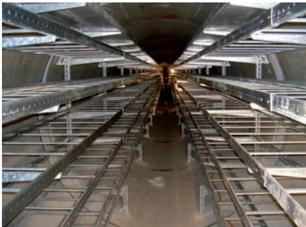
Inside the 30 kV E-collector DN2600 Image: PORR
