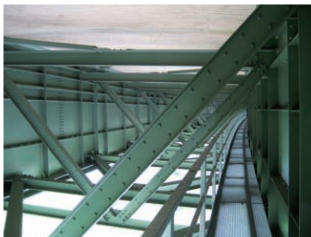
Completion corrosion protection work – inside steel structure with inspection gangway Image: PORR
