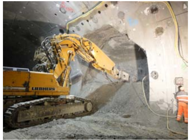
Excavation of cross heading 3 Image: PORR
