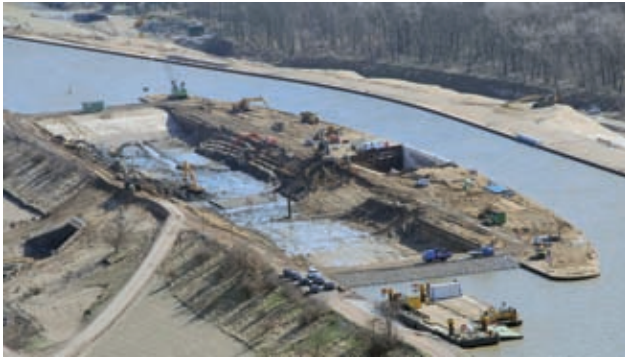
Stripping away the soil to demolish the existing tunnel, March 2012 Image: J. Bunte
