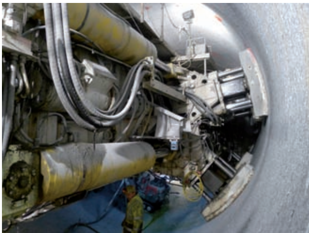
Illustration 5: Pressure gallery with machine tunnelling, feed cylinders (yellow) and gripper Image: PORR
