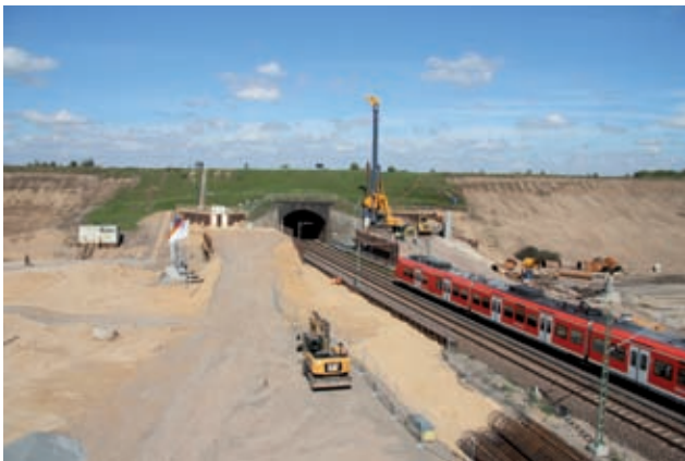
Working level with production of the bore pile wall, September 2010 Image: PORR
