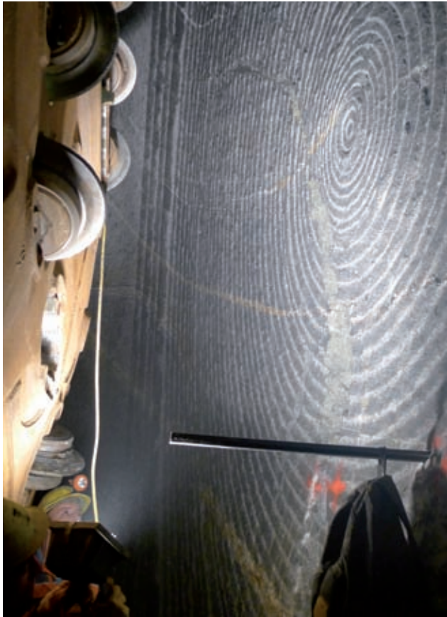
Illustration 4: Pressure gallery with machine tunnelling, chisel marks on the heading face Image: PORR
