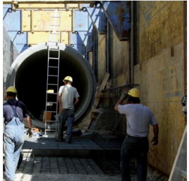
Standard cross-section DN2400 in MEGA double slide rail shoring Image: PORR
