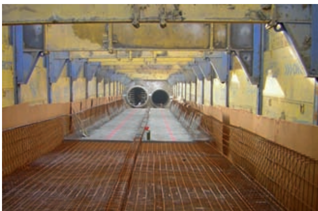
Standard cross-section DN2600/DN2200 in MEGA double slide rail shoring Image: PORR
