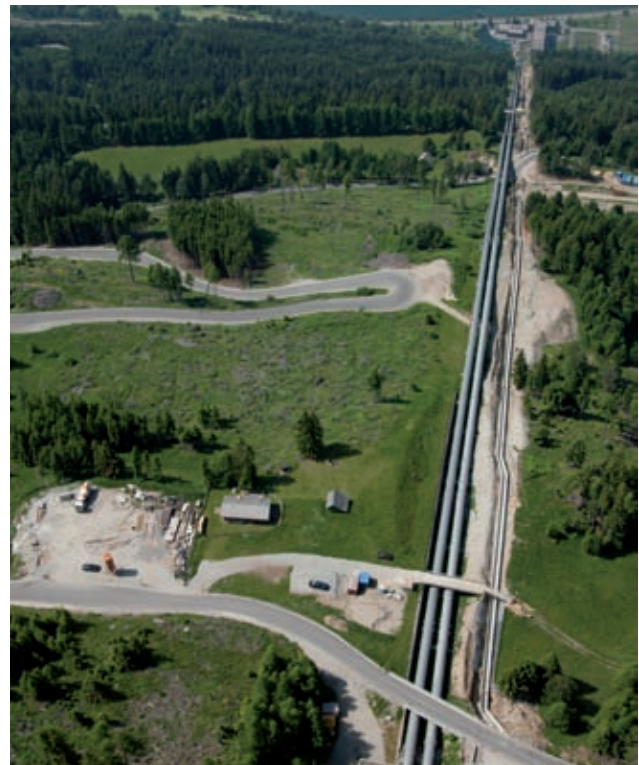
Illustration 14: Power transmission along the existing pressure pipeline, supply via the aerial railway Image: PORR
