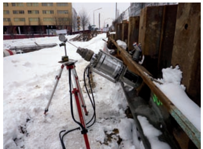
Tensioning of the anchor is performed with a standard tensioning press and short tie rods which can be easily removed on dismantling of the anchor head. Image: PORR
