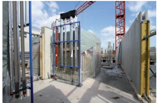
Installation of pre-fabricated bathroom units Image: PORR
