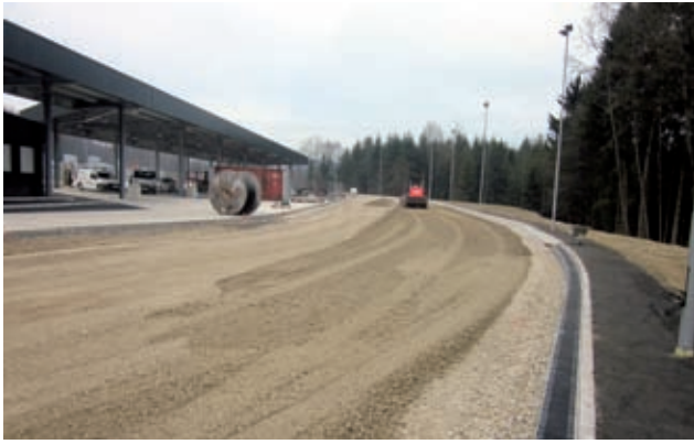
Loose upper base course with projecting roof Image: PORR
