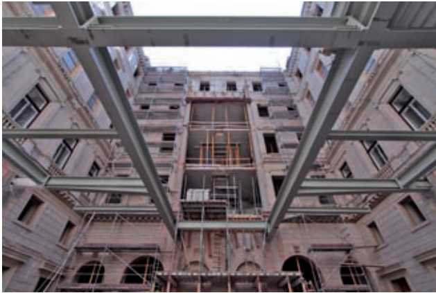
Steel construction for courtyard roofing, incl. lift tower Image: Irene Schanda
