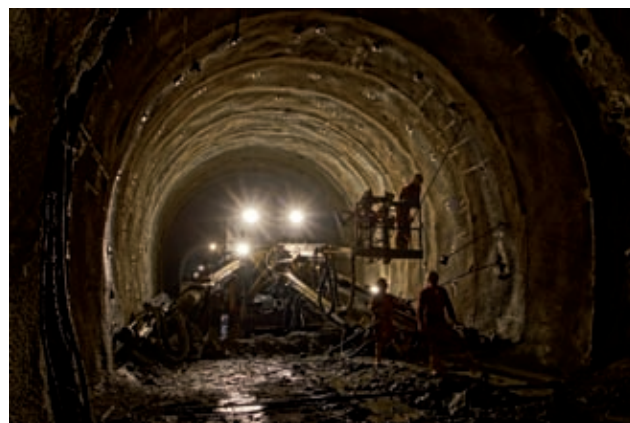
Anchor works Image: PORR
