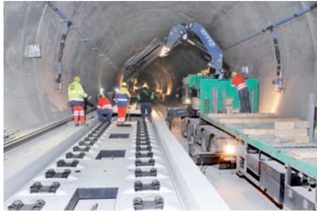
Installation of track support slabs Image: PORR
