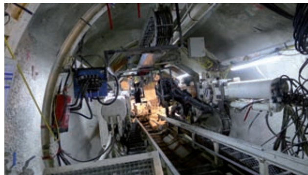
Illustration 9: Excavation of penstock, shaft-sinking, 42° gradient Image: PORR
