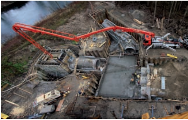
Culvert and distributor structures Image: PORR
