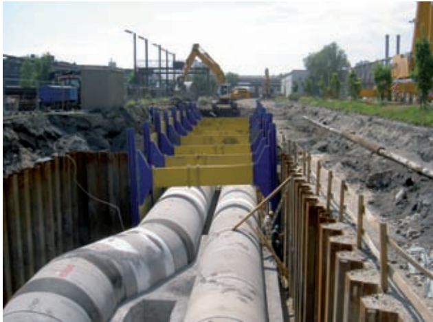
Transition from a sheet pile wall to MEGA double slide rail shoring Image: PORR
