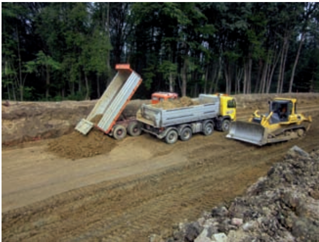
Soil stabilisation Image: PORR
