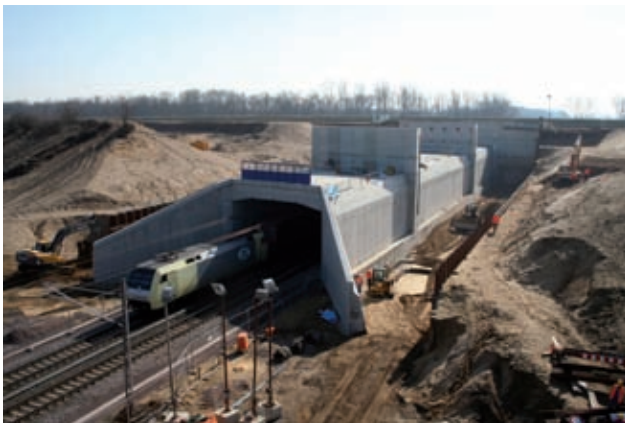
Construction pit and frame structure of the second construction stage, March 2013 Image: PORR
