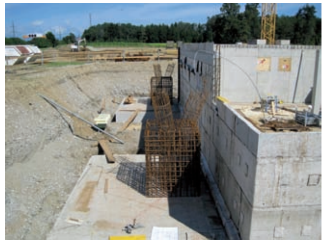
Reinforcement for supports Image: PORR
