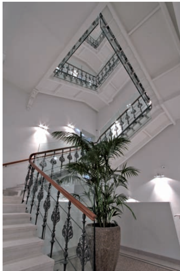
Historical staircase – with restored banisters, glass panels and underpinning of original wedge steps Image: Irene Schanda
