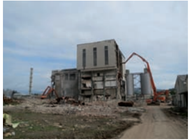
Hitachi 870 boiler dismantling Image: PORR
