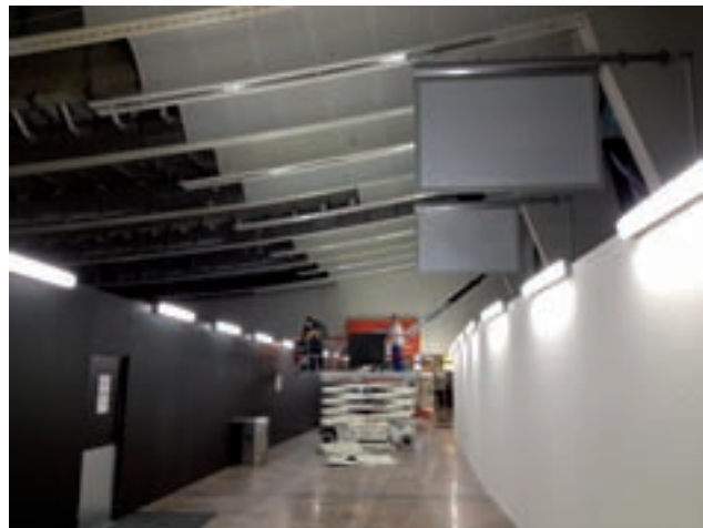
Dismantling of the existing ceiling on the night shift (Links: Dust protection wall, Construction section 1, Right: Dust protection wall, Construction section 2) Image: PORR
