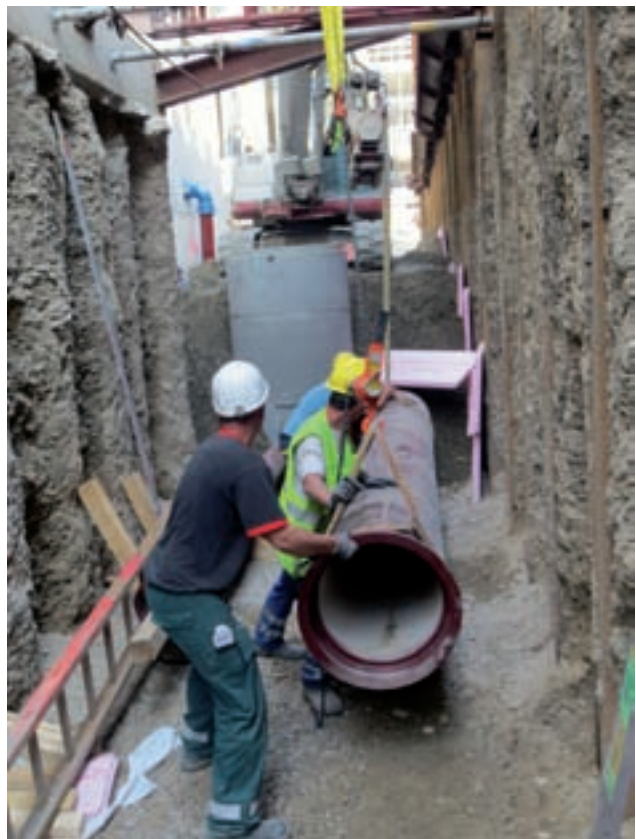
Laying of the drainage Image: PORR
