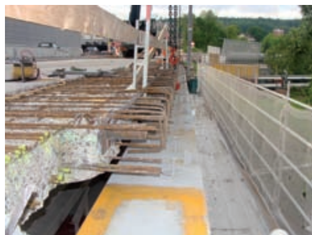
Reinforcement and renovation of the Lehen Viaduct Image: PORR
