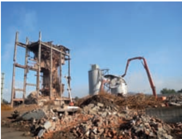
Hitachi 870 boiler dismantling Image: PORR
