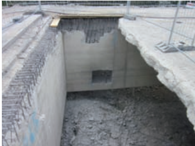
Surface removal work, preparation for pre-stressing measures, P44 abutment Graz Image: PORR
