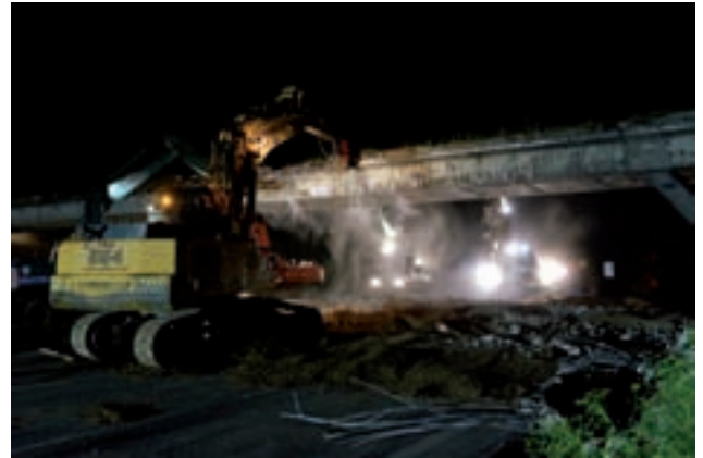
Night-time bridge demolition Image: PORR
