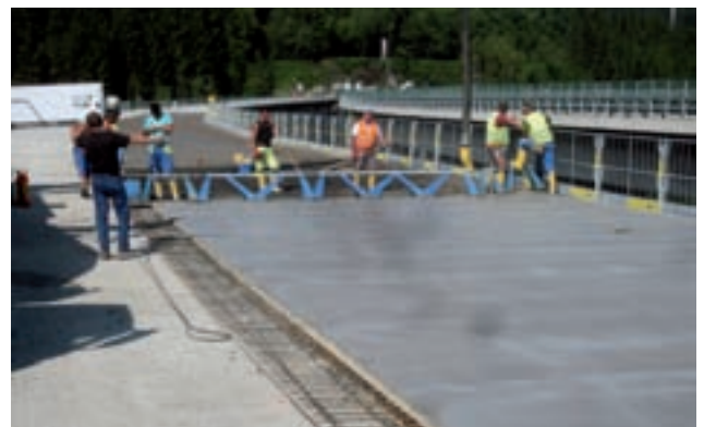
Concreting top cover of P46 Image: PORR
