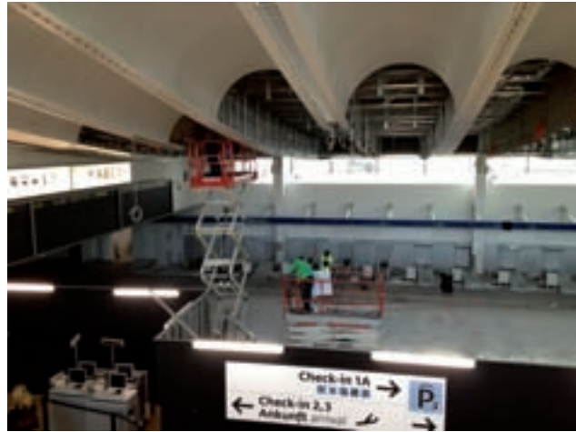
Dismantling of the existing ceiling with the aid of scissor-lift work platforms Image: PORR
