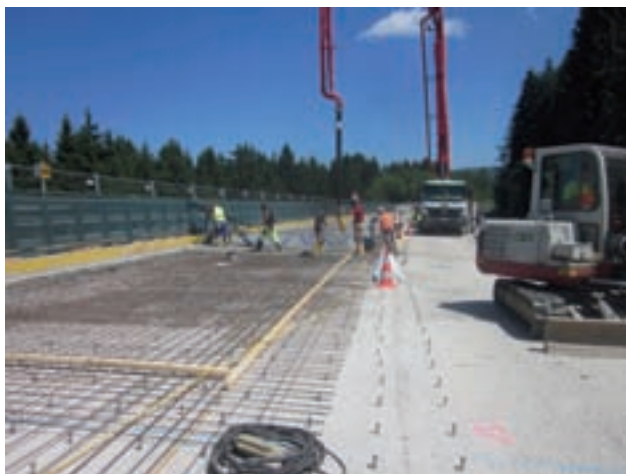
Concreting top cover of P45 Image: PORR
