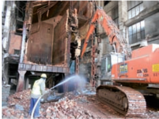
Picture 4: Boiler dismantling within building shell Image: PORR
