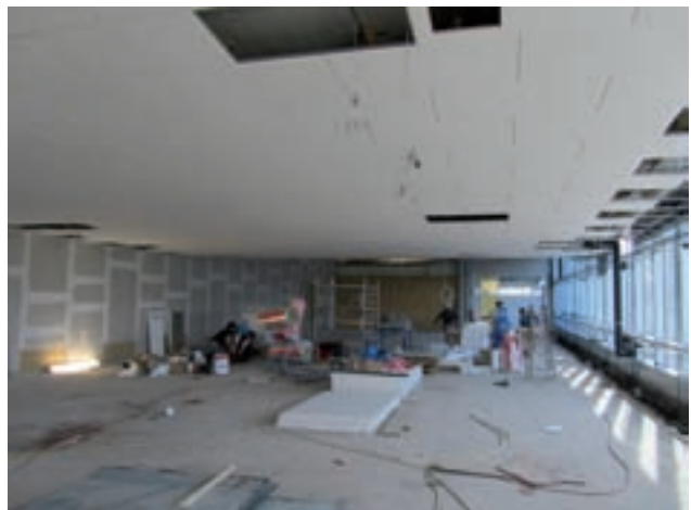
New metal cassette ceiling Image: PORR
