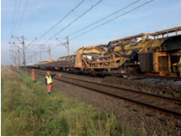
Sleeper replacement on Line 351 with the aid of the conversion vehicle Matisa P93 Image: PORR
