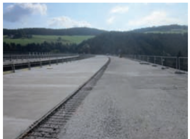
P46 top cover laid on one lane Image: PORR
