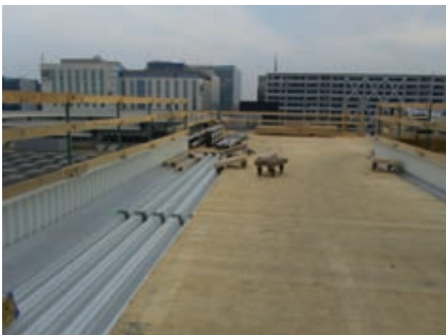
Ramp for construction site logistics Image: PORR
