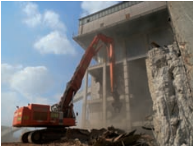
Hitachi 870 boiler dismantling Image: PORR
