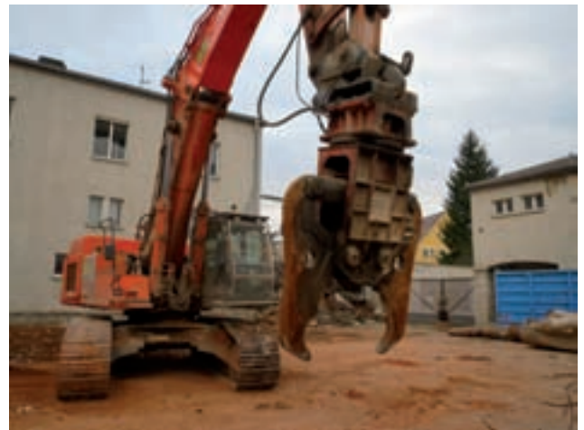
Hitachi 870 boiler dismantling Image: PORR
