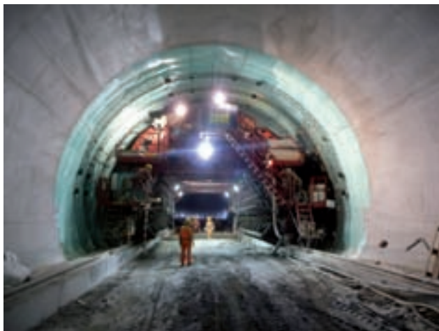
Arch formwork cart in bored tunnel construction Image: PORR
