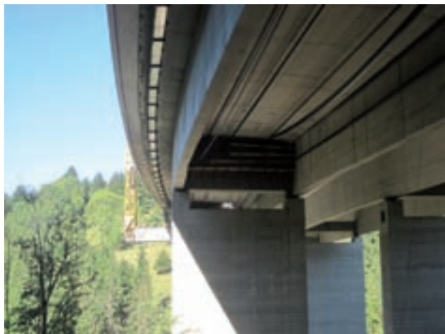
P44 External pre-stressing Image: PORR
