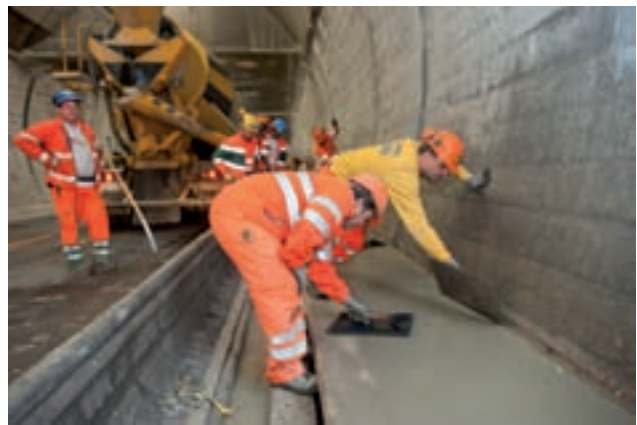
Hard shoulder concrete SBTU Image: PORR
