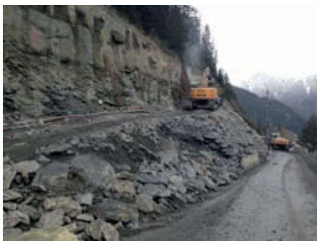
Anchoring work - Shotcrete work Image: PORR
