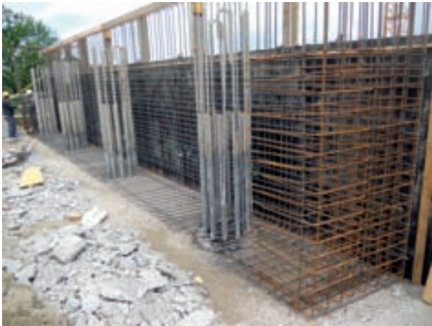
Abutment plate with connection to the drill pile Image: PORR
