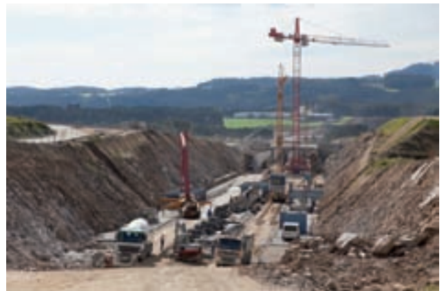
Pre-cutting of underground course UFT34 Image: PORR
