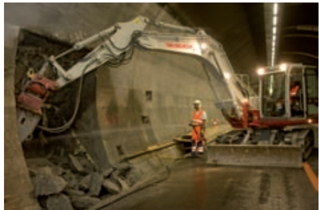
Construction of SOS niches Image: PORR
