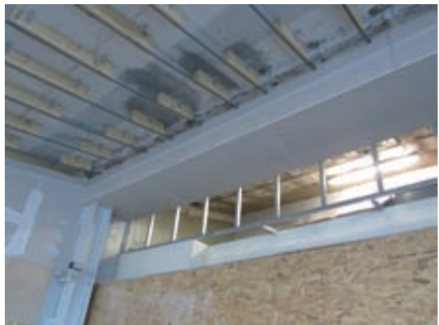
Steel cables under the new heat insulation layer Image: PORR
