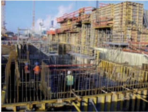
Condensate pit with turbine foundation and turbine platform Image: PORR
