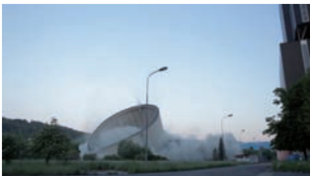
Cooling tower demolition Image: PORR
