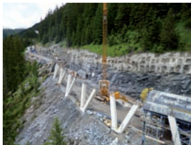
Production of the valley-side V-supports Image: PORR
