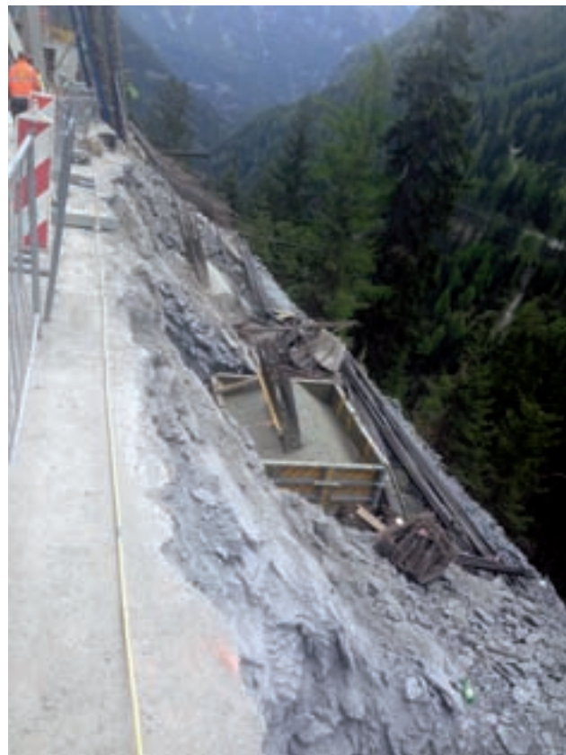
Production of the valley-side support foundations Image: PORR
