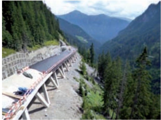
Gallery roof – Sealing work Image: PORR
