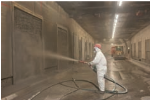
Spray concreting work Image: PORR
