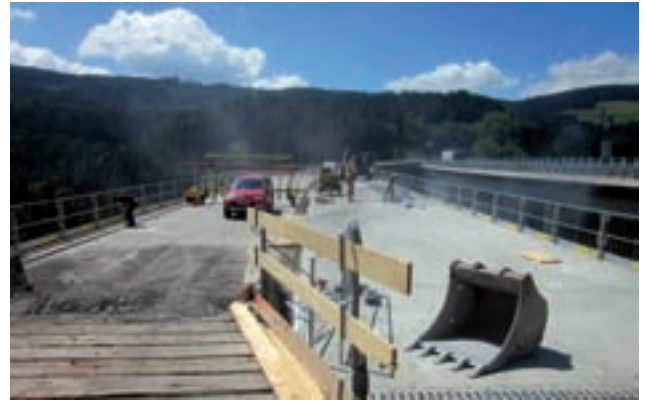
Preparation for concreting of top cover P46 Image: PORR
