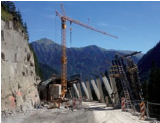
Start of block production by formwork cart Image: PORR
