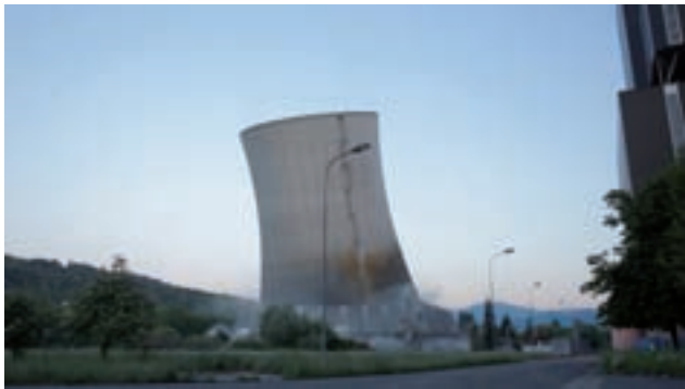
Cooling tower demolition Image: PORR
