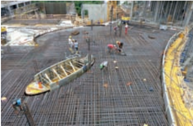
High reinforcement content BT 10 Image: PORR
