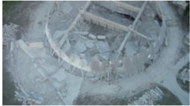
Cooling tower demolition Image: PORR
