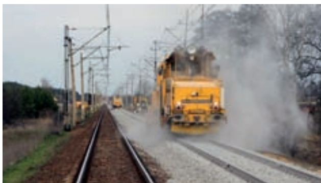
Ballast levelling machine of Austriarail in use on Line 273 Image: PORR
