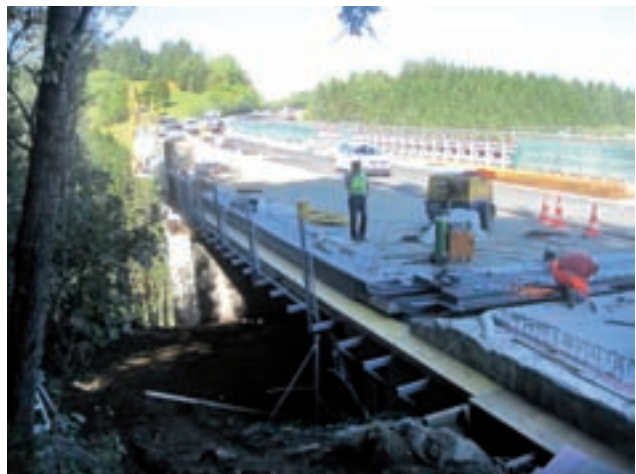
P44 abutment Graz, installation of carriageway transition construction Image: PORR
