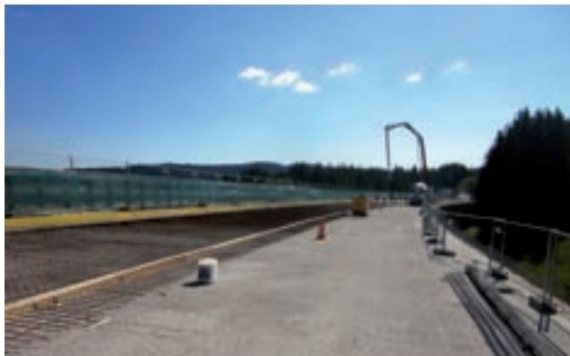
Preparation for concreting of top cover P45 Image: PORR
