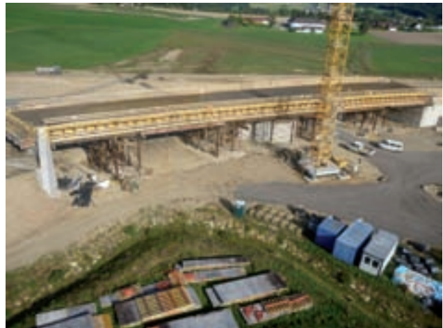
2-field integral construction Image: PORR
