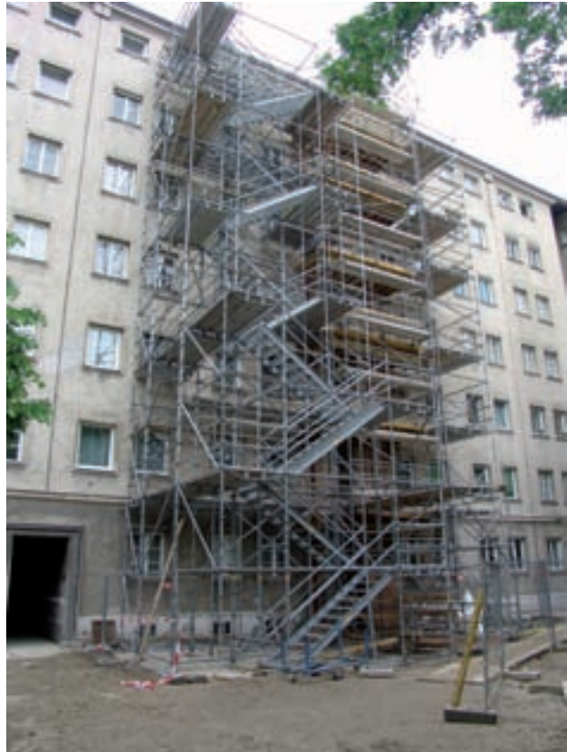
Temporary stairwell as escape stairwell tower Image: silberpfeil - architekten
