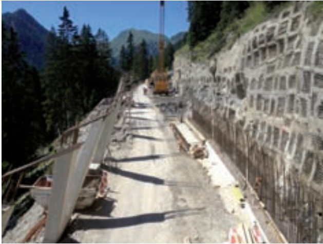
Production of the mountain-side strip foundations Image: PORR
