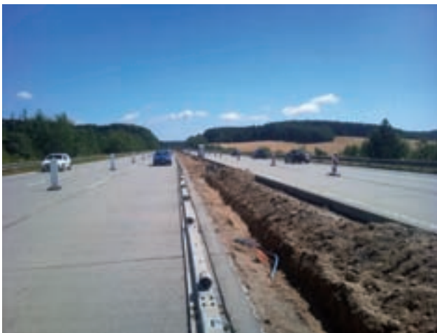
Renovation of the centre dividing strip, replacement of all lines and cabling and renovation of the central drainage pipe Image: PORR
