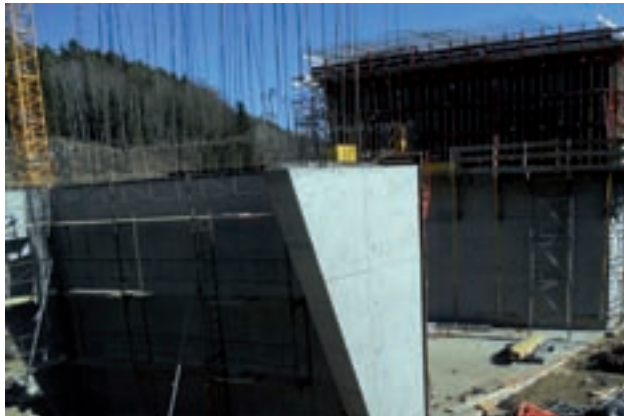
Formwork of the 12 m high abutment walls Image: PORR
