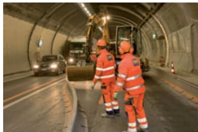
Miniguard relocation RPTU Image: PORR
