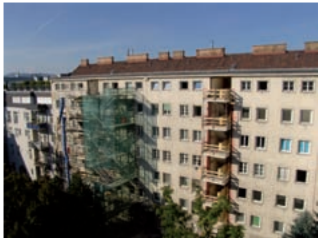
Completed stairwell tower after shell construction of the neighbouring stairwell Image: silberpfeil - architekten
