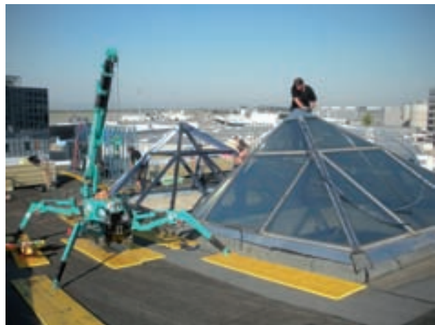
Demolition of the glass pyramids with the aid of a mini ramp crane Image: PORR
