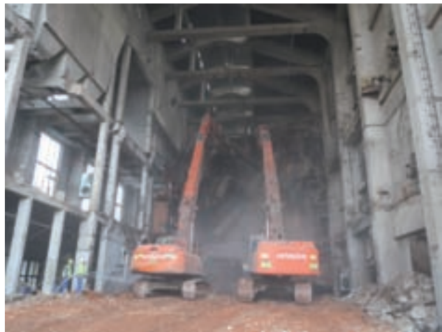
Picture 5: Boiler dismantling within building shell Image: PORR
