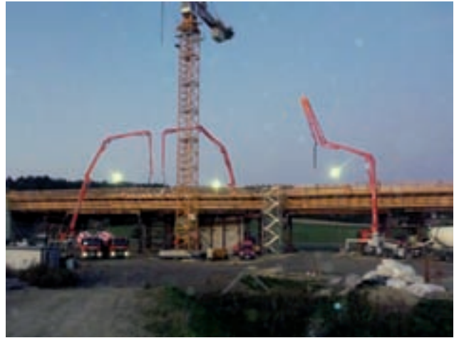
Concreting of supporting structure Image: PORR
