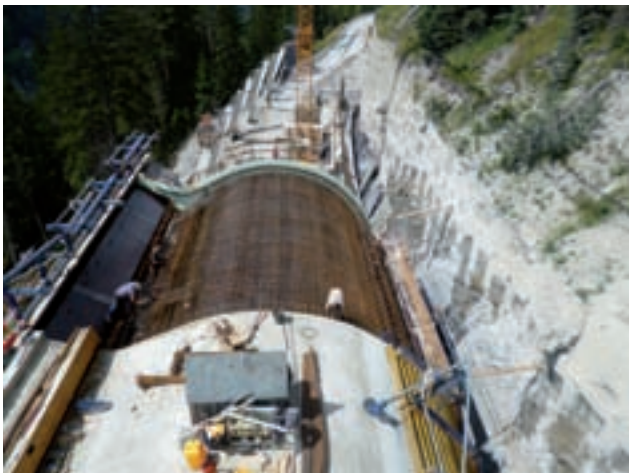
Reinforcement work – Arch supporting works Image: PORR
