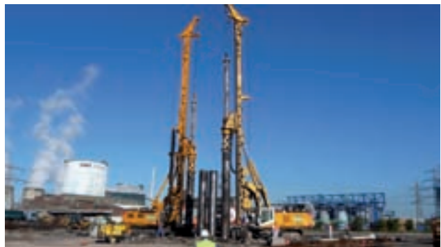
Production of the drill piles Image: PORR
