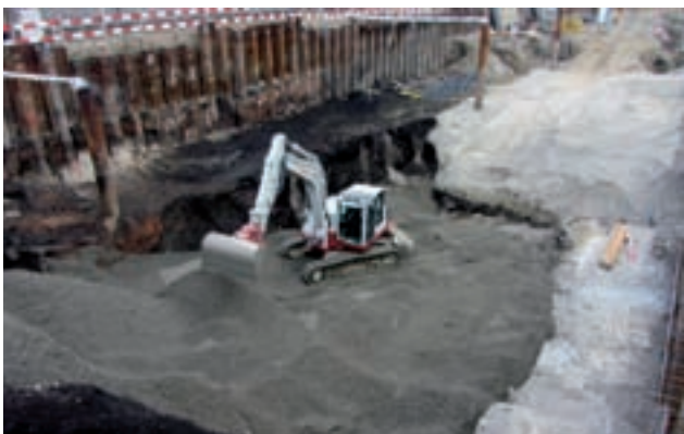
Soil replacement in the area of contaminated slag Image: PORR
