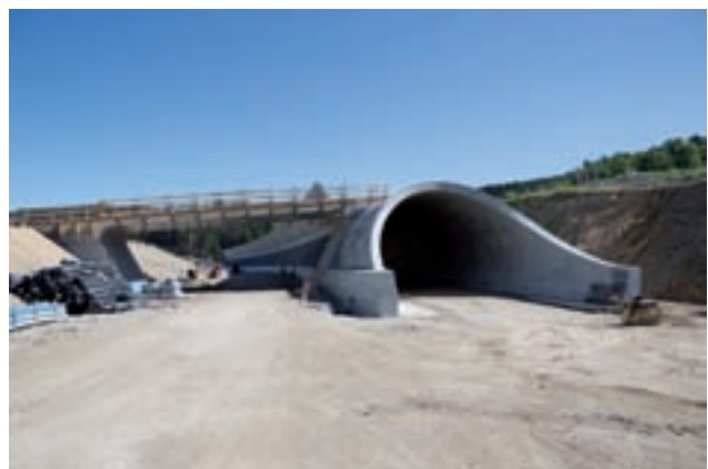
Concreting sections of the bored tunnel construction Image: PORR
