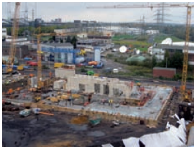
Turbine foundation and machinery building baseplate Image: PORR
