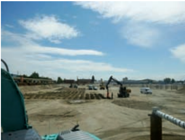
Sounding for unexploded munitions Image: PORR
