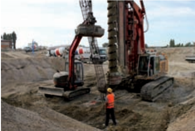
Drill pile works Image: PORR
