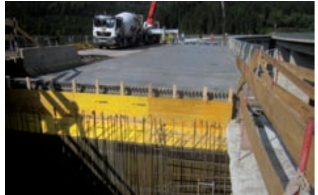
Concreting top cover of P46 Image: PORR
