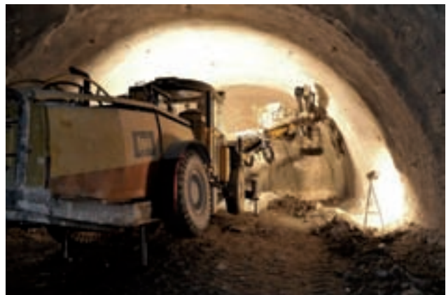
Drilling rig during drilling of the open face Image: PORR
