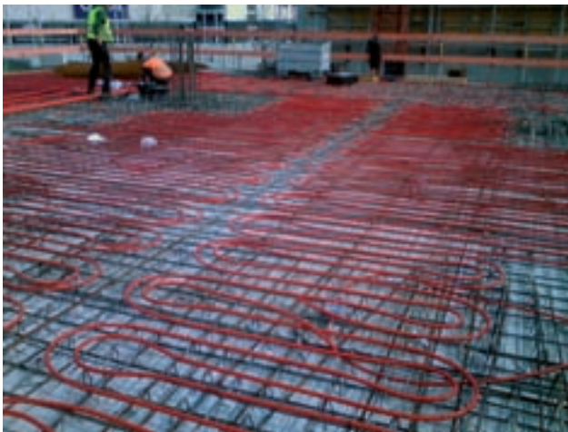
Concrete core temperature control Image: PORR
