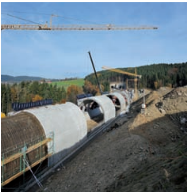
Brandstätter gallery concreting sections Image: PORR
