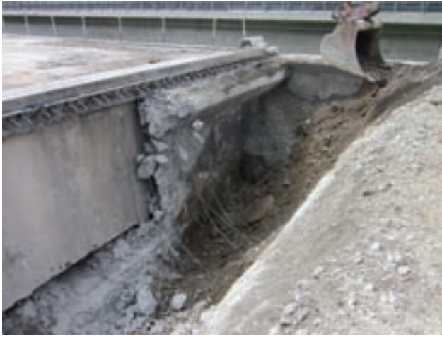
Demolition of bulkhead wall P46, abutment Graz Image: PORR
