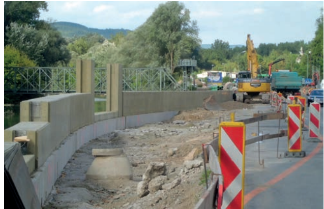
Completed flood protection wall Image: PORR
