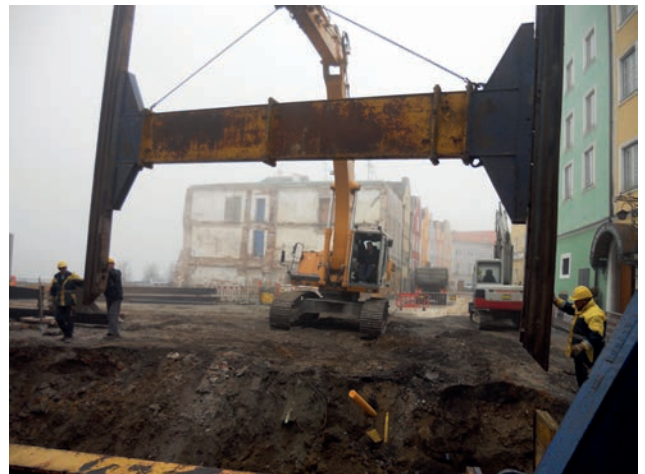
Installation of SBH earthwork supports at the Wienerstraße pump station Image: PORR
