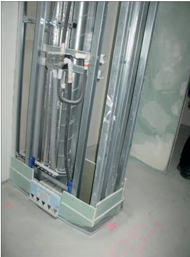
Supply pipes with floor-level inflow Image: PORR
