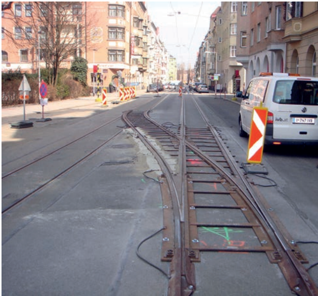
Climber points for diversion of tramway Image: PORR
