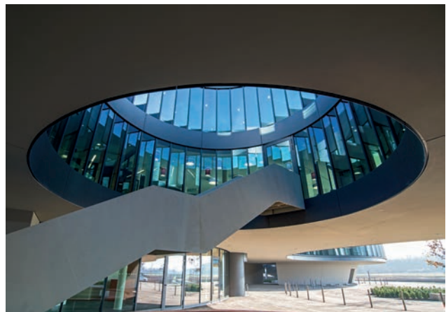
Timber stick-system curtain walling in inner courtyard Image: ALU-SOMMER
