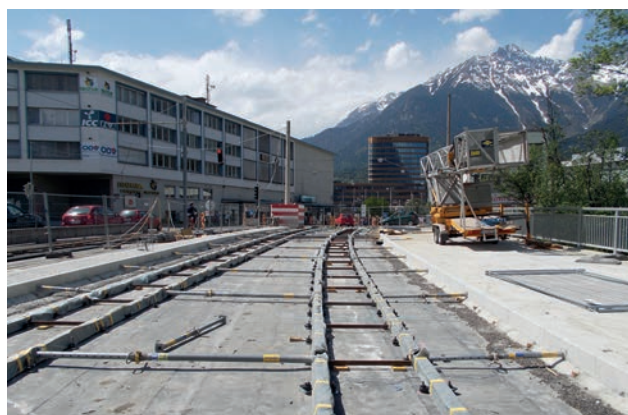
Attachment and protection of tracks on the bridge Image: PORR
