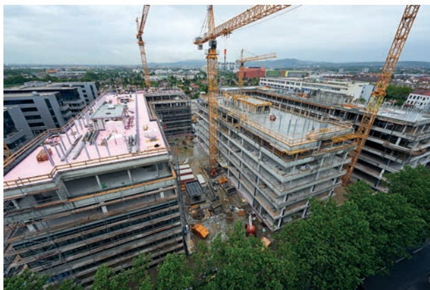
Steel support assembly and formation of inverted roof Image: Toni Rappersberger
