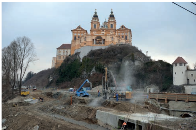
Melk Abbey – underground sealing works Image: PORR
