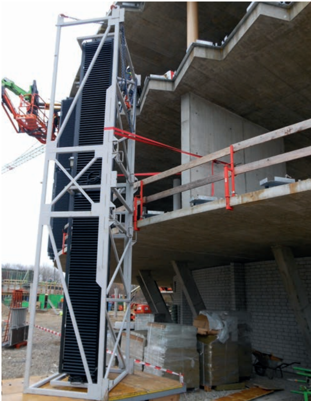
Installation of zigzag curtain walling (22.11.2012) Image: ALU-SOMMER
