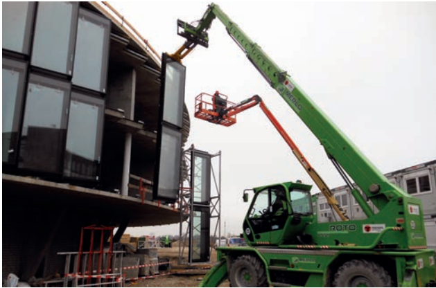
Installation of zigzag curtain walling (22.11.2012) Image: ALU-SOMMER
