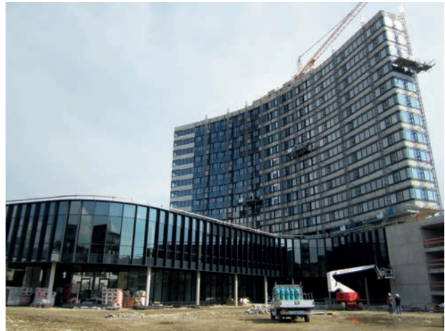
Curtain wall installation with mast climbers Image: PORR
