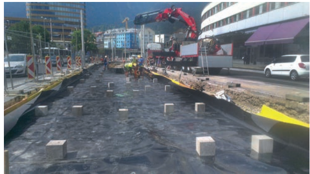
Installation of PE sheet and concrete blocks Image: PORR
