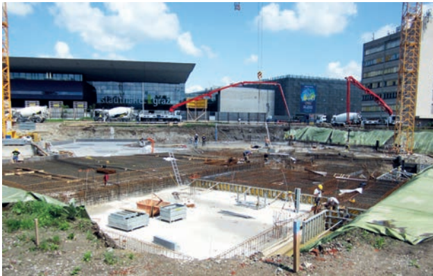
Basement pit with ground slab and, in background, bentonite tanking system Image: PORR
