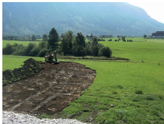
Fill placement for access road Image: PORR
