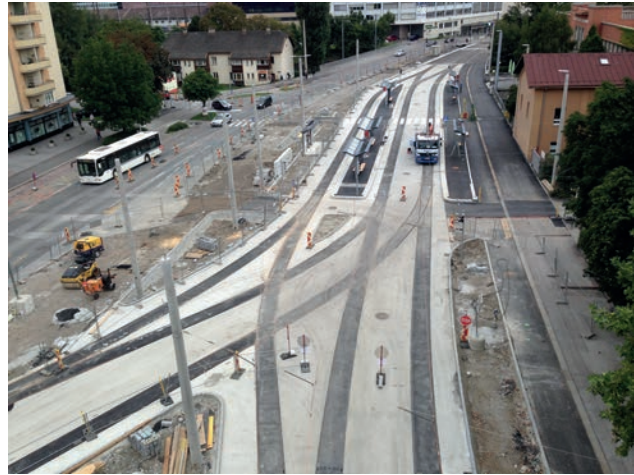
Semi-rigid surface in station area Image: PORR
