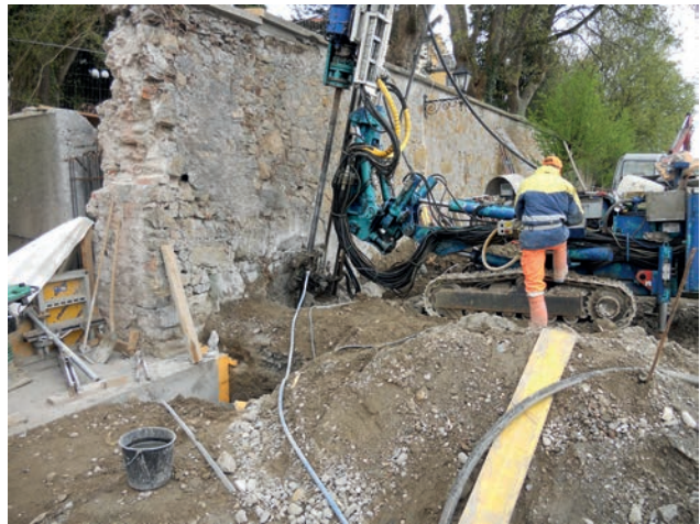
Injection grouted cut-off barrier below the town walls Image: PORR
