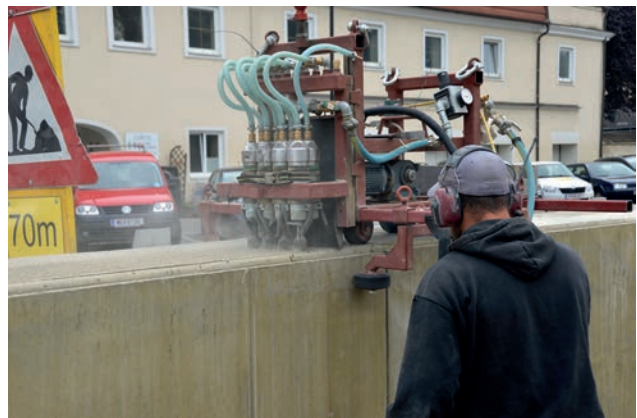
Bush hammering the top wall Image: PORR
