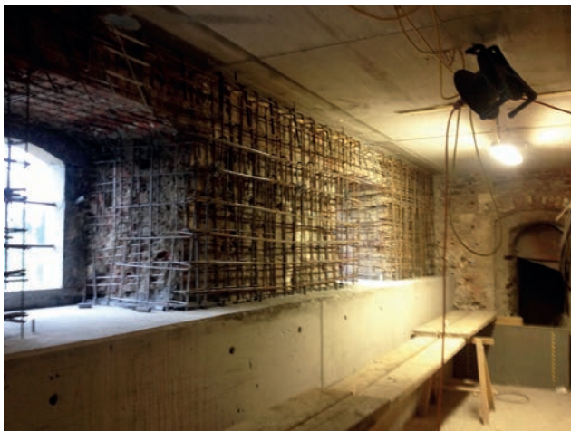
Concrete reinforcement on the building interior Image: PORR
