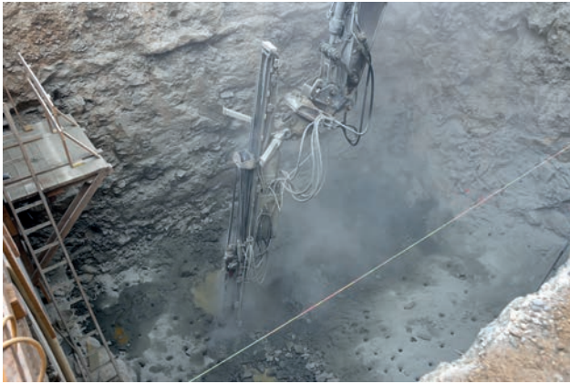
Pre-drilling for the installation of driving machines Image: PORR
