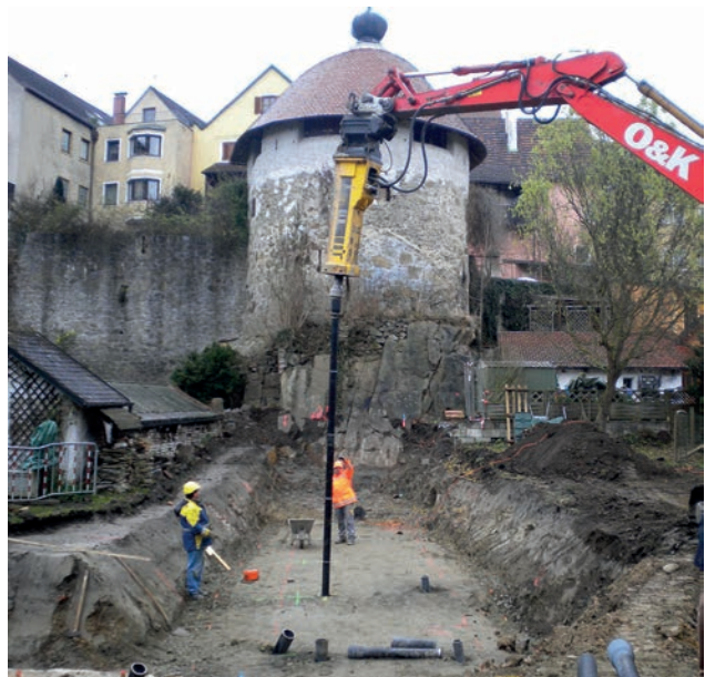
Ductile cast-iron piles as foundation for the floodwalls Image: PORR
