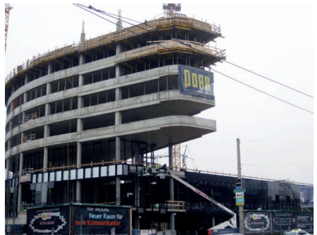
Building cantilever on Conrad-von-Hötzendorf-Straße front Image: PORR
