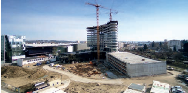
Concurrent construction of structural frame and curtain walling Image: http://smc.netzcam.net
