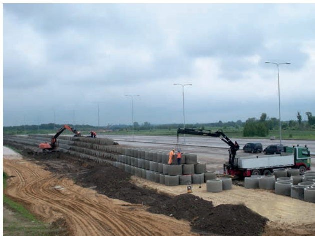
Construction of planted precast-concrete noise barriers Image: PORR
