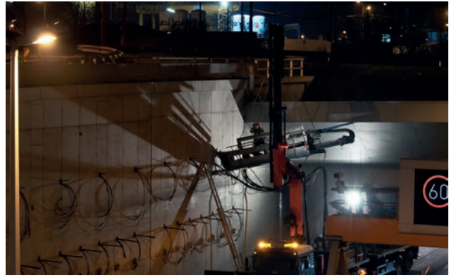
Fig. 5: Adapted drilling unit with drill carriage at a height of approx. 8.50 m Image: PORR
