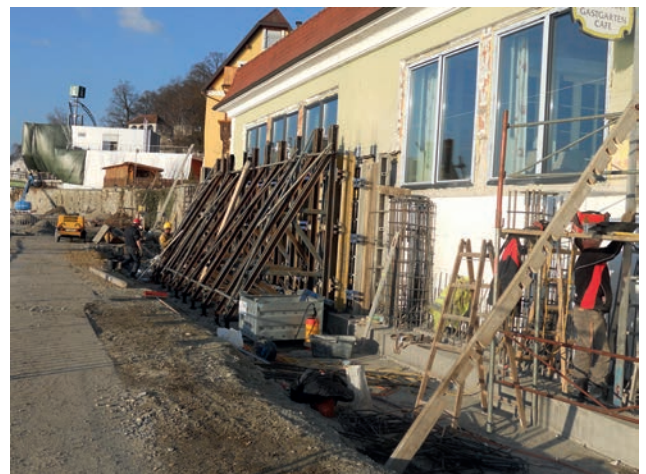
Formwork erection for foreland flood walls (Polder 2) Image: PORR
