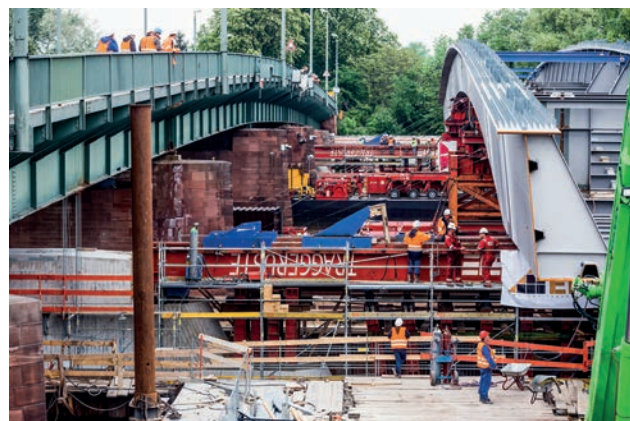
New bridge in Offenbach floated into temporary position Image: PORR
