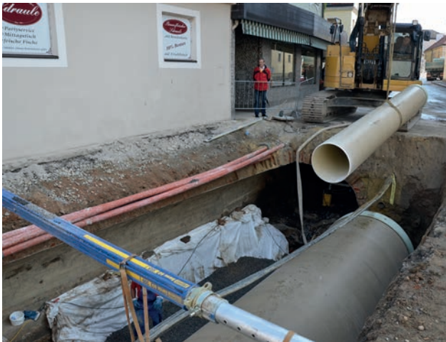
Demolition of the old Weierbach watercourse and construction of the new casing Image: PORR
