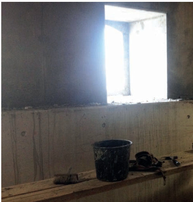
Fair-faced self-compacting concrete wall Image: PORR
