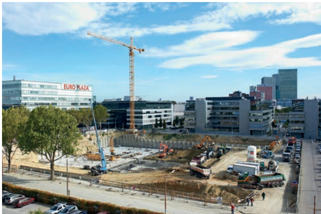
Initial base slab sections and earth excavation Image: Toni Rappersberger
