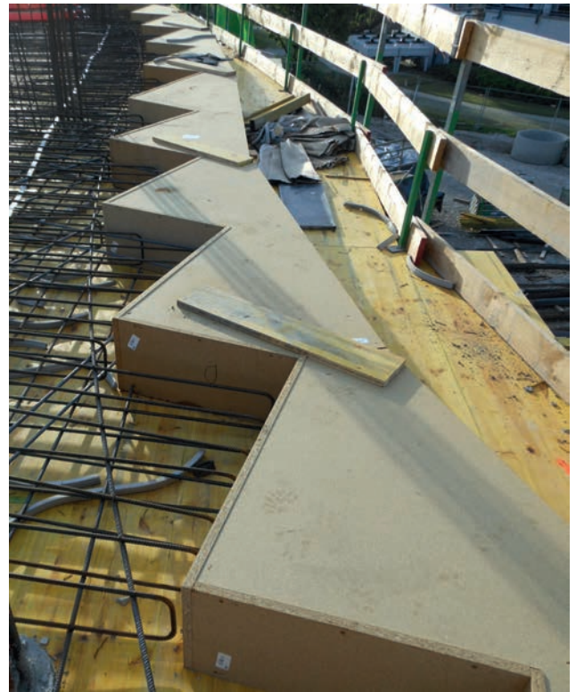
Outline of structural slab edge Image: ALU-SOMMER
