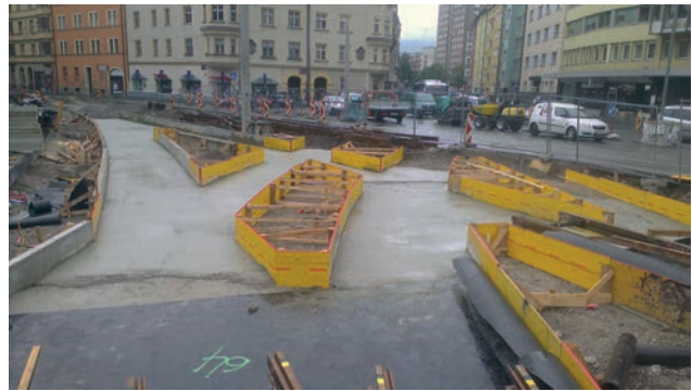
Preparation of subbase – track bed Image: PORR
