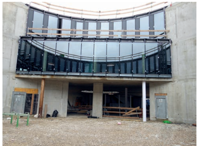
Stick-system curtain walling installed as preassembled units in inner courtyard (18.12.2012) Image: ALU-SOMMER
