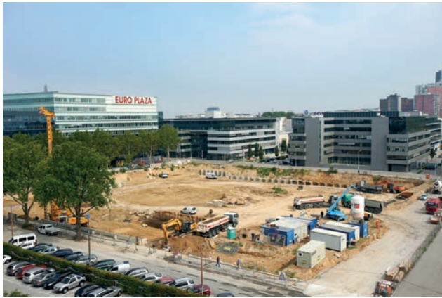
Initial excavation and pit support by means of cast-in-situ piles Image: Toni Rappersberger
