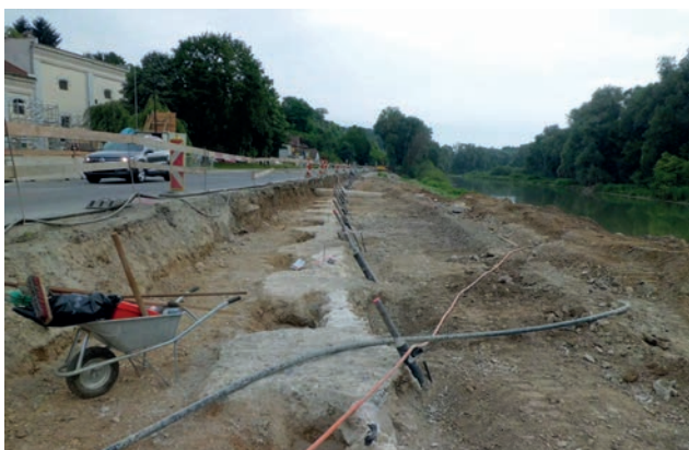
Exposed underground sealing with GEWI piles Image: PORR
