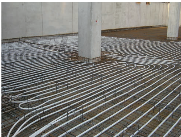
Concrete-core activation Image: PORR
