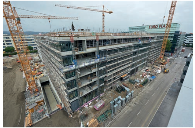
Facade assembly and mounting apertures by scaffolding platforms Image: Toni Rappersberger
