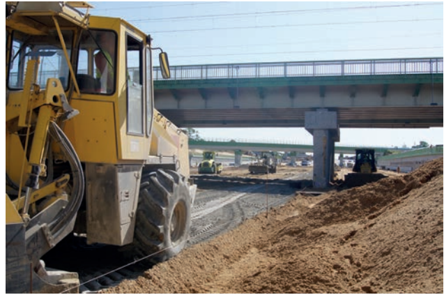
Cement stabilization of subgrade in cutting Image: PORR
