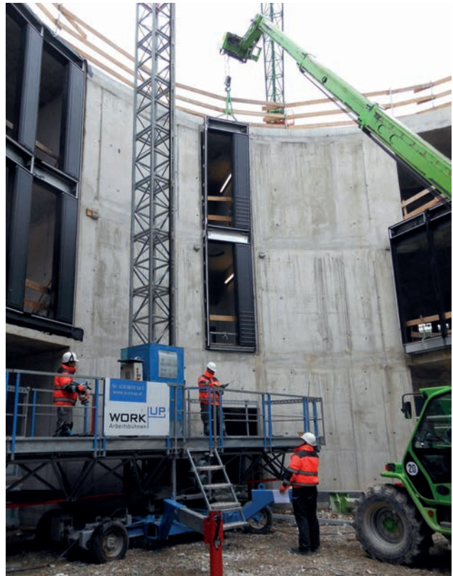
Installation of stick-system unit with telescopic handler (18.12.2012) Image: ALU-SOMMER
