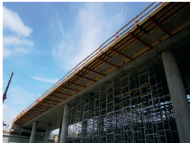
Formwork to bridge kerbs/perimeter strips for WD-20 Image: PORR
