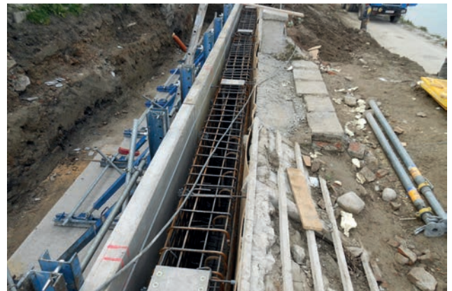
Anchor plates fixed in position prior to concreting Image: PORR
