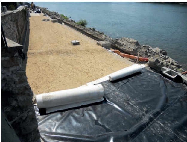
Sand bed to lay the waterproof membrane in Polder 2 Image: PORR
