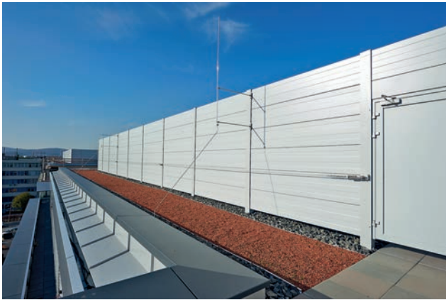
Crossover to mezzanine floor; angled sheet metal edging; planted roof and soundproof wall Image: Toni Rappersberger
