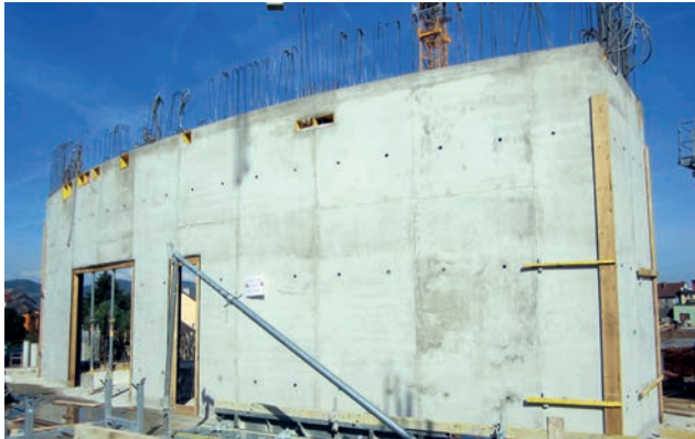
Section of fair-faced concrete wall Image: PORR
