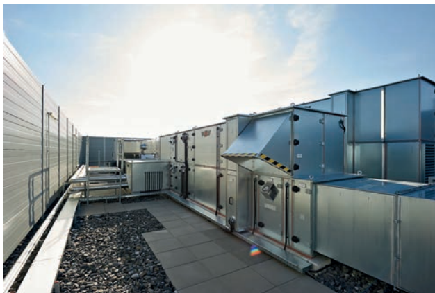
Ventilation facilities behind soundproof walls on roof BT J Image: Toni Rappersberger
