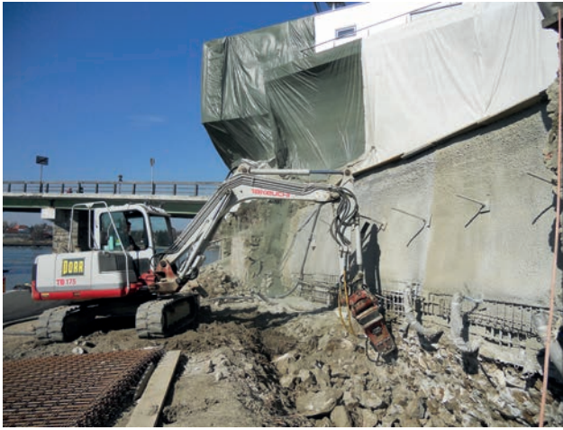
Removal of granite walls and simultaneous construction of shotcrete wall Image: PORR
