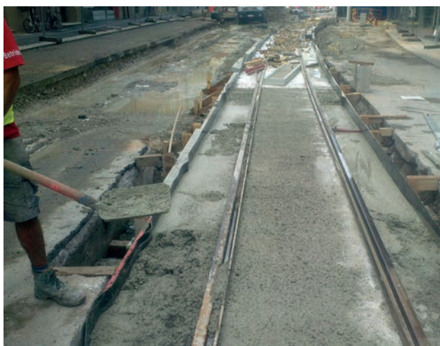
Concreting the track supporting layer Image: PORR
