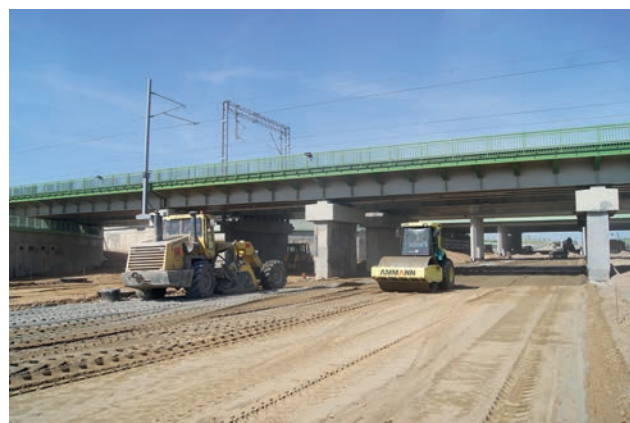
Ground improvement by cement stabilization in cutting – with railway overpass in background Image: PORR
