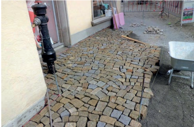
Natural stone paving Image: PORR
