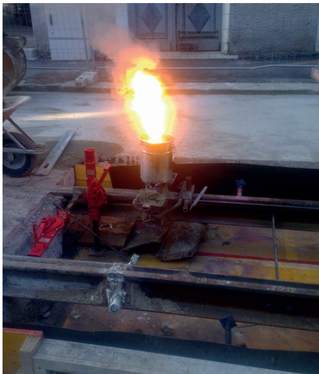
Welding the track joints Image: PORR
