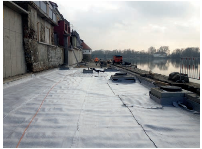
Membrane laid with drainage mat in Polder 1 Image: PORR
