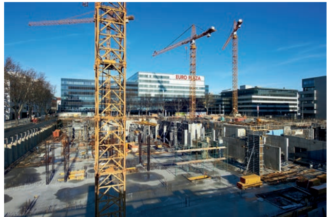
Concrete and reinforced concrete work on basement level 1 Image: Toni Rappersberger
