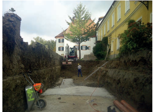
Excavation works for the floodwall behind the town walls Image: PORR
