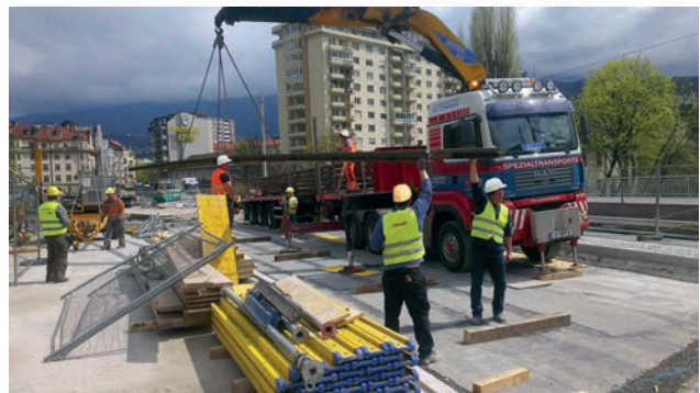
Hoisting the track panels Image: PORR
