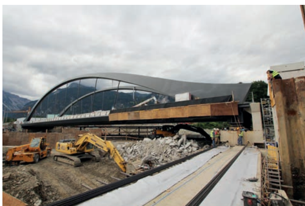
Transversal skidding Image: PORR AG
