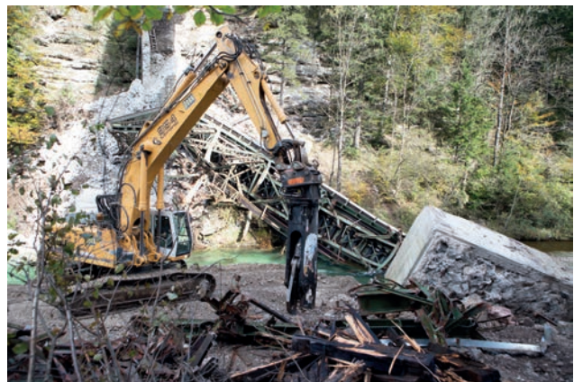
Removal of the blasted river Teichl bridge Image: Günther Gröger
