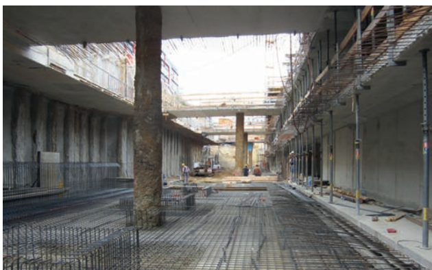
Cut-and-cover construction method Image: PORR AG
