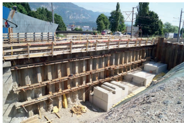
Abutment Kufstein – Pile grillage and foundations for wing wall Image: PORR AG
