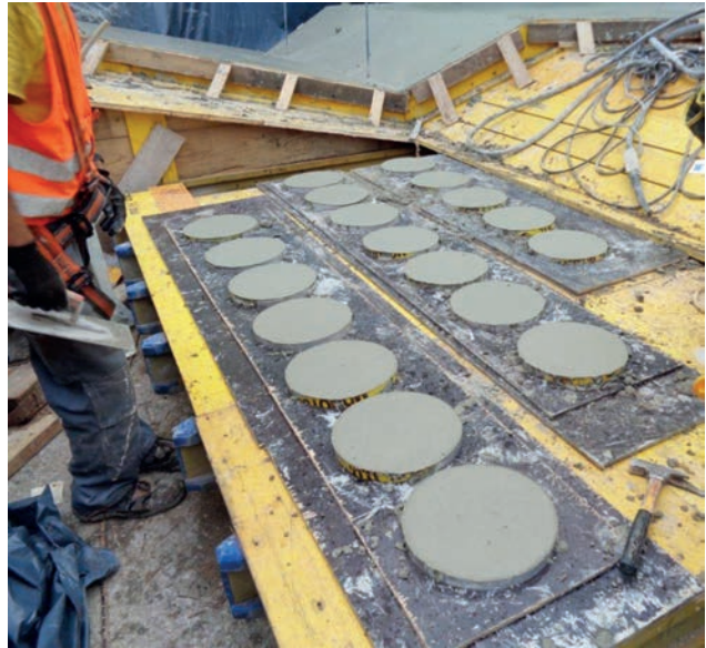
Production of deck panels for the purpose of closing the assembly openings Image: PORR AG
