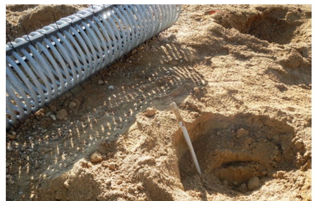
Borehole heat exchangers Image: PORR AG
