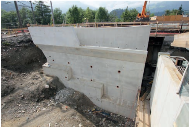
Abutment Kufstein – Completed wing wall Image: PORR AG
