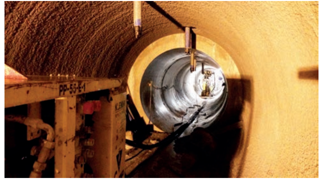
Seepage water tunnel with drainage well in the area of the tunnel top during horizontal drilling between tunnel and well Image: PORR AG
