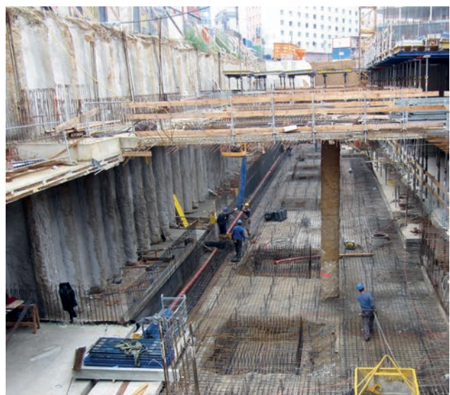
Cut-and-cover construction method Image: PORR AG
