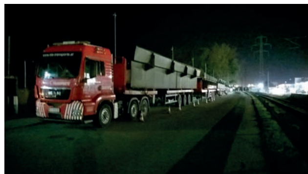
Existing superstructure supported on low-bed semi-trailers Image: PORR AG
