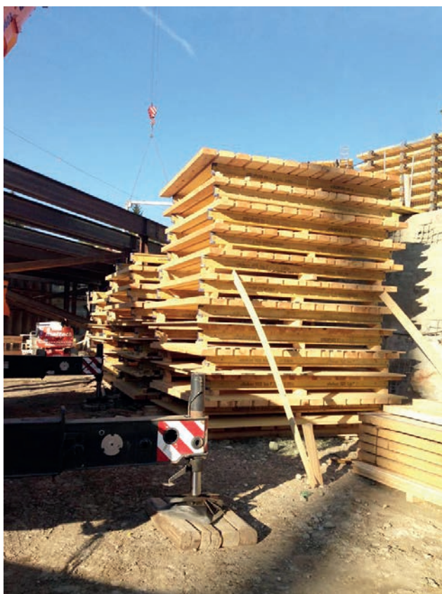
Storage of on-site constructed assembly bases for the safety scaffold Image: PORR AG
