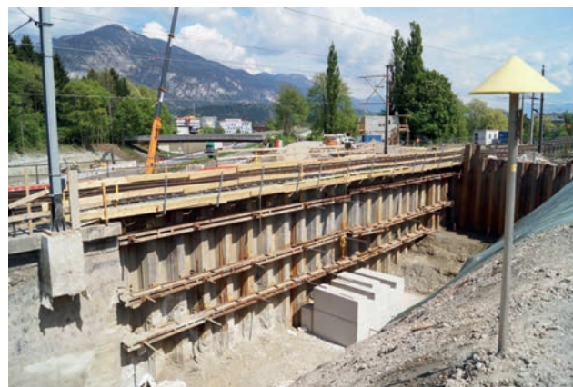
Abutment Wörgl – Cofferdam construction including operating path Image: PORR AG
