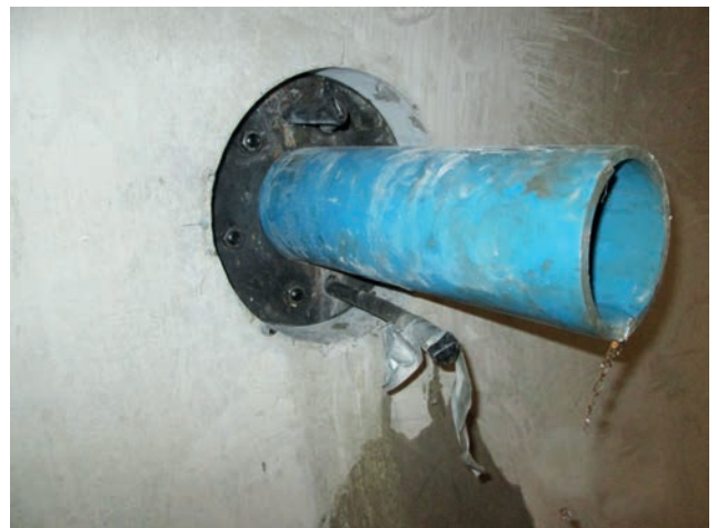
Completed drainage line with sealing using a packer system for the collection of seepage water from the drainage well Image: PORR AG
