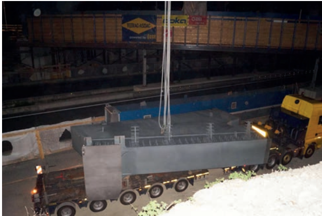
Installation of 80 t arch base Image: PORR AG
