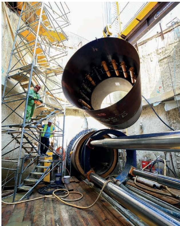
Installation of the interjack station Image: APA/Wien Kanal
