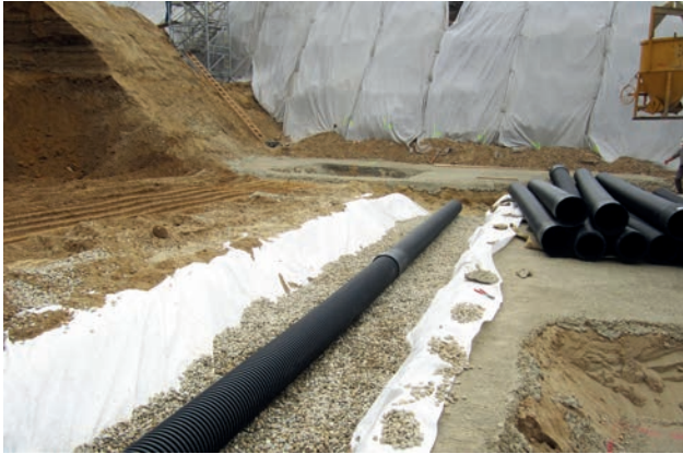
Seepage underneath the bottom slab Image: PORR AG
