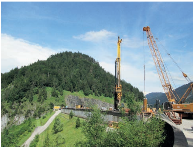
Building site with BG 36 drilling rig for drilling work and LH853 cable excavator for well removal and dismantling of piping d=880mm Image: PORR AG
