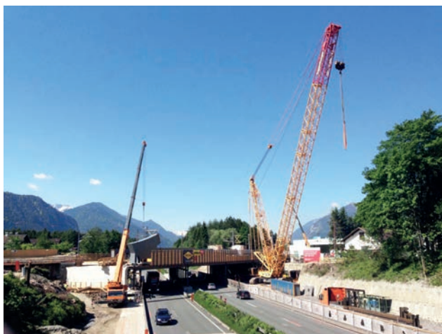
Assembly of steel frame Image: PORR AG
