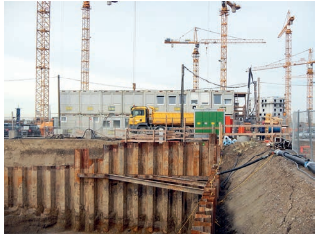
Temporary construction pit system by means of sheet piling Image: PORR AG
