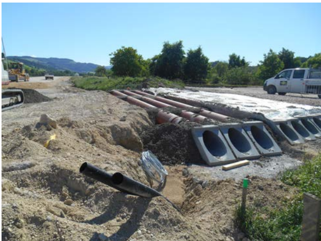
Construction of pipe culverts for flood water drainage Image: PORR AG
