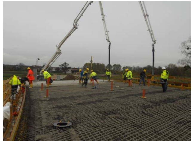
Bridge over the Kleine Erlauf river, concreting of the superstructure Image: PORR AG
