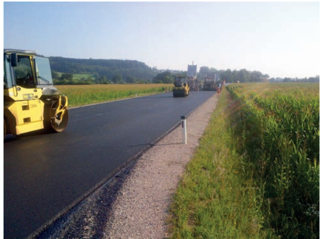
Application of the asphalt cover layer with two tracked pavers Image: PORR AG
