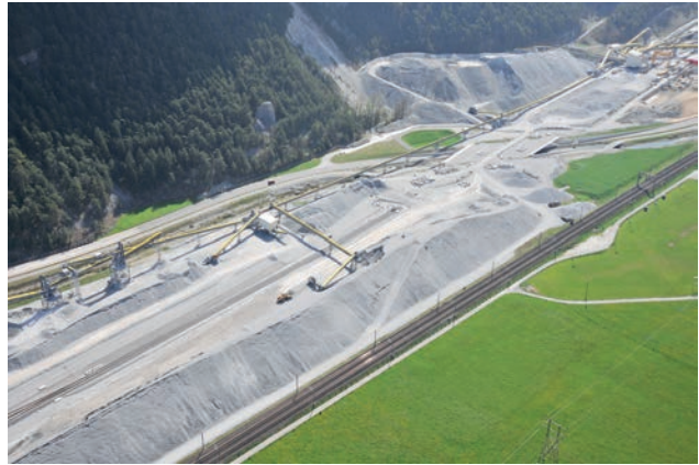
Conveying devices and temporary storage of the excavated material for ballasting
