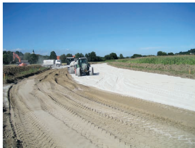
Ground stabilisation in the area of embankment road-contact surfaces Image: PORR AG
