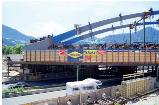
False work for superstructure form work Image: PORR AG
