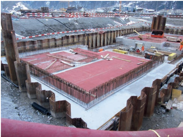
Construction pit and bottom slab of northern pipe basement Image: PORR AG
