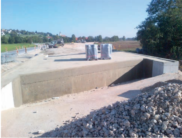
Mühlbach river bridge – sealing work Image: PORR AG
