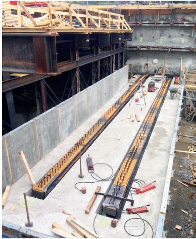
Installation of skid rails in their foundations Image: PORR AG
