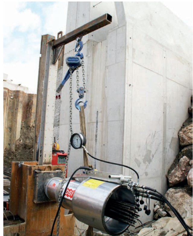
5 MN stressing jack for transversal skidding Image: PORR AG
