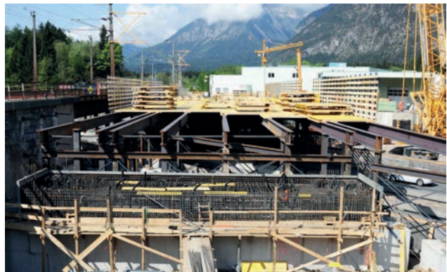
Reinforced and formed bearing blocks with concreting and ventilation openings Image: PORR AG
