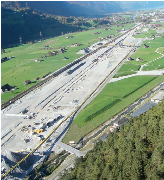
Railway bed in northern direction - construction condition of the northern segment after half a year of construction; on the left one can see the core line of the Gotthard railway, on the right: the conveying system's yellow belts
