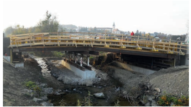
Bridge over the Kleine Erlauf river, completion of form work Image: PORR AG
