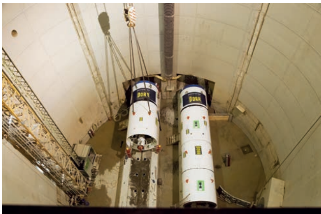
Insertion of tunnel boring machine using 800 t crane Image: PORR AG
