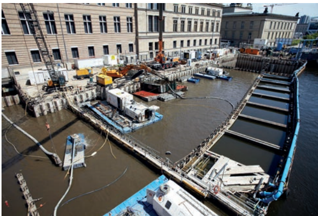
View into the manufactured and partly pumped out trough type pits Image: PORR AG
