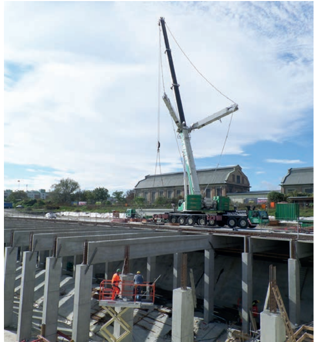
Shifting of the precast beams from the ceiling by means of a 400t crane Image: PORR AG
