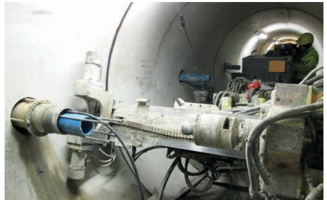
Execution of horizontal drilling using basement drilling rig in the tunnel with a diameter of 2.4 m. Installation of the drainage pipe inside the temporary piping (d=178 mm) Image: PORR AG
