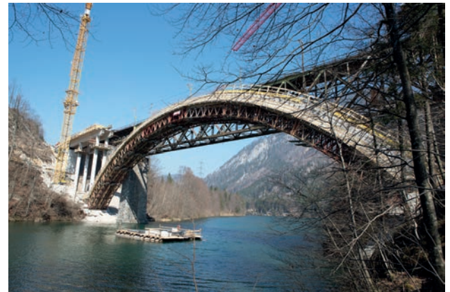
False work arch support structure Image: PORR AG
