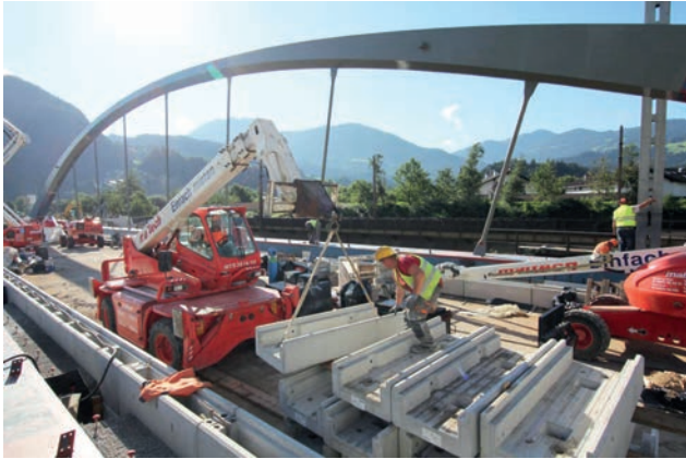
Installation of pre-fabricated cable troughs on the superstructure Image: PORR AG
