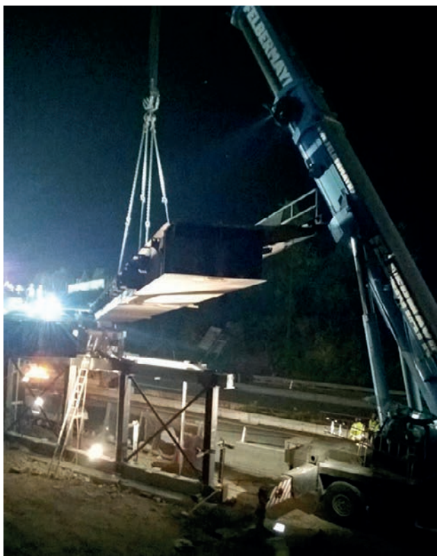
Excavation existing superstructure by means of a 500 t mobile crane Image: PORR AG
