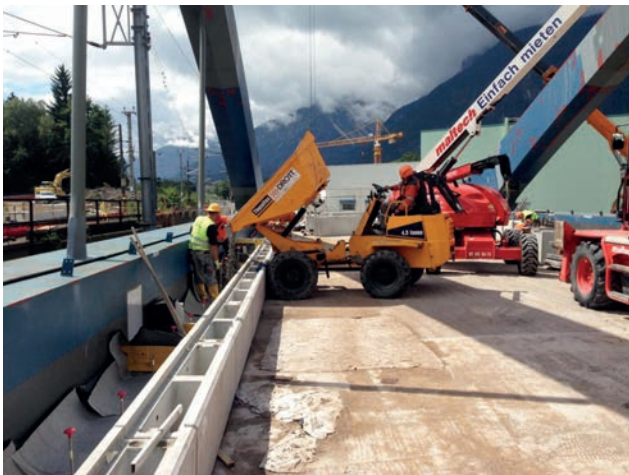
Placement of single-grain concrete below the pre-fabricated cable troughs Image: PORR AG
