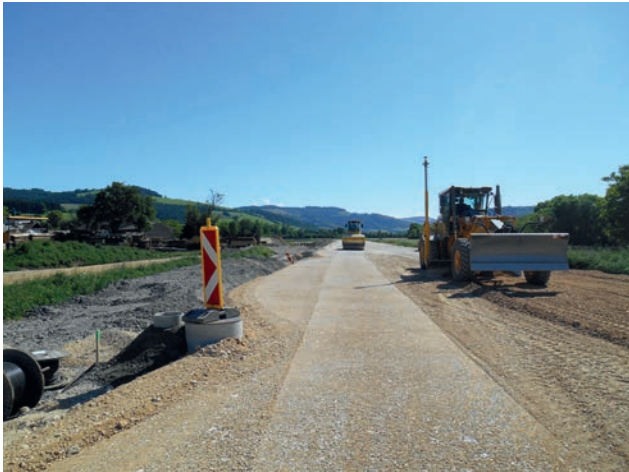
Installation of unbound supporting layers with theodolite-controlled grader Image: PORR AG
