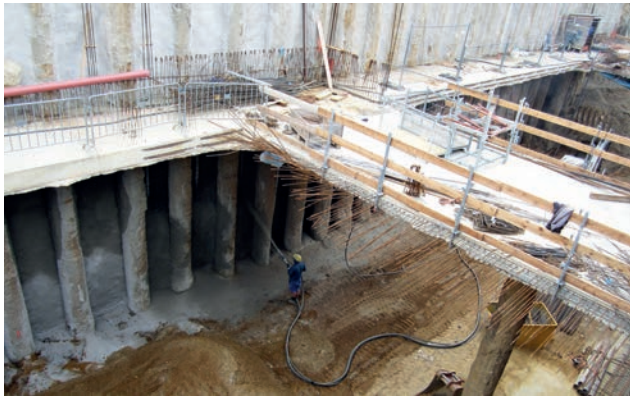
Cut-and-cover construction method Image: PORR AG
