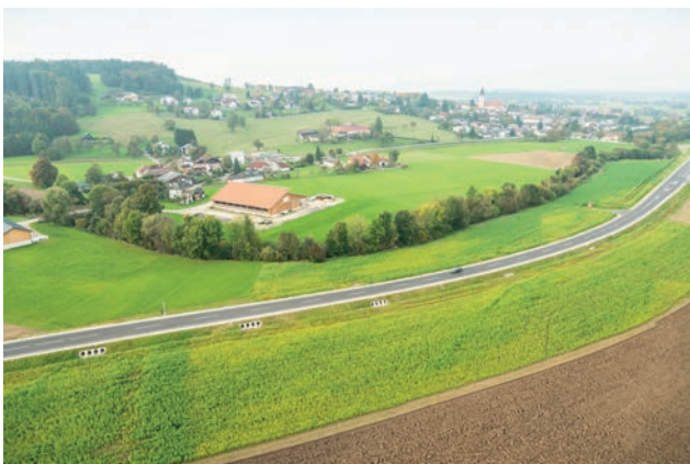
Pipe culverts through bypass road for the purpose of flood water drainage Image: Markus Hahslinger
