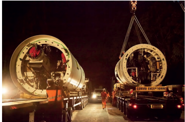
Insertion of tunnel boring machine / heavy transport Image: PORR AG
