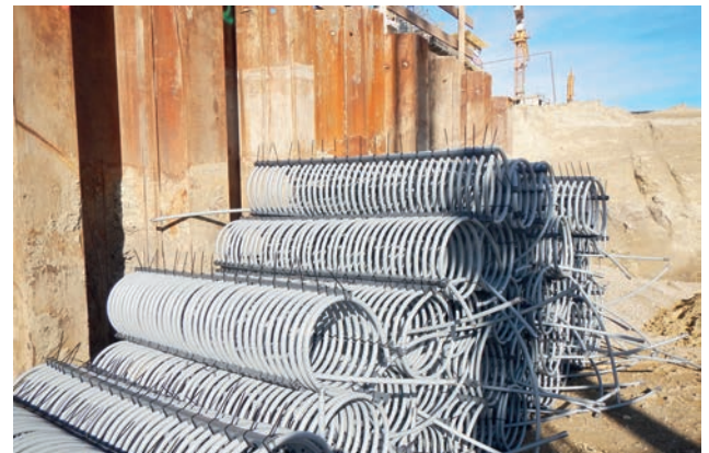
Borehole heat exchangers Image: PORR AG
