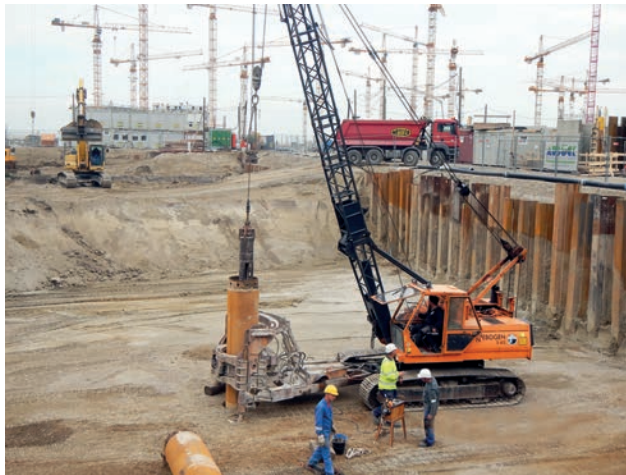
Well installation for lowering the ground water table Image: PORR AG
