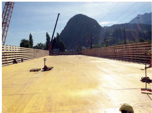
Safety scaffold above A12 motorway Image: PORR AG
