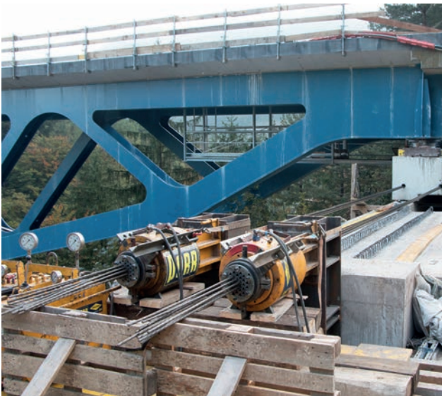
Lateral shifting of the new river Teichl bridge Image: Günther Gröger
