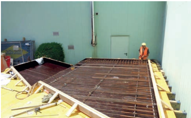
Installation of pre-fabricated chamber walls Image: PORR AG
