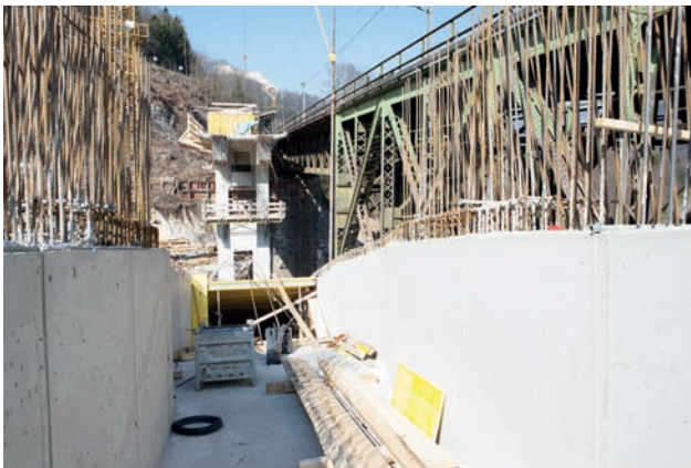
Manufacturing of arch box girder Image: Günther Gröger
