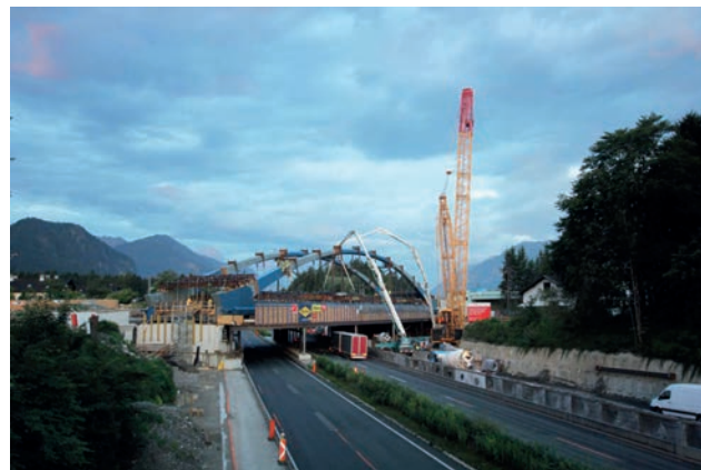
Concreting of 1,100 m 3 track supporting layer Image: PORR AG
