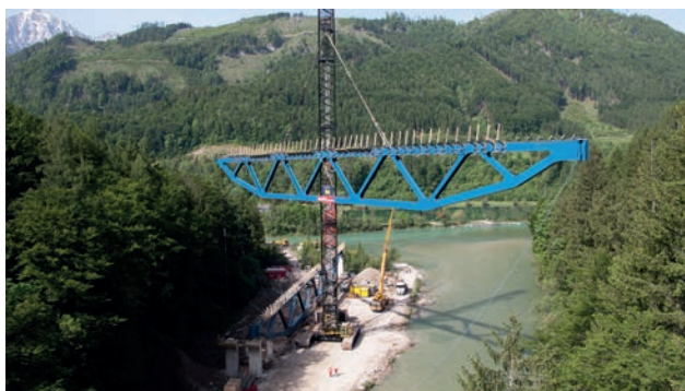
Shifting of steel form work girders and pre-assembly site Image: Günther Gröger
