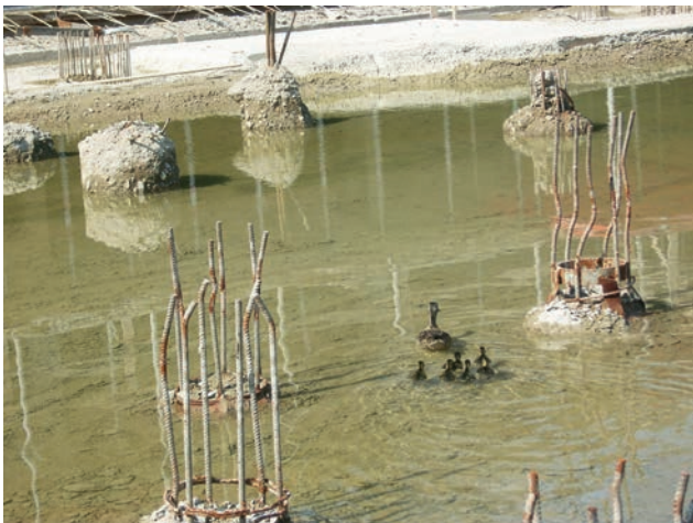
Pile caps in the underground car park construction pit during the flood Image: PORR AG
