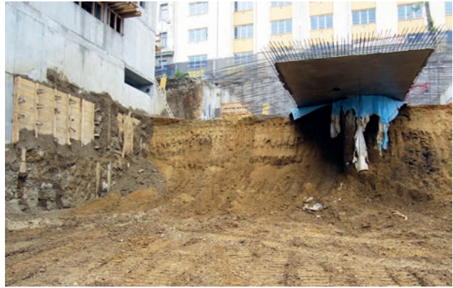
Construction pit reinforcement by means of concrete grates and protruding platforms Image: PORR AG
