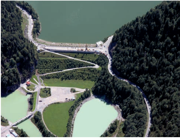
Aerial shot in direction of Sylvenstein reservoir: in the foreground, one can see the outlets for the regulation of the water level Image: PORR AG
