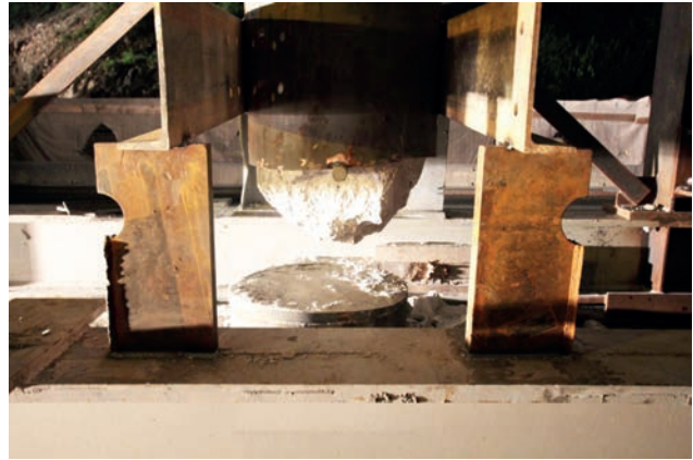
Cut-off rocking pier after 20 cm of transversal skidding Image: PORR AG
