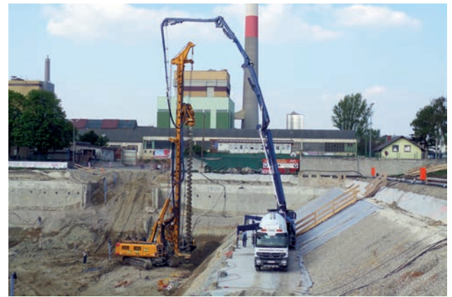
Manufacturing of CFA piles Image: PORR AG
