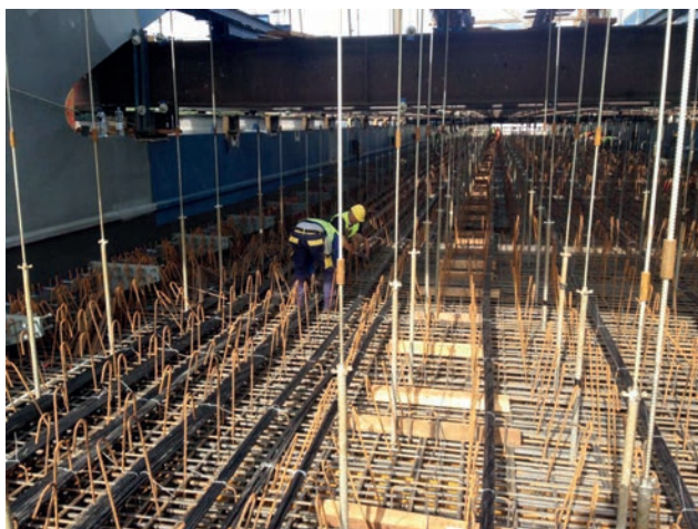
Feeding and fastening of tension members Image: PORR AG
