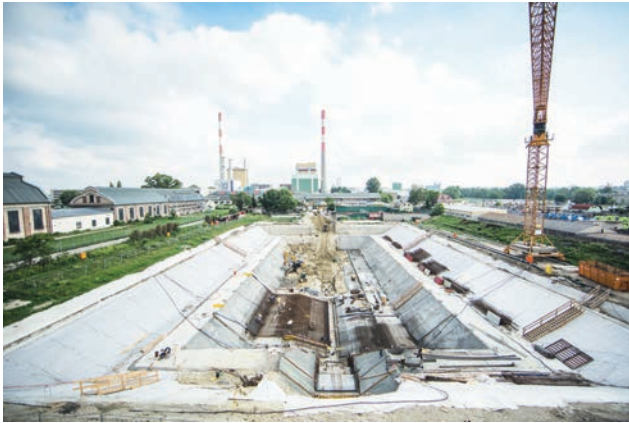
Completed construction pit including clear layer Image: APA/Wien Kanal
