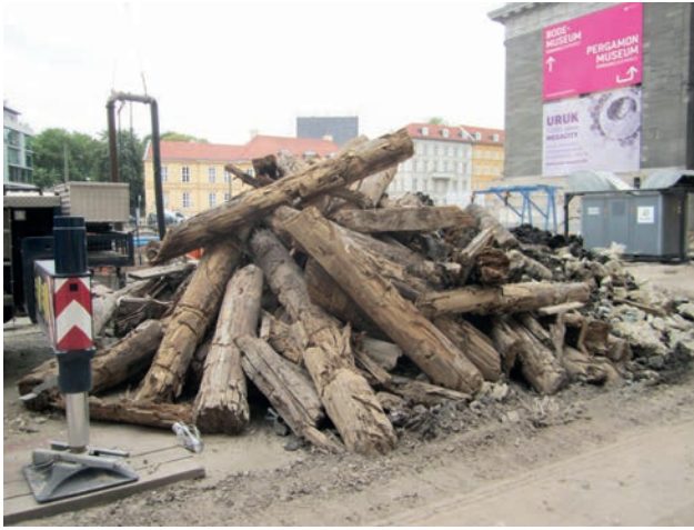
Recovered wood piles from the former foundations on the building site Image: PORR AG
