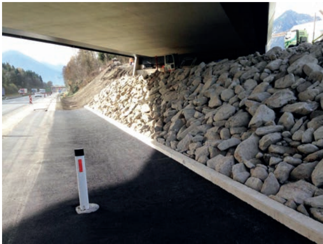
Installation of dump stone riprap below the new bridge Image: PORR AG
