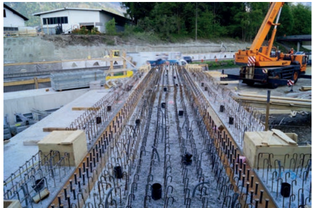
Laid counterform work (deck panels) for the construction of the bearing blocks Image: PORR AG
