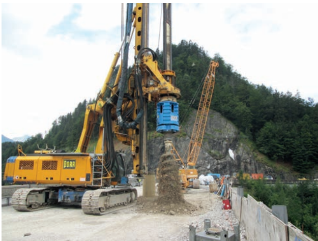
BG36 drilling rig with automated rotary table and drilling auger during drilling work on the dam body Image: PORR AG
