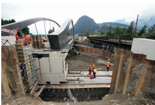
Transversal skidding Image: PORR AG
