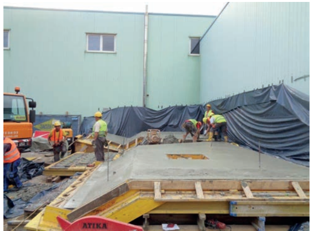
Concreting of pre-fabricated chamber walls Image: PORR AG
