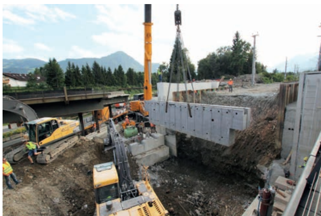
Installation of pre-cast shoes for subsequent skidding Image: PORR AG
