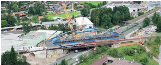
Completed arch superstructure and false work for superstructure form work Image: PORR AG
