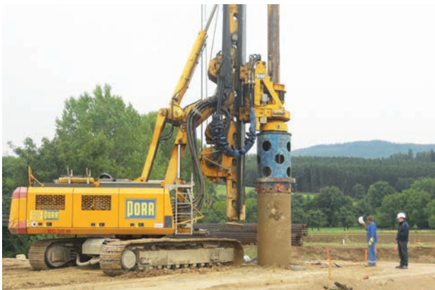
Bridge over the Kleine Erlauf river, construction of deep foundations using bored piles Image: PORR AG
