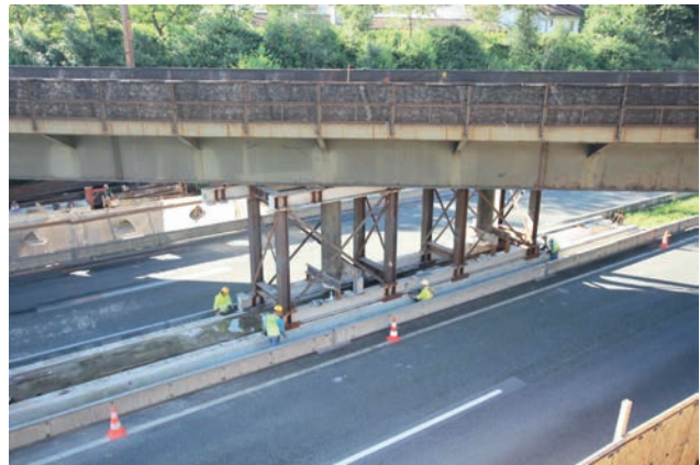
Transversal skidding of the existing structure Image: PORR AG
