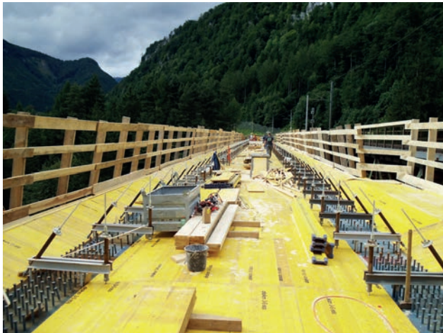
Composite track slab manufacture Image: PORR AG
