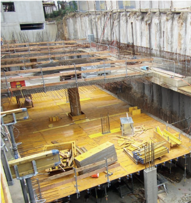
Cut-and-cover construction method Image: PORR AG
