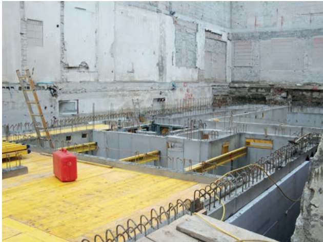
Newly constructed basement in the existing building Image: PORR AG
