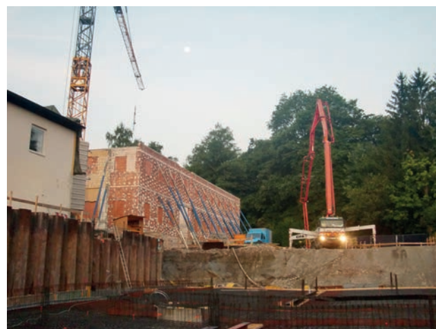
View of supported existing walls Image: PORR AG
