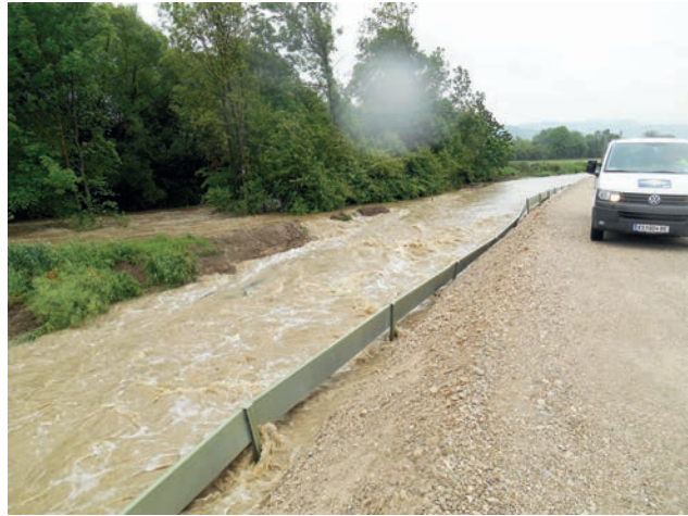
Flooding on the commercial roads, underwashing of the amphibian protections Image: PORR AG
