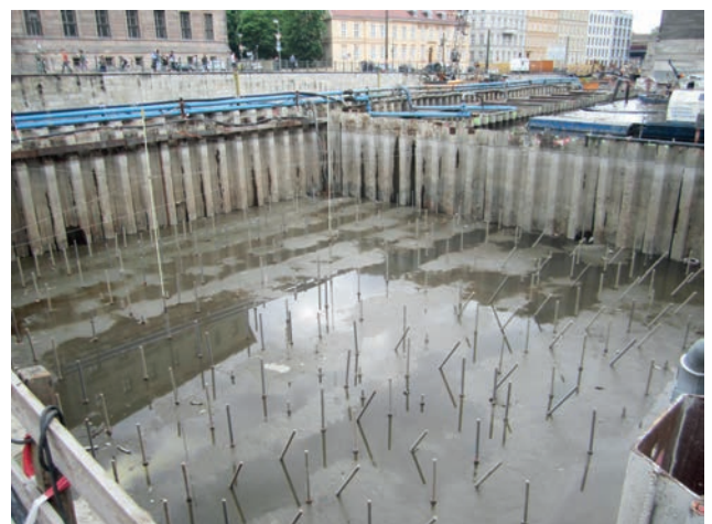
View into a pumped out trough type construction pit with underwater concrete base and micropile back-anchoring Image: PORR AG
