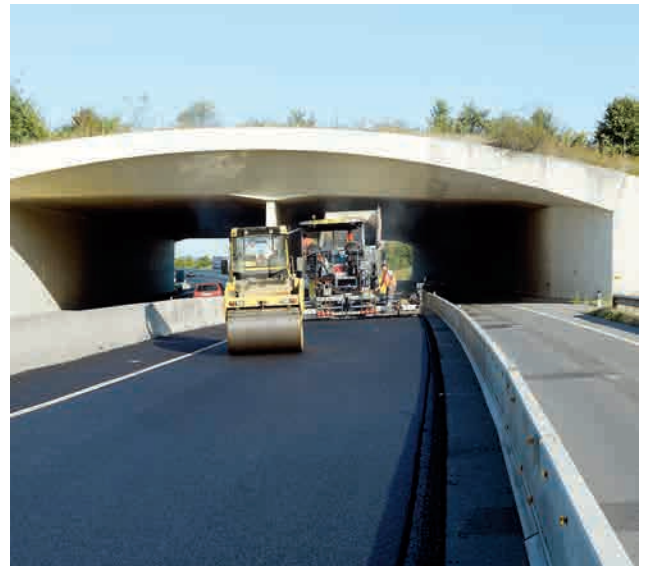
Laying asphalt Image: PORR AG
