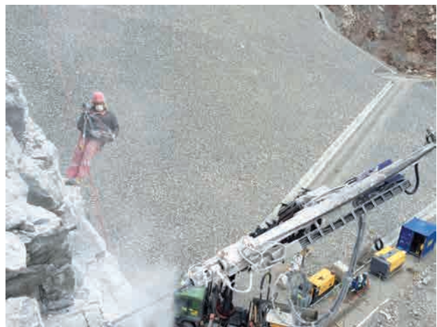
Creation of drill holes for the rock nails by means of drilling lorry Image: PORR AG
