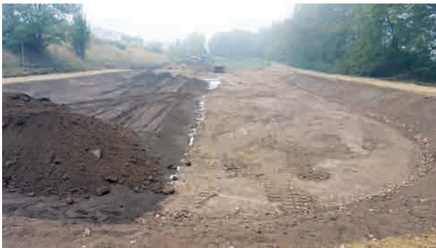
Earthworks on soakaway pits Image: PORR AG
