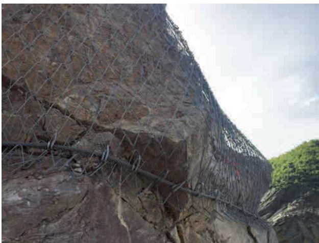
Completed high performance net Image: PORR AG
