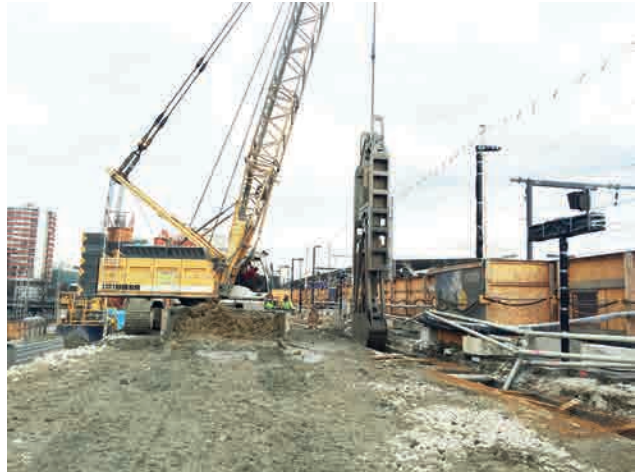
Perron high-rise building at Salzburg Main Station: Difficult diaphragm wall construction in direct vicinity of the platform Image: PORR AG
