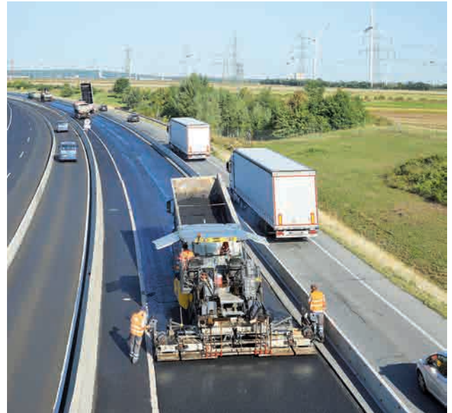
Laying asphalt Image: PORR AG
