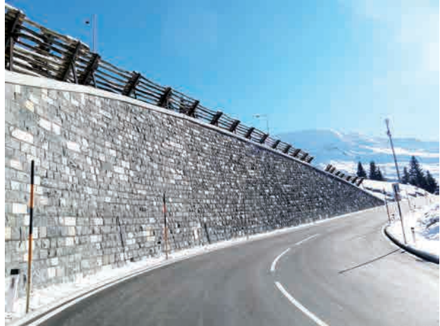
Support wall no. 1 with natural stone cladding, October 2015 Image: PORR AG
