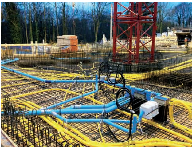
Underground car park ceiling installations Image: PORR AG
