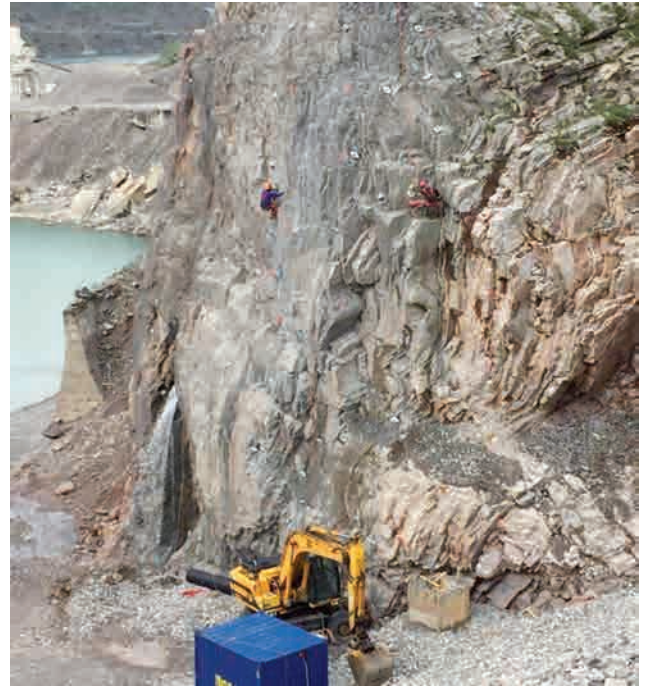
Completion of rock stabilisation by means of wire nets – working while suspended from ropes Image: PORR AG
