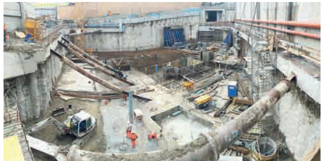
Walking a technical borderline – Orbi Tower construction pit in the triangle between underground, flight control and motorway. Piles, jet grouting, anchors, steel reinforcements, dewatering system, project planning: everything from a single source. Image: PORR AG
