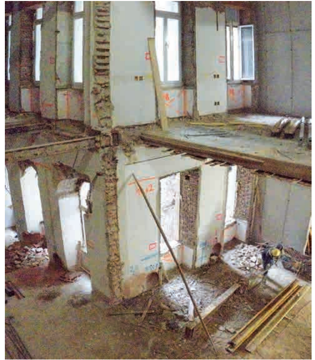
Timbered ceiling removal Image: PORR AG
