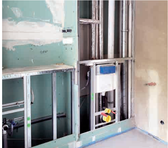
Service lines with inlet at floor level Image: PORR AG
