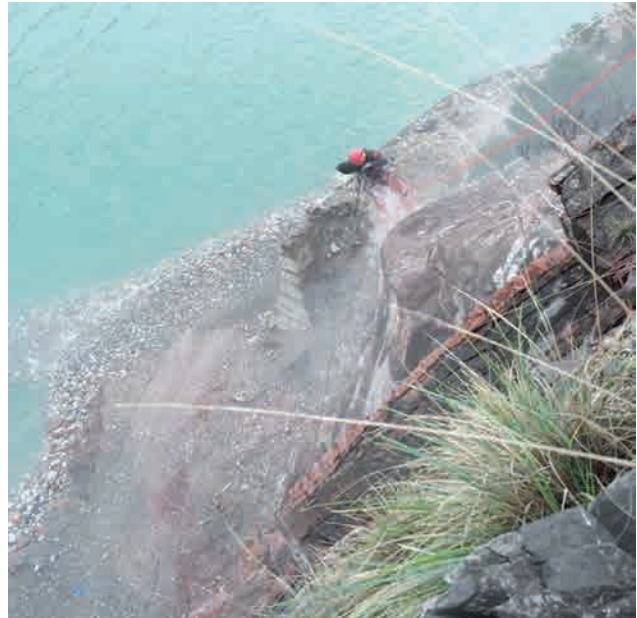
Creation of fixed points for safety cables Image: PORR AG
