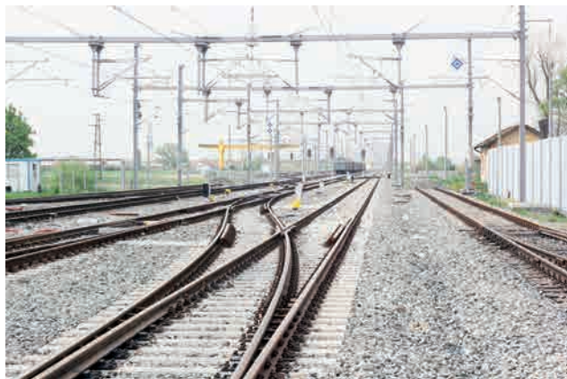
Newly laid tracks and switches as well as newly installed catenaries in Svilengrad
