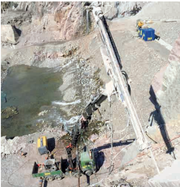
Creation of drill holes for the rock nails by means of drilling lorry Image: PORR AG
