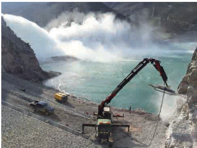
Rock stabilisation by means of wire nets at BVH Komani Dam in Albania Image: PORR AG
