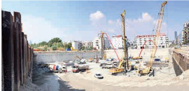
Development site 8, bore pile work protected by the diaphragm wall and sheet pile wall enclosure Image: PORR AG
