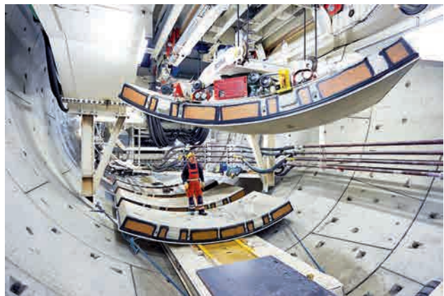
Tubing installation Image: Toni Rappersberger
