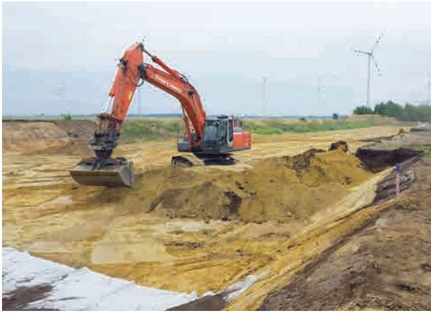
Earthworks on soakaway pits Image: PORR AG
