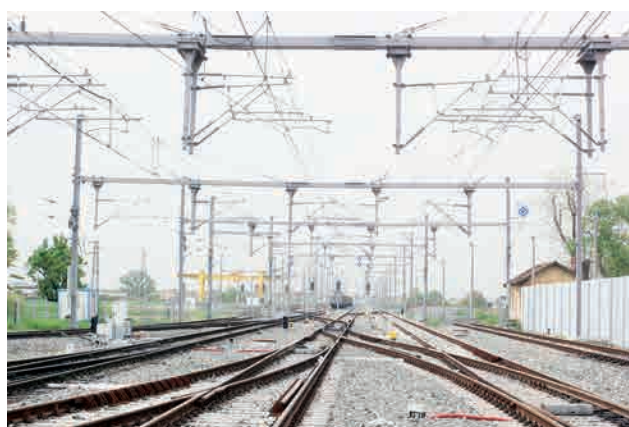
Newly laid tracks and switches as well as newly installed catenaries in Svilengrad Image: PORR AG
