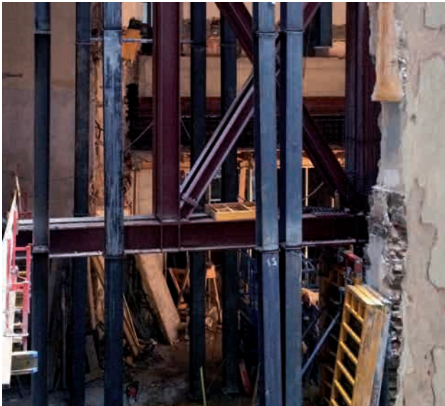
Underpinnings spanning two storeys Image: PORR AG
