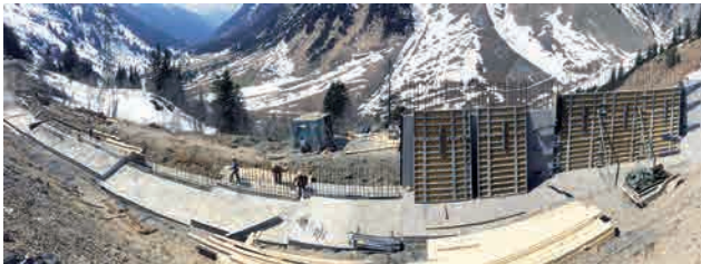
Support wall no. 2, under construction, June 2015 Image: PORR AG
