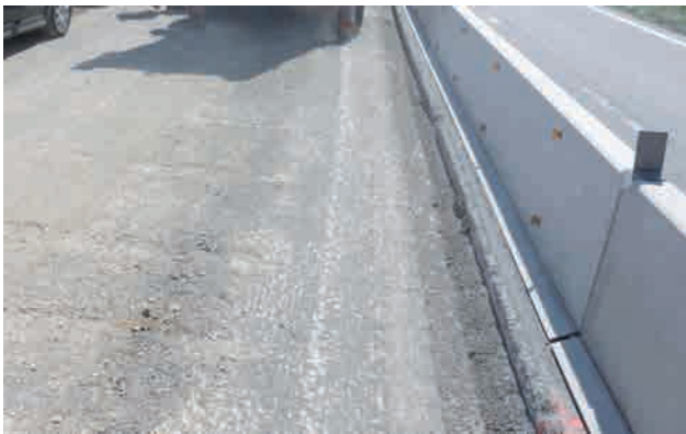
Surface after relieving stresses Image: PORR AG
