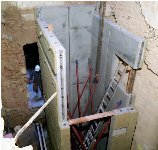
Lift made from pre-cast concrete parts Image: PORR AG
