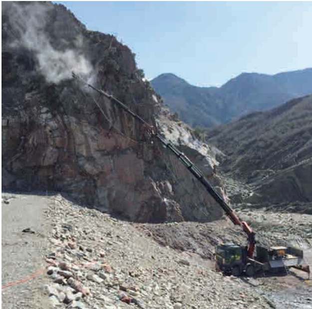
Creation of drill holes for the rock nails by means of drilling lorry Image: PORR AG
