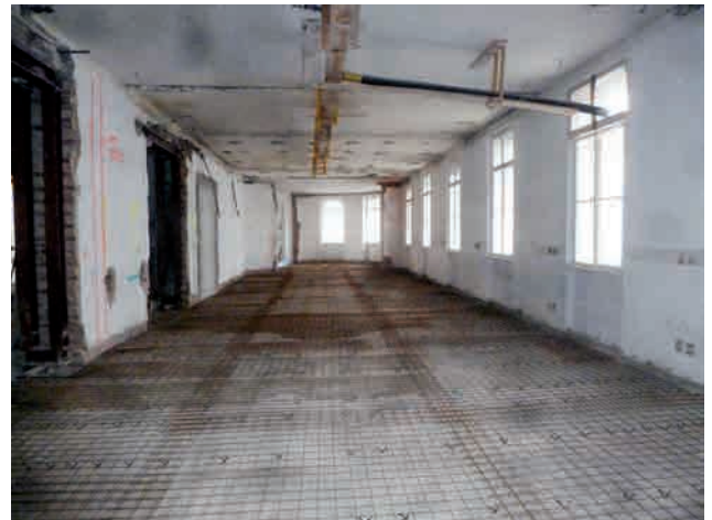
Timber-concrete compound ceilings Image: PORR AG
