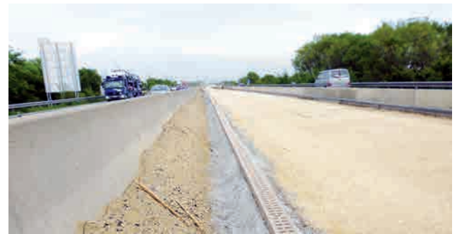
New relocated drainage gullies Image: PORR AG
