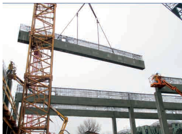
26 t semi-finished beam Image: PORR AG
