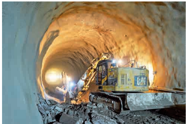
Bench cutting south tube Image: Toni Rappersberger
