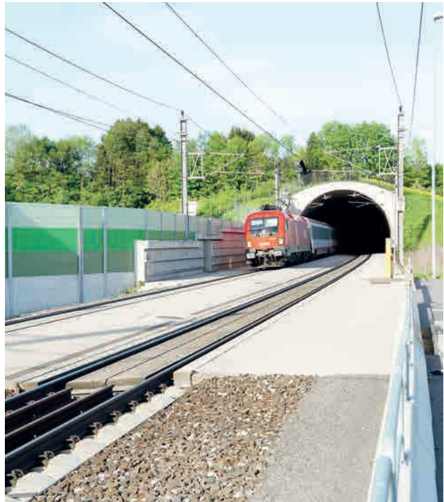
ÖBB-PORR slab tracks with load bearing sound-absorbing slabs Image: PORR AG
