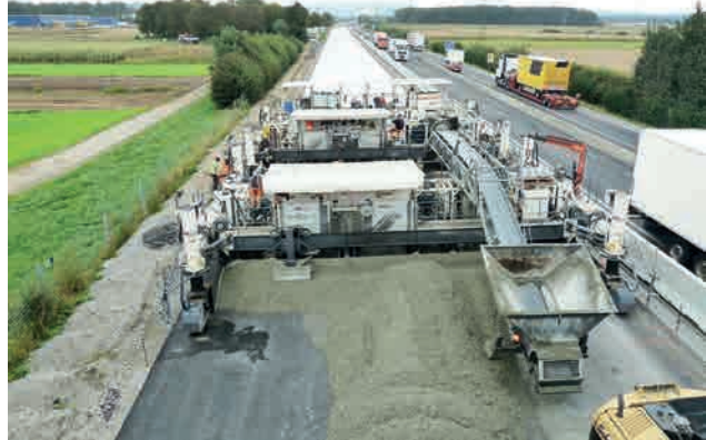
Concrete slab installation on A9 Pyhrnautobahn motorway in Austria Image: PORR AG
