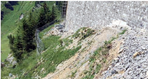
Support wall no. 2 with natural stone cladding, July 2015 Image: PORR AG
