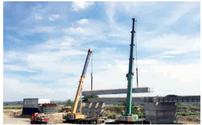
85-t prefabricated girders are lifted into place Image: PORR AG
