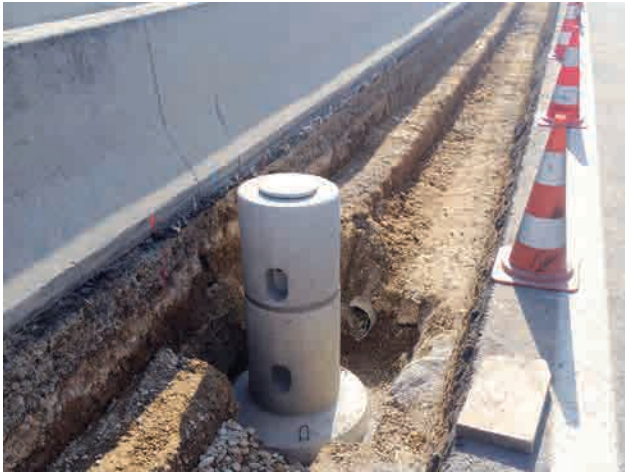
Earth works for lighting including lamp post foundations Image: PORR AG
