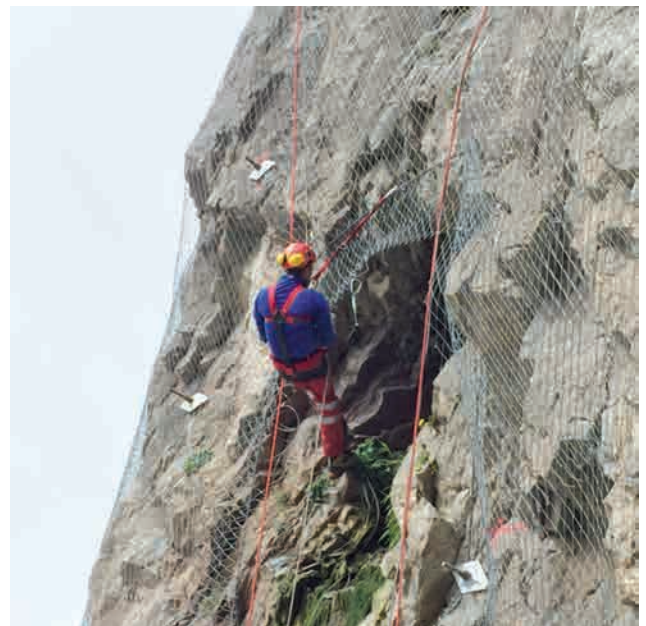
Completion of rock stabilisation by means of wire nets – working while suspended from ropes Image: PORR AG
