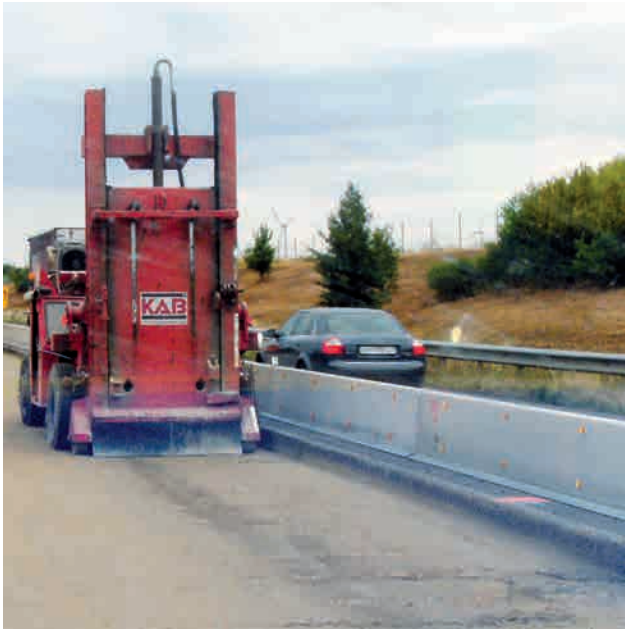
Relief using a shearing blade Image: PORR AG
