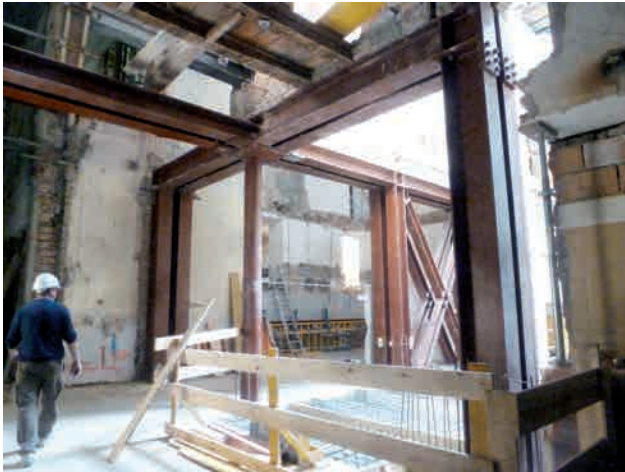
Underpinning of the reception hall Image: PORR AG
