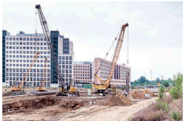
Diaphragm wall work Image: PORR AG
