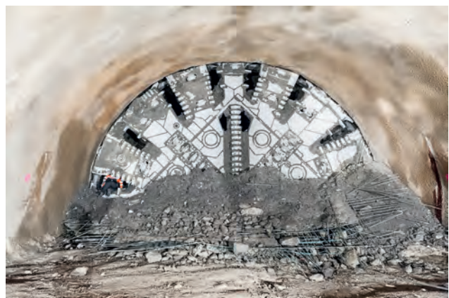
TBM driving through the exploratory section which had previously been executed conventionally in the Umpfen Valley intermediate attack. Image: ATA
