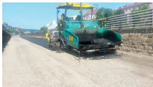
Installation of the bituminous base layer for drainage Image: PORR AG
