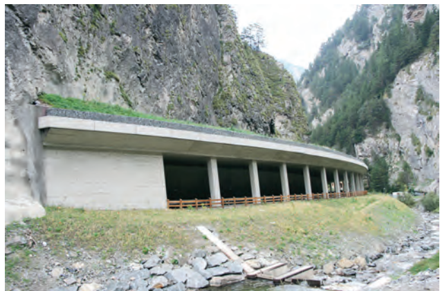
Connection of gallery structure with natural tunnel Image: PORR AG
