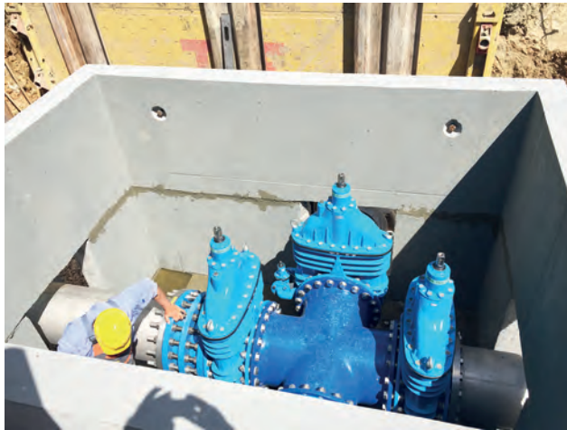
Branch shaft with fittings DN600 / 500 – assembly condition Image: PORR AG
