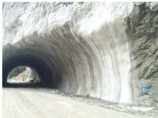
Natural tunnel – expanded and secured Image: PORR AG
