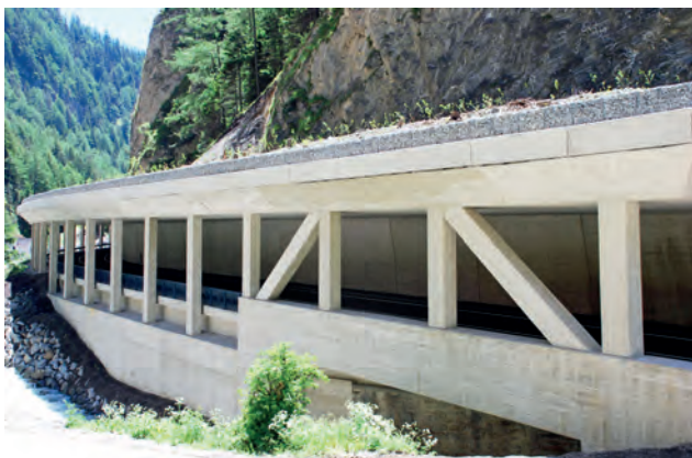
Incorporation of Stillerbach bridge into Niklasgalerie Image: PORR AG
