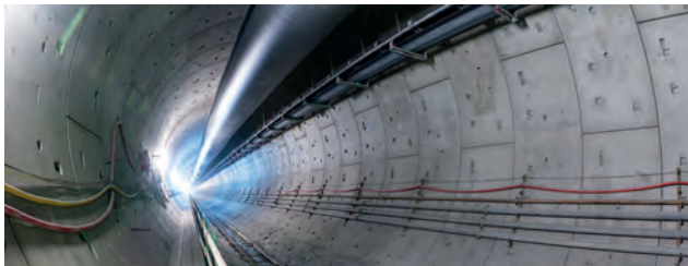
Tübbingausbau Boßler tunnel east tunnel 2016 Image: ATA
