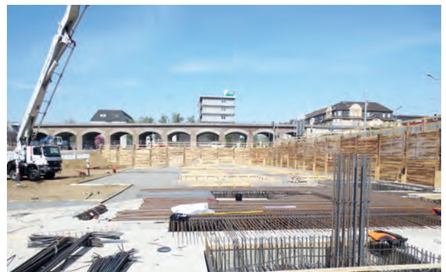
Flat foundation work Image: PORR AG
