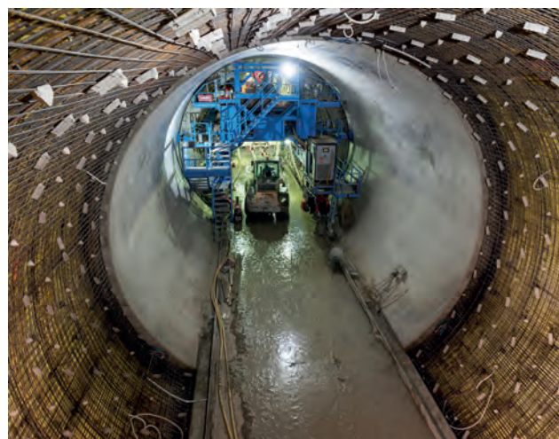
Reinforced concrete ring: d=45cm and block length=12.5m Image: ATA
