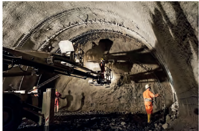
17,500m of shotcrete tube ... Image: ATA
