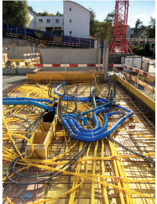
Ceiling inlays above the ground Image: PORR AG
