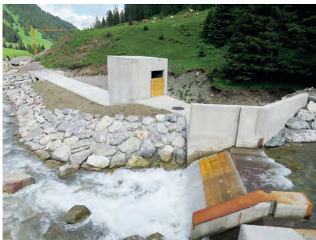
One of the two "Tyrolean Weirs" incl. sedimentation basin Image: PORR AG
