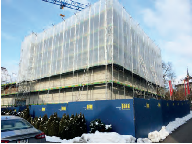
Enclosure of the facade as preparation for application of the window mosaic Image: PORR AG
