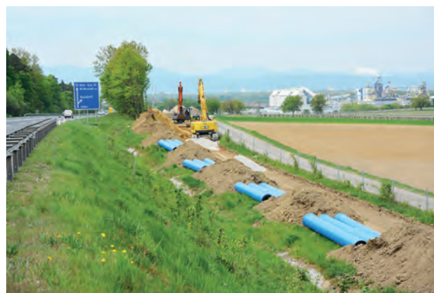
Cast line construction DN600 Neudörfl Image: PORR AG
