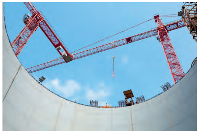
PEHD cladding in the shaft Image: PORR AG
