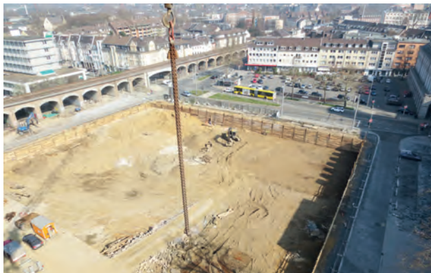
The construction pit with Berlin type pit lining Image: PORR AG
