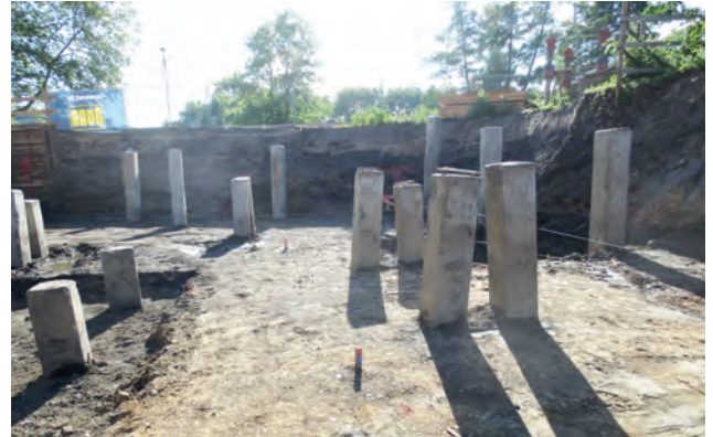
Driven pile foundations: The pile heads are still to be cut. Image: PORR AG
