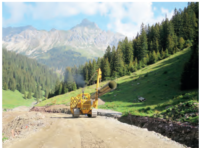
Delivery and laying of the pressure line Image: PORR AG
