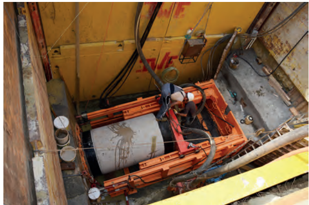
Micro-tunnelling launch shaft including hydraulic press frame Image: PORR AG
