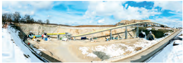
Steinbühl tunnel material conveying via the intermediate access Image: ATA
