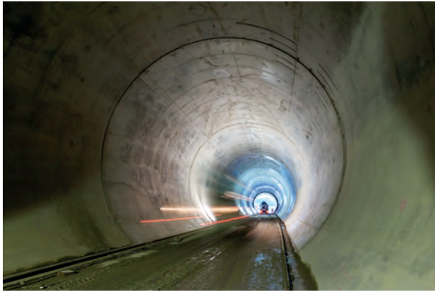
4.8km of completed inner lining prior to road surfacing Image: ATA
