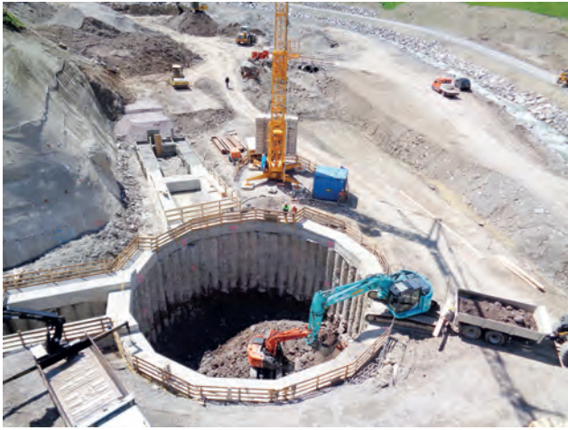
Excavation work for the powerhouse's construction pit Image: PORR AG
