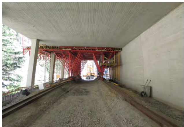
Gallery formwork carriage Image: PORR AG
