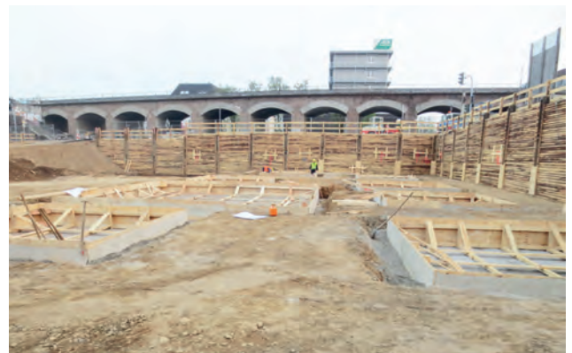
Individual foundations within the flat foundations Image: PORR AG
