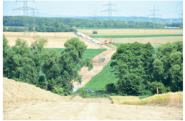
Pipeline route after humus removal in the Sigless area Image: PORR AG
