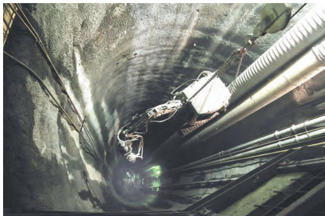
Exploratory shaft: Depth: 55m, diameter: 8m Image: ATA
