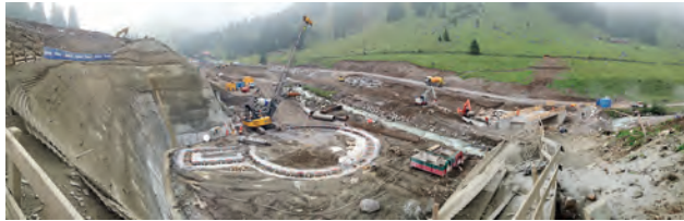
Bored pile work in the powerhouse area Image: PORR AG
