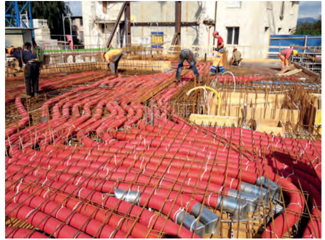
Ceiling inlays for the building services installations Image: PORR AG
