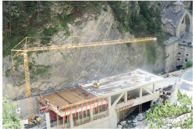
Construction of blocks 1 and 2 / Stillerbach bridge superstructure Image: PORR AG
