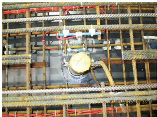
Comprehensive monitoring of all construction stages. In the picture: Measuring systems in the segment to determine utilisation ratio. Image: ATA
