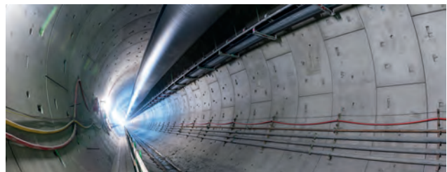
... become 17.500m of segment ring tube Image: ATA
