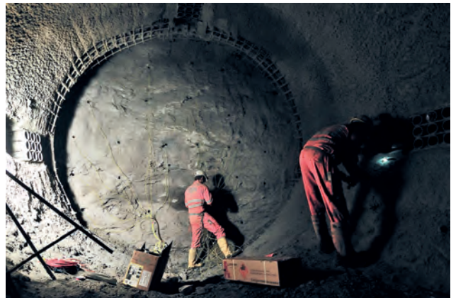
Exploratory gallery: Diameter: 3.6m. For the purpose of advance exploration of tunnel sections forecast to show squeezing rock Image: ATA
