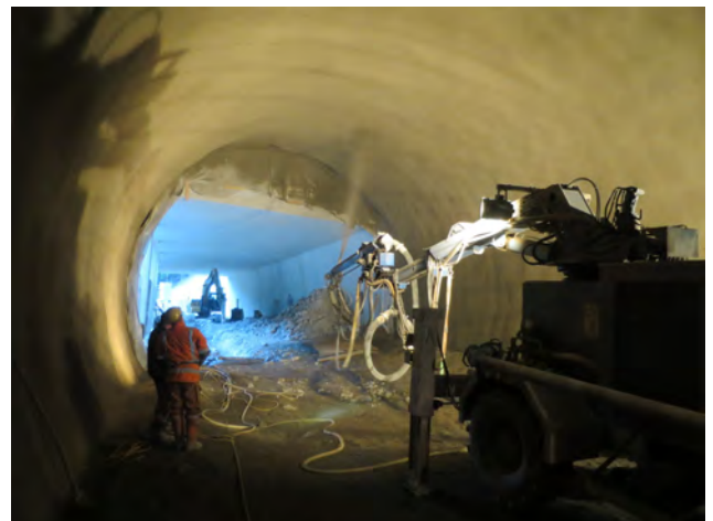
Inner lining – shotcrete shell natural tunnel Image: PORR AG
