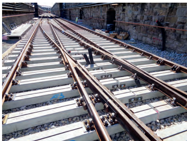
New points system Image: PORR AG
