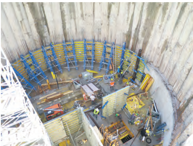
Single-sided wall construction – concreting to bored pile wall Image: PORR AG
