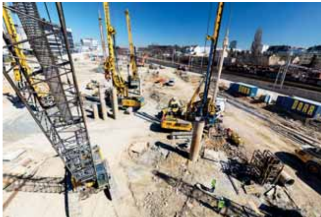
Construction of the bored pile walls enclosing the construction pit Image: PORR AG/Harry Schiffer
