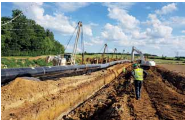
Pipe trench excavation Image: bayernets
