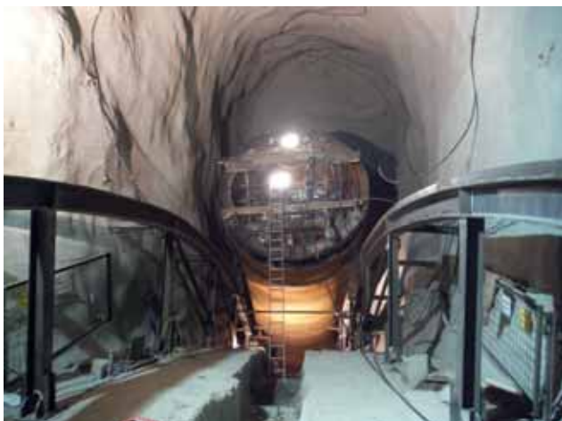
Pressure shaft, upper vertical elbow, installation of steel armouring, inside cross section 4.5 m Image: ARGE Bau OVWII
