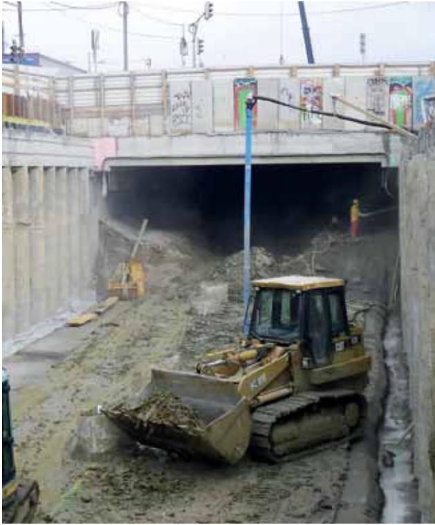
Construction pit excavation in the transition from open cutting to a covered section Image: PORR AG
