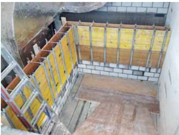
New lift shaft with a riser shaft behind it Image: PORR AG
