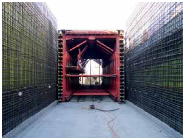
Inner layer reinforcement in the region of track 2, with formwork carriage Image: PORR AG
