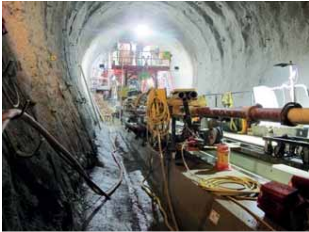
Silvretta tunnel, interior construction, advance excavation bed tubing, trailing formwork carriage for the vault Image: ARGE Bau OVWII
