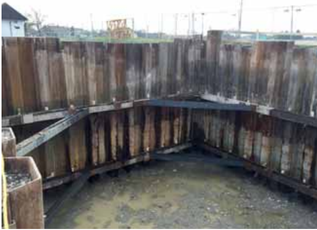
Watertight construction pit with sheet-pile walls and two reinforcements Image: PORR AG
