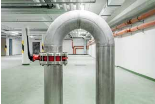
Scheduled, controlled flooding of the 2nd basement floor by flooding wells and pipes. Shut-off valves on the pipelines prevent flooding of the first basement floor with the technical installations
