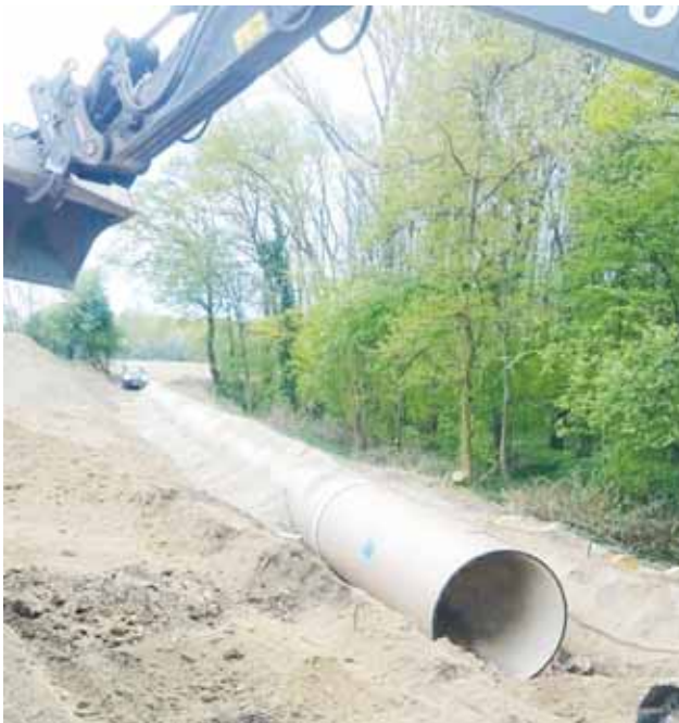
Laying the sewer overflow pipes near the Traismauer sewage treatment plant Image: PORR AG
