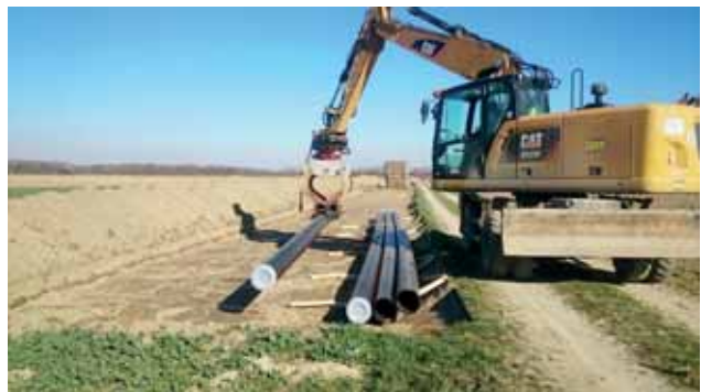
Handling the pipeline (section length 16 m) with an adapted sorting grapple on a mobile excavator Image: PORR AG
