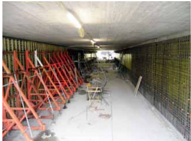
Shuttering and reinforcement works on the inner layers below the roof Image: PORR AG
