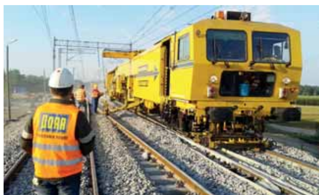
Regulation and plugging of switches on the main railway line LK 4 in Biała Rawska Image: PORR AG
