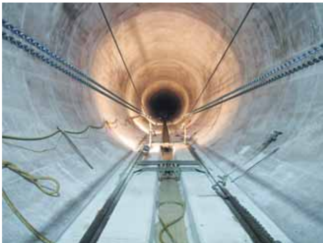
Silvretta tunnel, unreinforced concrete inner shell, cross section 6.80 m, longitudinal incline 9 %, rear-mounted vault formwork carriage Image: ARGE Bau OVWII
