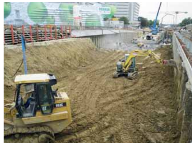
Excavation between bored piles with jetcrete and concrete structures subsequently added Image: PORR AG
