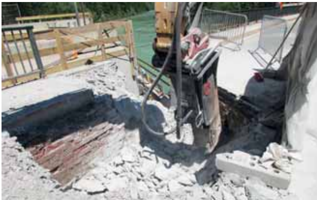
Removing the bridge Image: PORR AG
