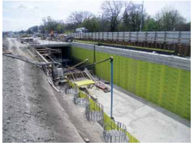
Open cutting with lost shuttering for concreting the spandrels between bored piles Image: PORR AG
