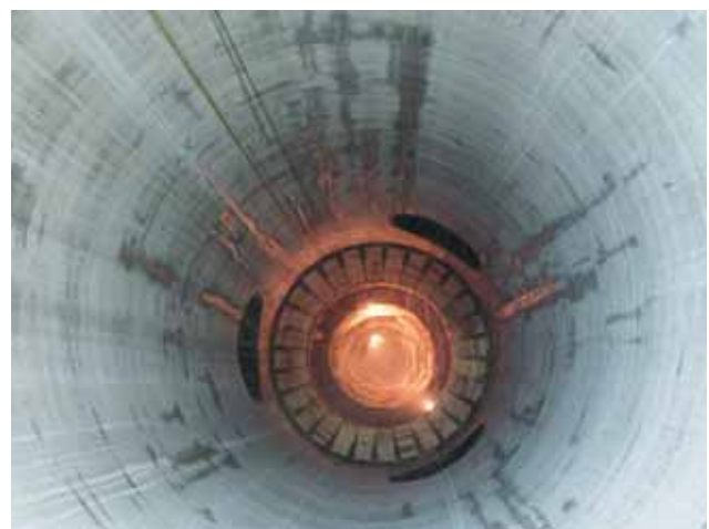
Krespa waterlock, riser duct, inner shell completed by slip-form method, inner cross-section 17 m, three branching and lower chambers, equipped warping section Image: ARGE Bau OVWII
