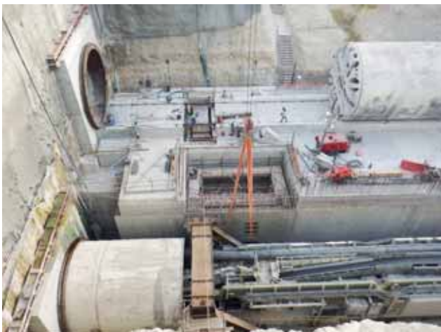
Transfer in the switchbox Image: PORR AG
