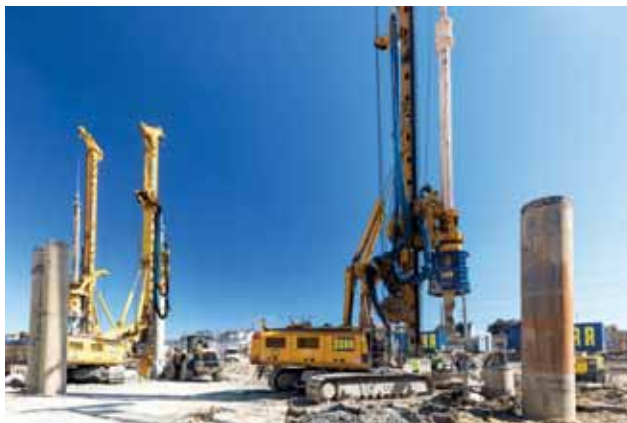
Construction of a cut-out bored pile wall near the tunnel Image: PORR AG/Harry Schiffer
