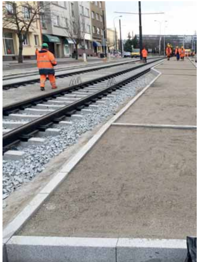
Kubánské náměstí stop (city-bound). Completion of the concrete bedding layer C 20/25. Preparation for mounting of the railings and canopy before installation of the mastic asphalt, separating and top layers (MA8). Image: PORR AG
