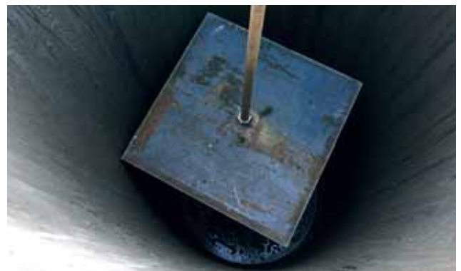
Installation of an auxiliary support Image: PORR AG
