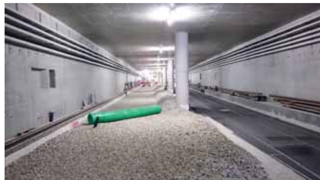
Installation of sound insulation mats and ballasted track underground Image: PORR AG
