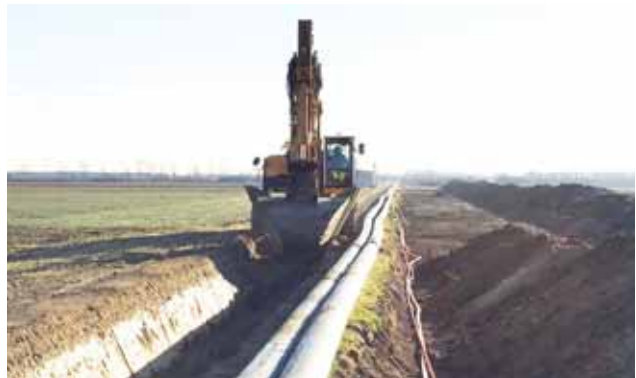
Laying the pre-welded HDPE pipelines Image: PORR AG
