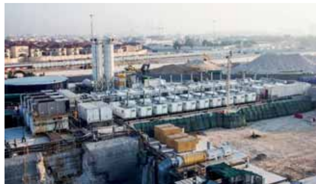
Diesel generators, starting shaft at Al Messila Image: PORR AG
