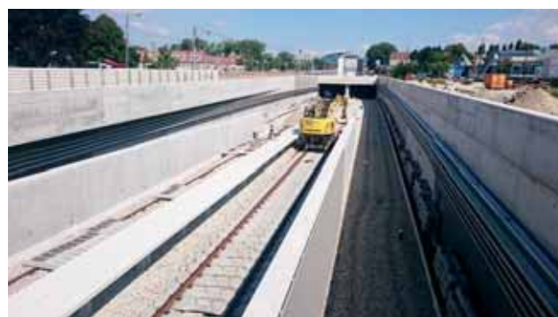
Track construction works around the open track Image: PORR AG
