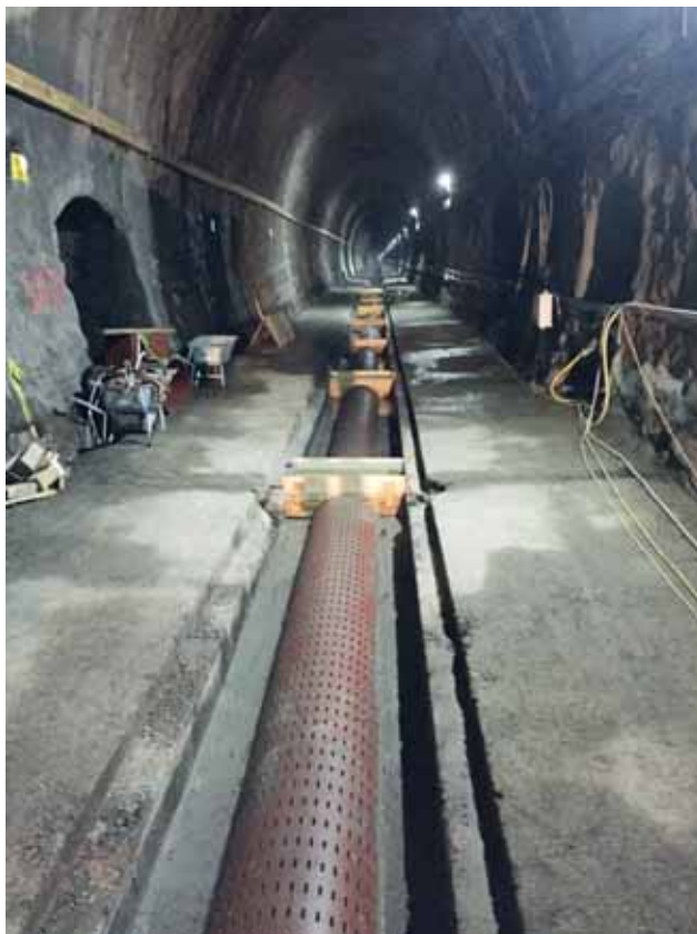
Pipe work of the sole flue Image: PORR AG
