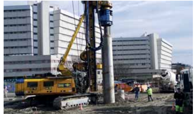
Bored pile construction works for U1/13 between Favoritenstraße and Per-Albin-Hansson-Siedlung Image: PORR AG
