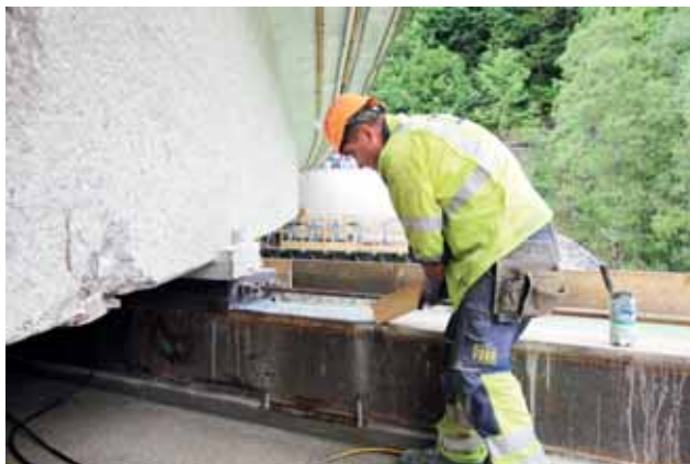
Preparations for the sideways shunt Image: PORR AG
