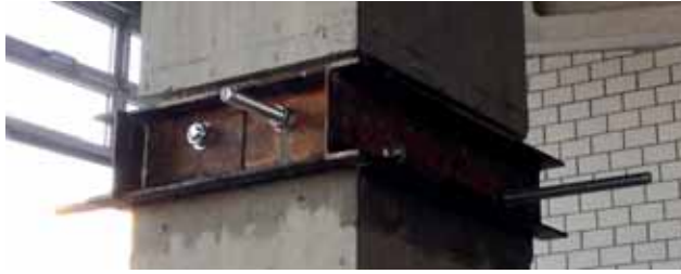
U-section with threaded rod through existing column Image: PORR AG
