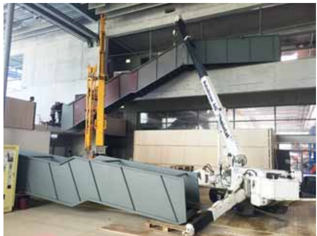
Installation of the steel staircase Image: PORR AG
