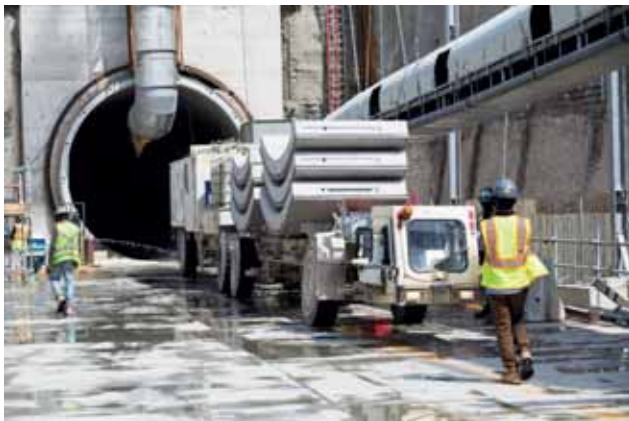
Tubbing transport with Multi-Service-Vehicles Image: PORR AG
