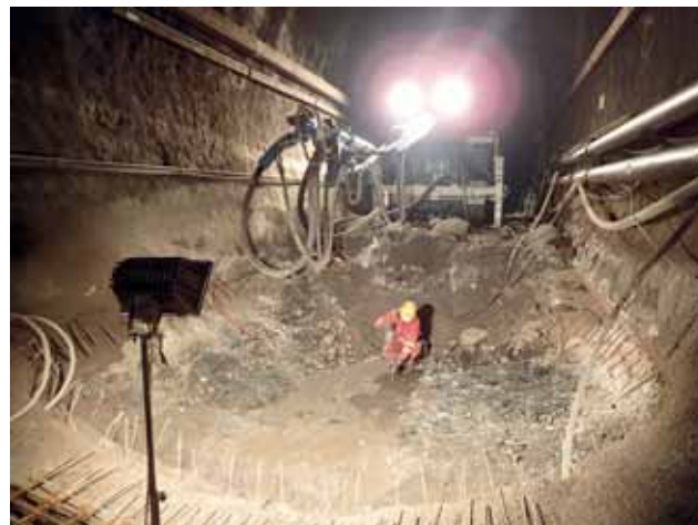
Base section prior to SpC Image: PORR AG
