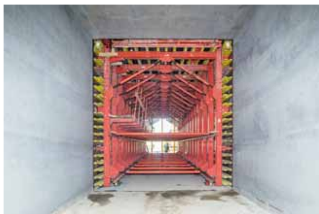
Concreted right-angle cross-section with formwork carriage Image: PERI
