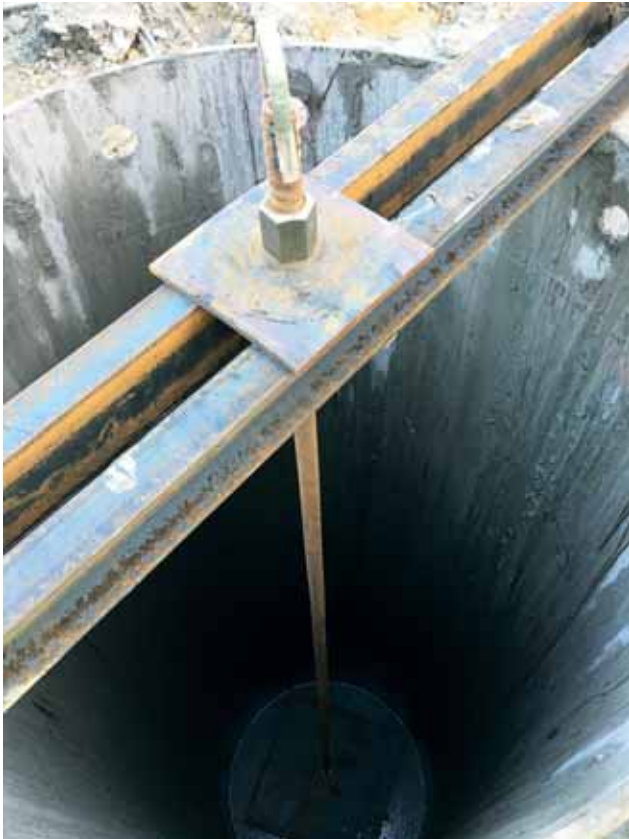
Installation of an auxiliary support Image: PORR AG
