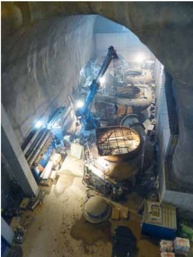
Transformer cavern, location for pre-assembly of pump and turbine spirals Image: ARGE Bau OVWII
