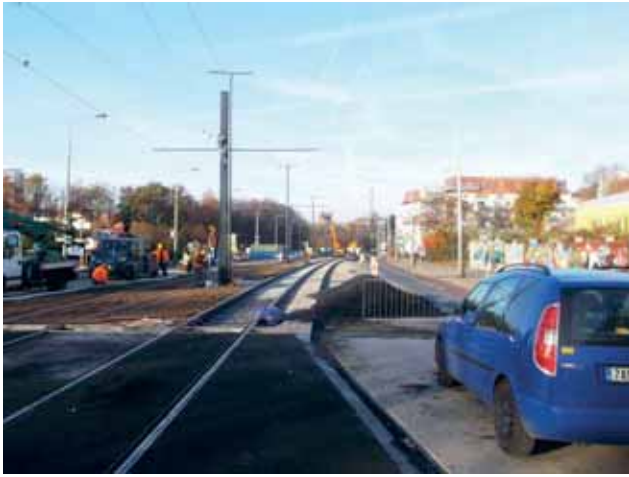
Finishing work on the overhead line and distribution of the topsoil for the future grass cover of the tram section between the stops Nádraží Vršovice (city-bound) – Otakarova.
