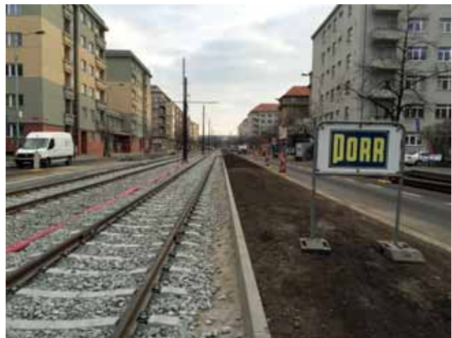
Section of the tram line from Slavia stop (coming from the city centre) – Kubánské náměstí. Tamping complete, preparation for the introduction of the topsoil for the future grass surface on the tram tracks. Image: PORR AG
