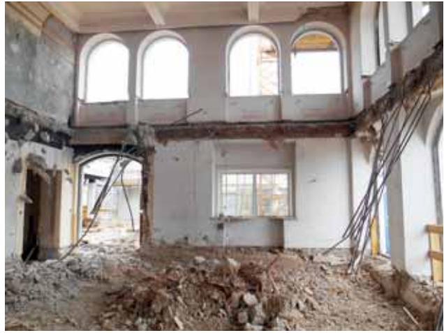
Demolition of the ceilings Image: PORR AG
