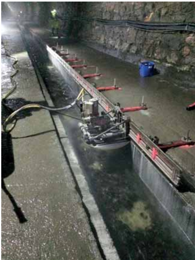
Cutting supports Image: PORR AG
