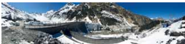
Installation of the main construction site, at the foot of Vermunt reservoir dam: Material processing, gravel works, two concrete mixers, a concrete laboratory, workshops, storage facilities Image: ARGE Bau OVWII
