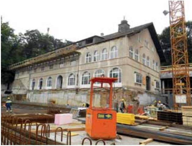
Hotel building after underpinning works and excavation of the underground garage Image: PORR AG
