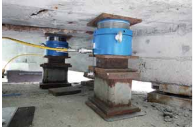
Jacks for raising the old bridge Image: PORR AG
