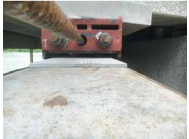
Shunt structure including shunt sledges, consisting of a layer of stainless-steel sheets mounted on Teflon slabs Image: PORR AG
