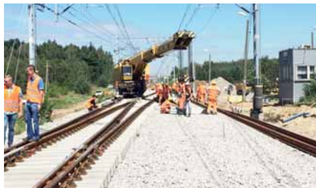
Switch assembly on the main railway line LK 4 in Biała Rawska Image: PORR AG
