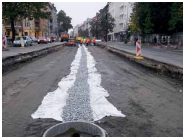
Reconstruction section of the base course around the future Bohemians tram stop (city-bound). In the middle of the track body construction, drainage pipe DN 150 is laid in a sand bed, with the separation geotextile and ballast fill, grain size 16/32.
