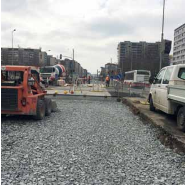
Finishing works on the crossing, consisting of prefabricated reinforced concrete slabs at the junction Vršovická - Bělocherkevská. Completion of the ballast bedding layer – grain size 32/63 – for laying of the sleepers. Image: PORR AG
