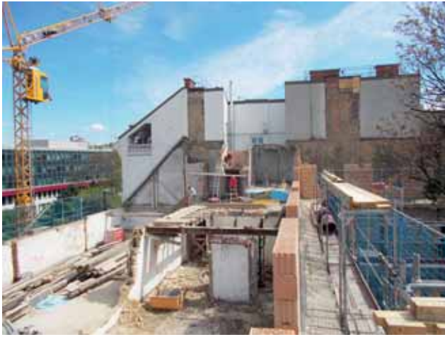
Demolition of the old roof truss and the ceilings Image: PORR AG
