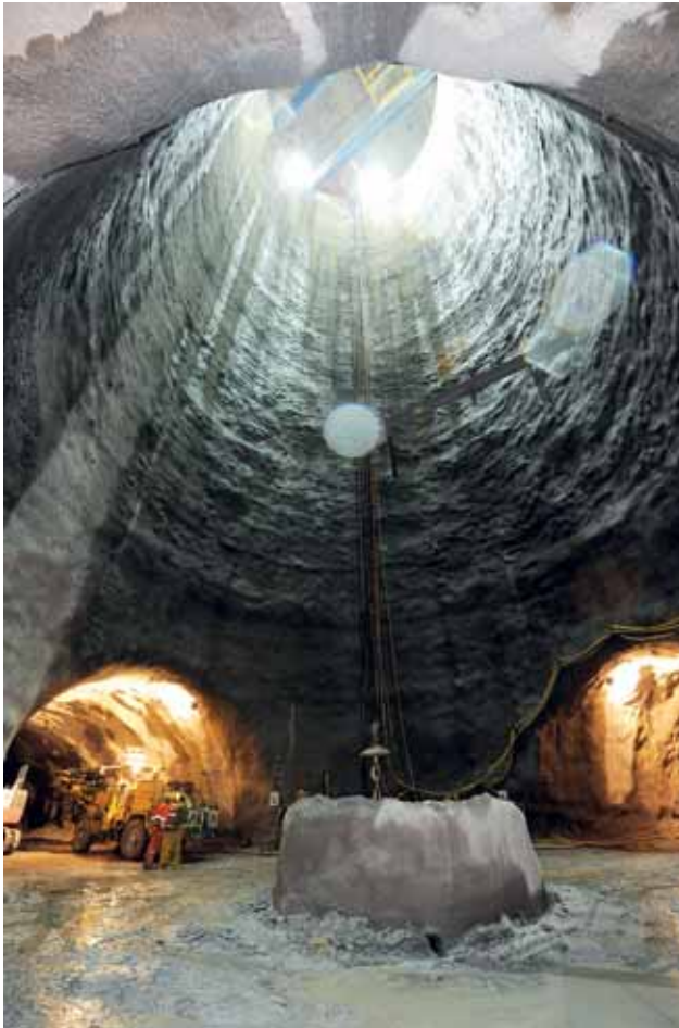
Krespa waterlock, excavated riser duct, tunnel crown excavation, lower chambers in progress Image: VIW
