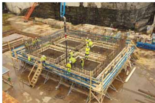
Construction of a bridge foundation at the drydock Image: PORR AG
