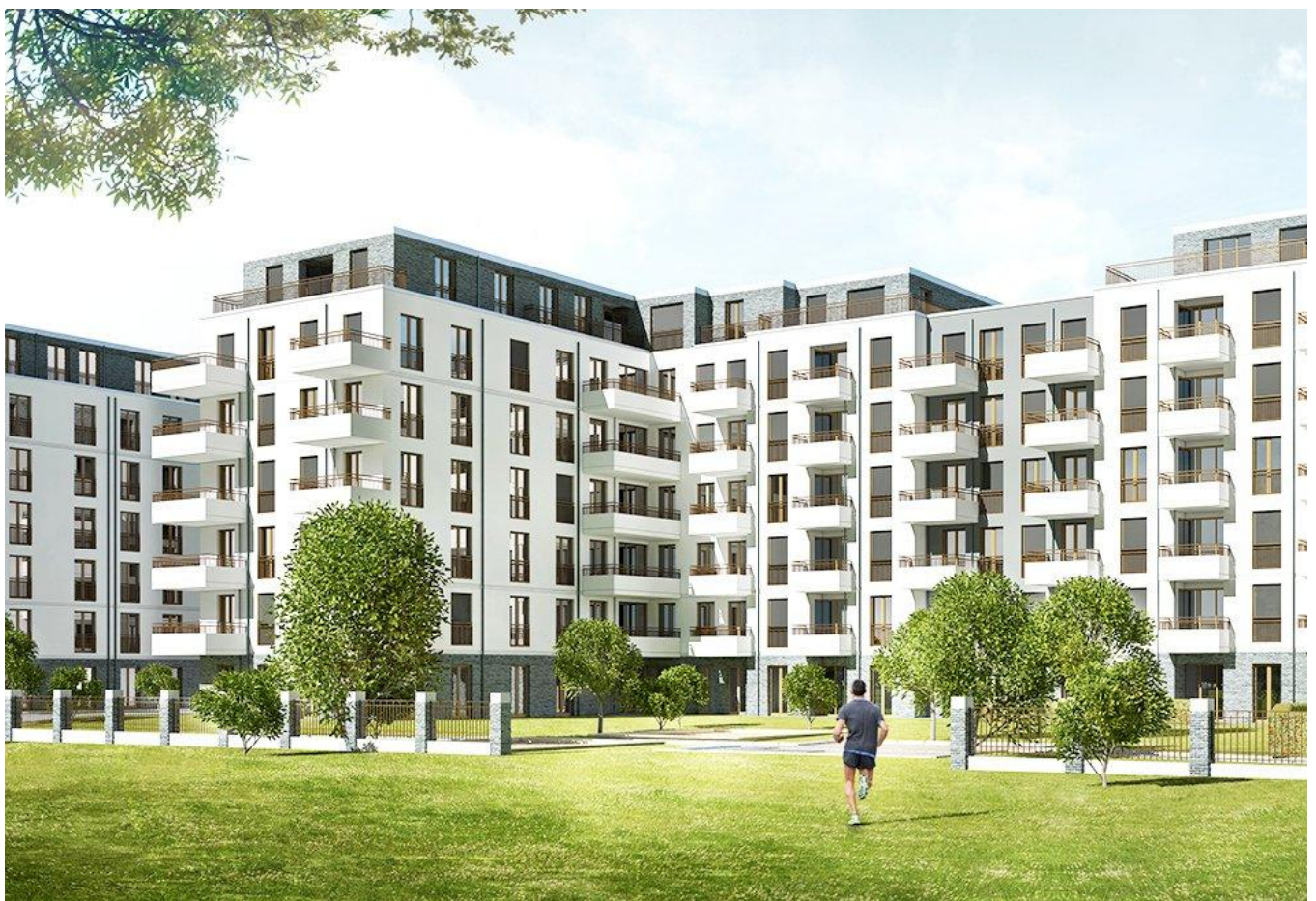
Modern housing complex in the Berlin district of Neukölln. Image: PORR Design & Engineering Deutschland GmbH
