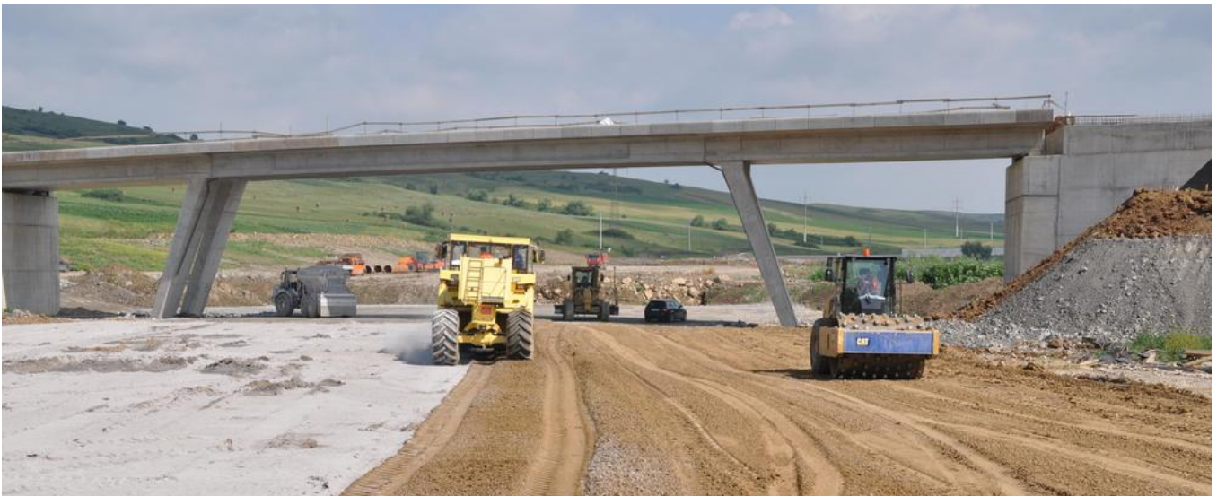
Demolished concrete surface with cleaned central line markings. Image: PORR AG
