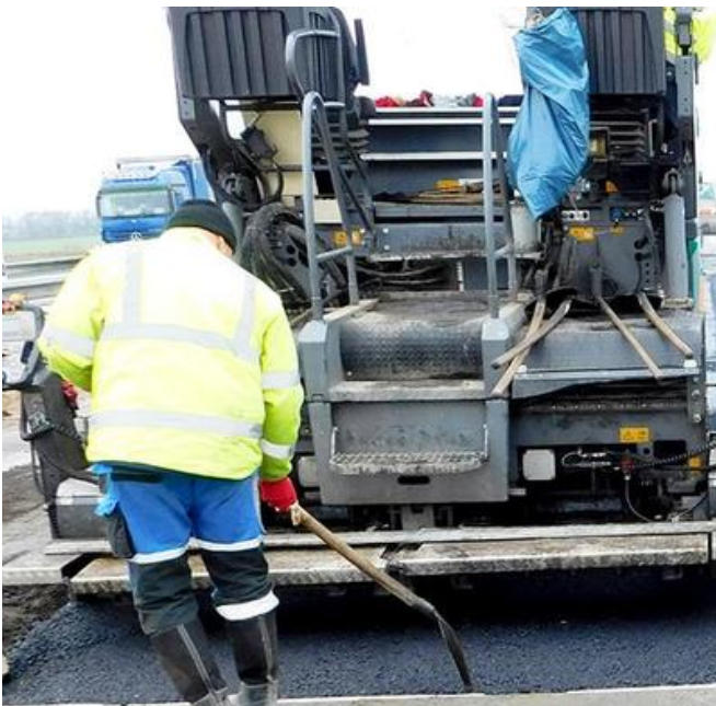
Laying of the compacted bitumen intermediate layers. Image: PORR AG
