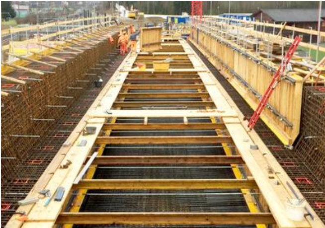
900m 3 of construction concrete was required for the construction of one section of the rail bridge. Image: PORR AG
