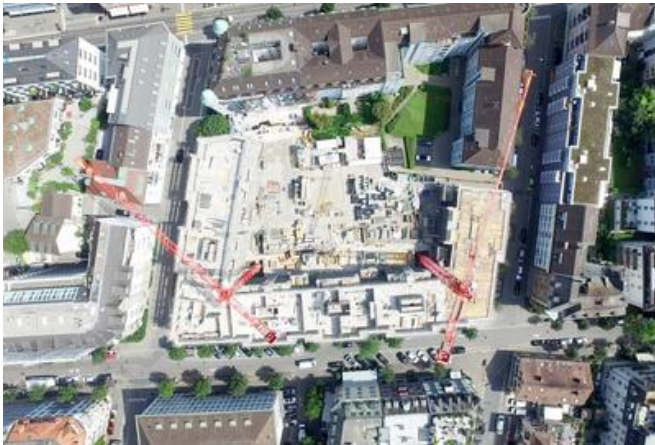
A bird's-eye view of the construction site. Image: PORR AG
