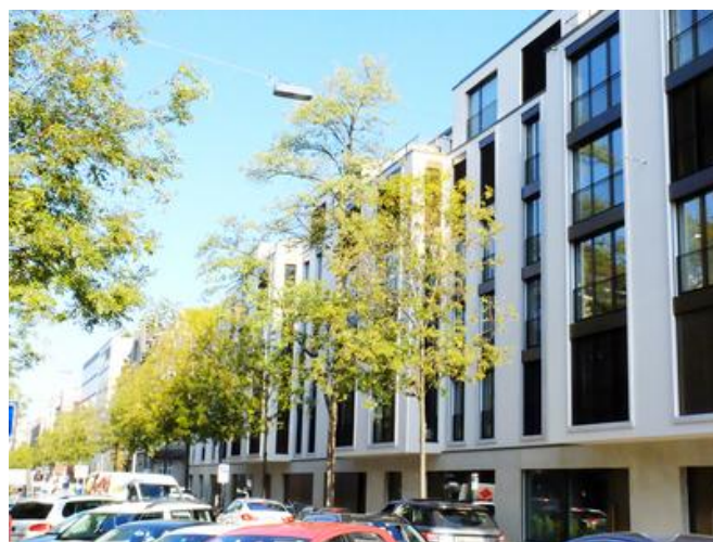
The orientation of the building allows a partial view of the lake from the upper floors. Image: PORR AG
