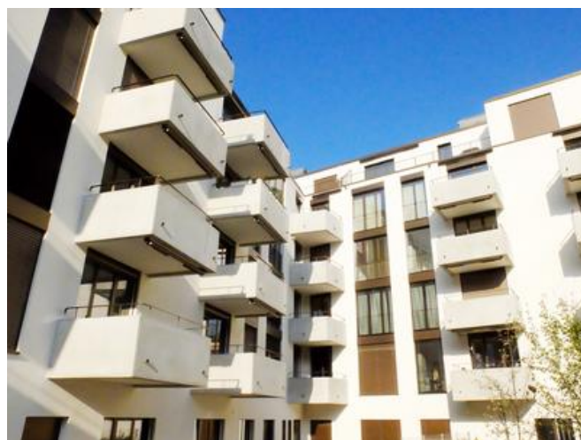
The project was completed in compliance with Swiss Minergie standards and therefore boasts higher energy efficiency than that mandated by law. Image: PORR AG
