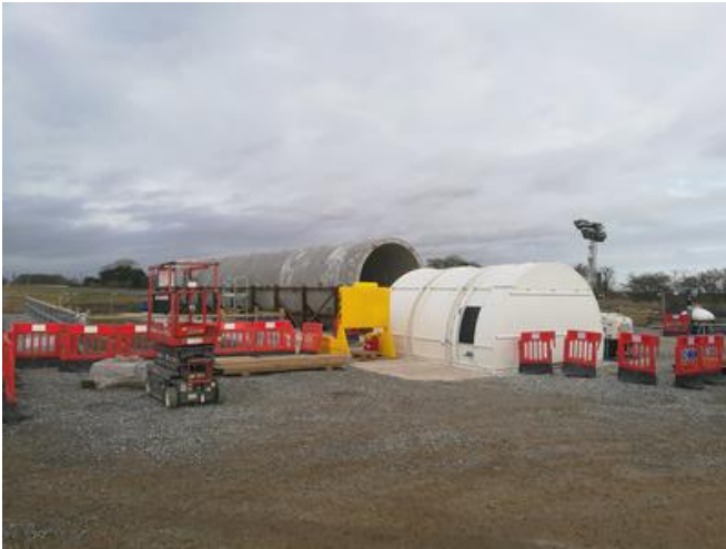
The tunnel mock-up for training purposes. Image: PORR AG
