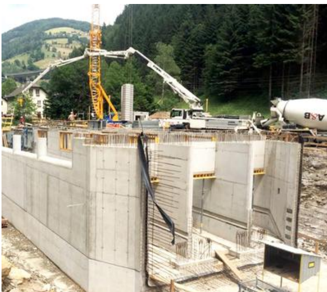
Concreting works on the three-chamber sand trap. Image: PORR AG
