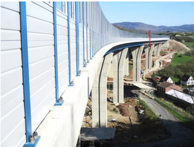
In spring, the final bridge sealing work and protective measures such as the noise protection wall were completed for partial structure 1. Image: PORR AG
