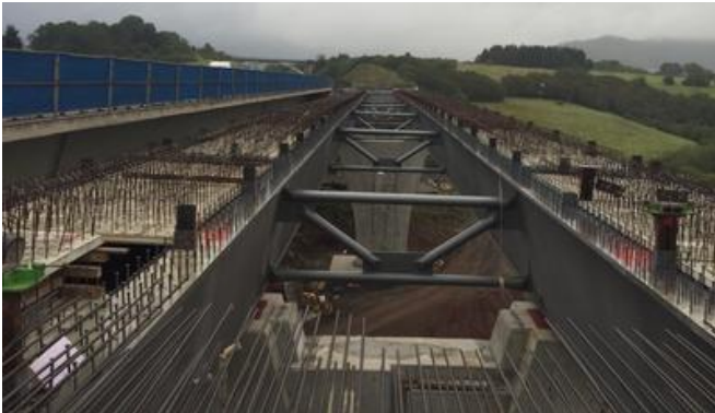
The shifted steel construction in its final location on the bridge columns. Image: PORR AG
