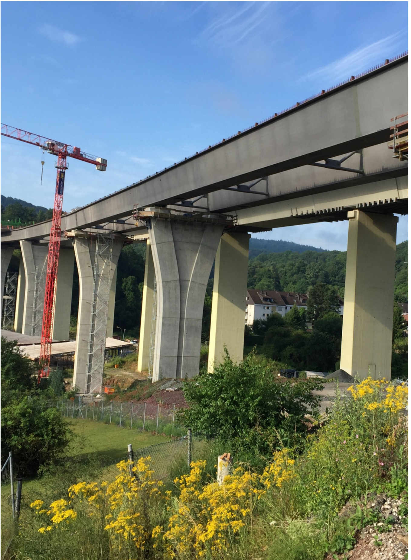
Manufacturing the new roadway slabs with the formwork carriage. Image: PORR AG
