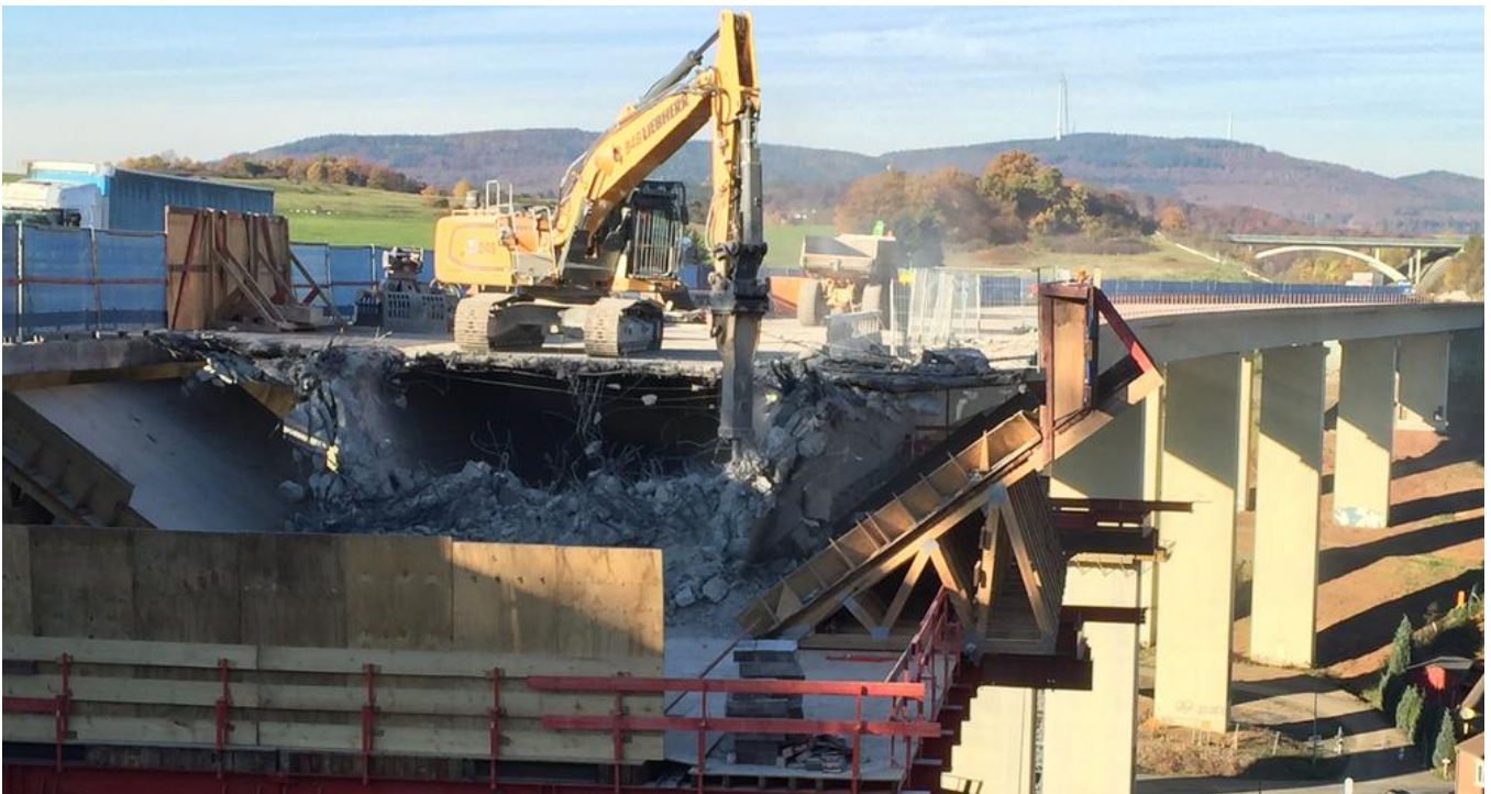
The demolition work was carried out using excavators. Image: PORR AG
