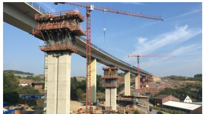
The new bridge columns, axis 50 and 60, are between 15.5m and 35m high and were concreted in individual sections of 5m each. Image: PORR AG
