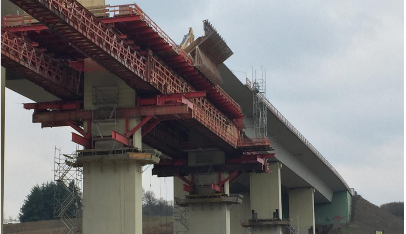
Demolition of the prestressed concrete box girders on the demolition scaffold. Image: PORR AG
