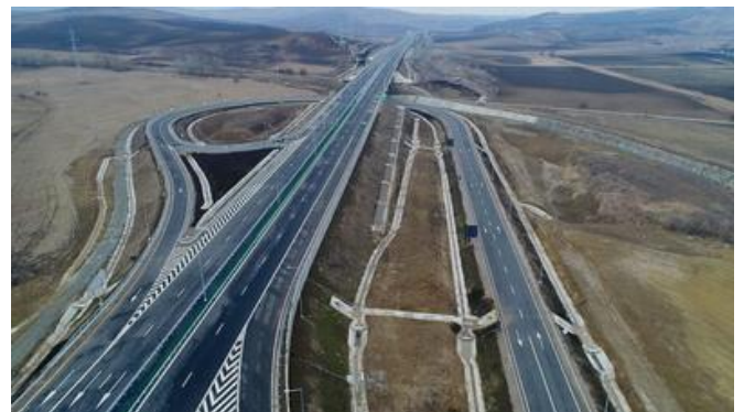
A glimpse of the comprehensive drainage measures included in the project. Image: Pro Infrastructura
