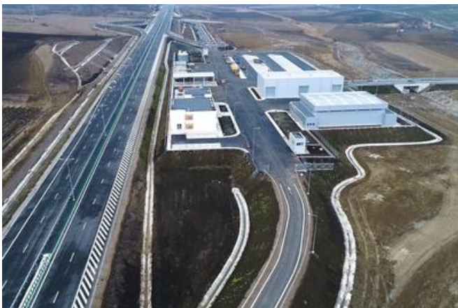
The road maintenance centre right next to the mothe new motorway rest areas. Image: Pro Infrastructura
