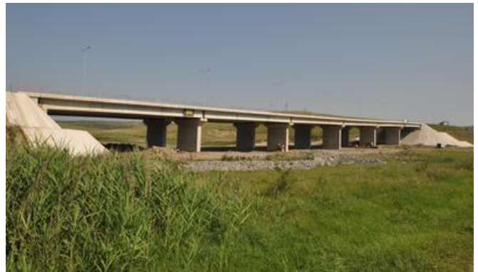
The 255m motorway bridge in Sector 5 is the longest bridge in the project. Image: PORR AG
