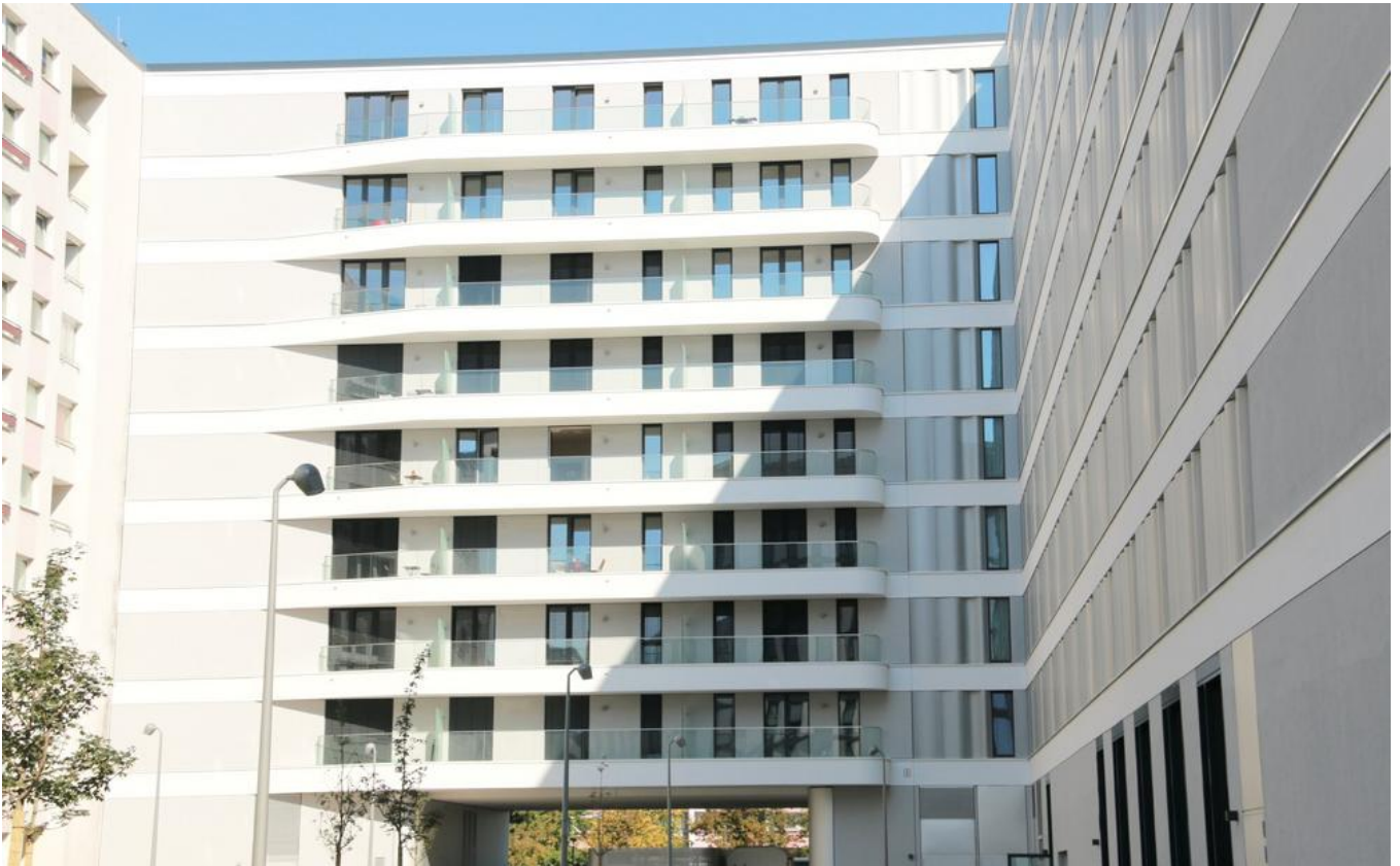
Front elevation of the apartment building. Image: PORR AG
