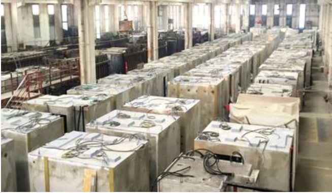
Production of the prefabricated bathroom pods out of reinforced concrete. Image: PORR AG
