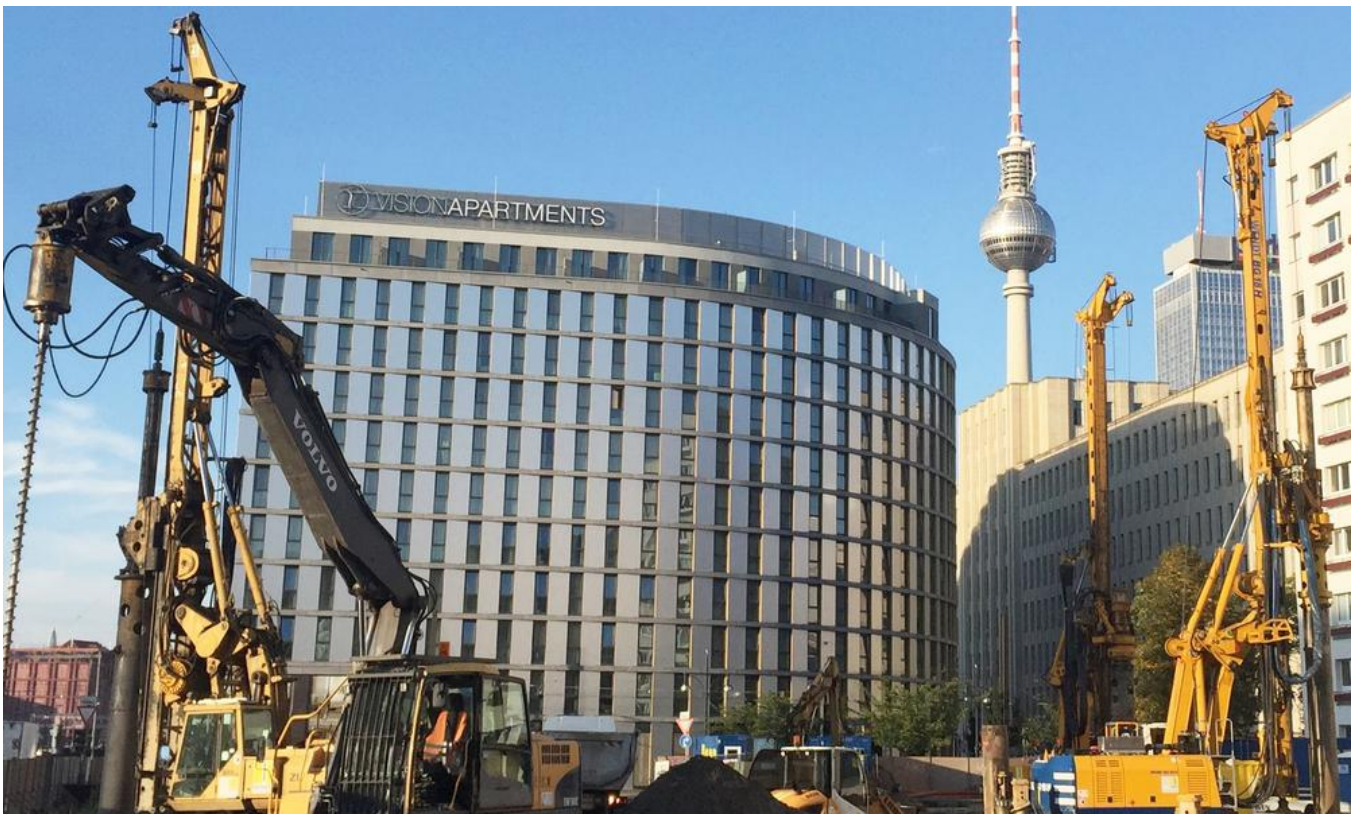
Large drilling equipment making the foundation piles. Image: PORR AG
