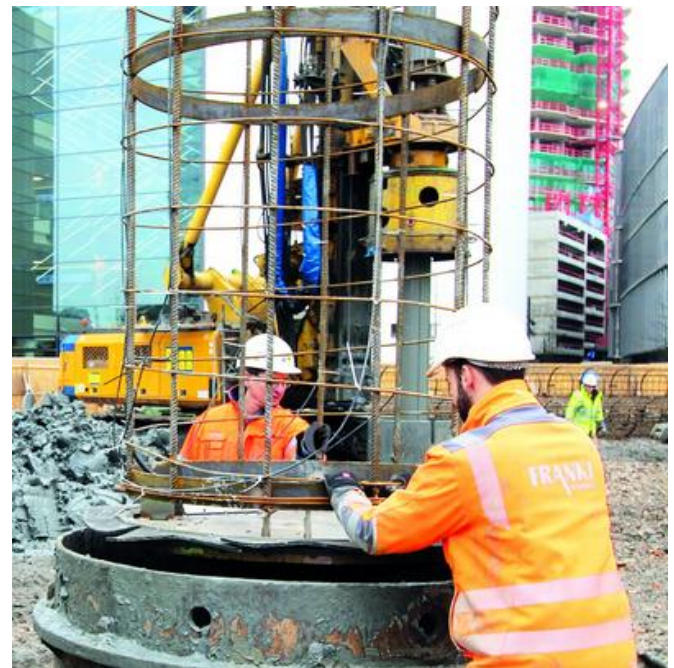
Inserting the reinforcement cage, which has been fitted with measurement instruments, into the pipe system. Image: isg
