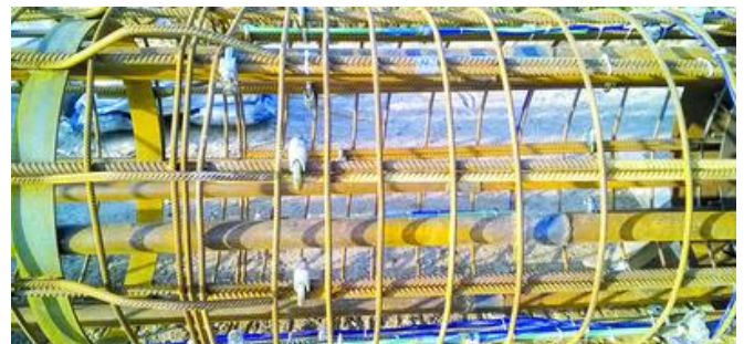
Reinforcement cage fitted with expansion sensors. Image: isg
