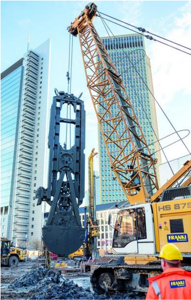
A diaphragm wall grab against a backdrop of Frankfurt's high-rise buildings. Image: FRANKI
