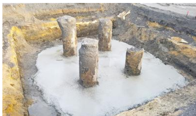
Exposed pile head with blinding layer. Image: FRANKI
