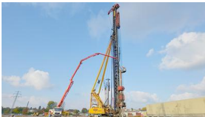
Concreting the simplex driven cast-in-situ concrete piles. Image: PORR
