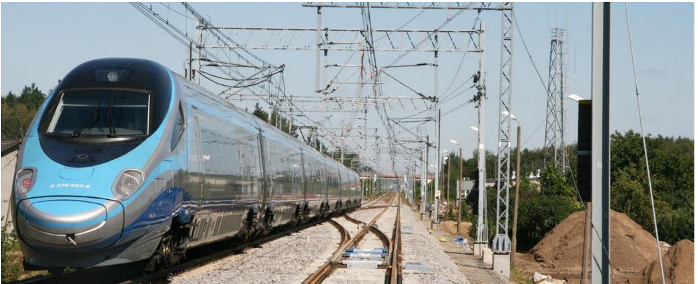
A train passing along the refurbished tracks at the Biała Rawska crossover. Image: PORR AG
