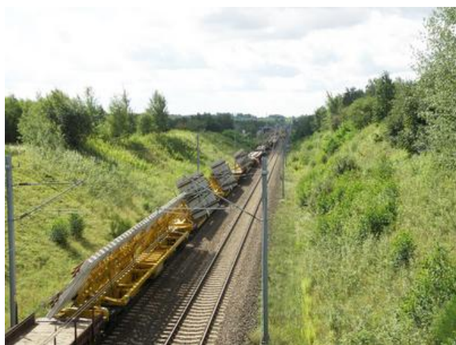
Transporting the switch blocks. Image: PORR AG
