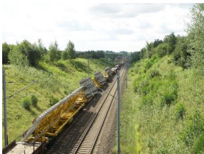
Transporting the switch blocks. Image: PORR AG
