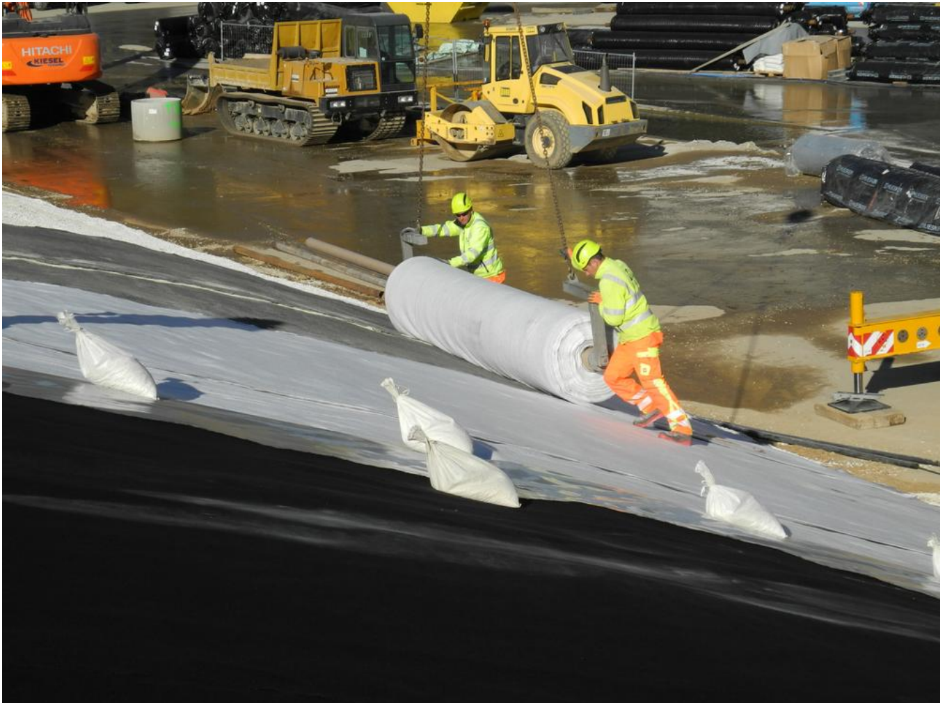
Laying the surface seal. Image: IAT GmbH
