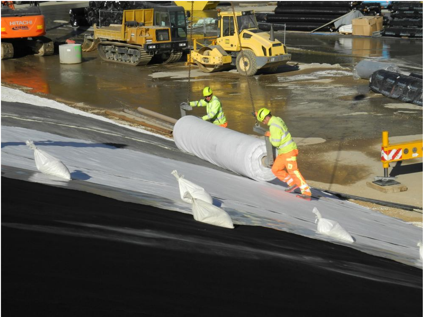
Laying the surface seal. Image: IAT GmbH
