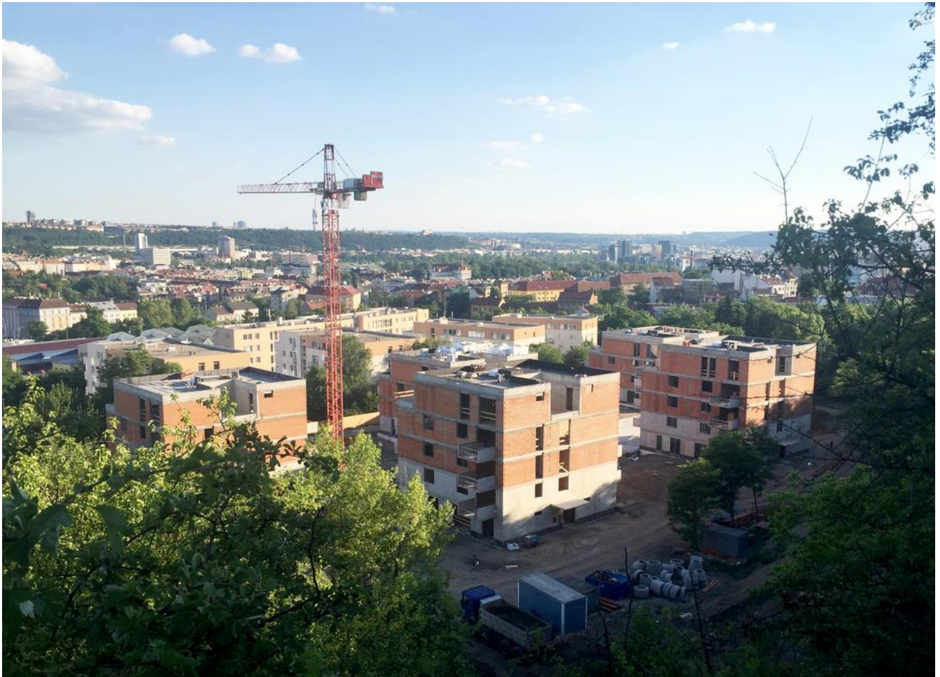
The shell of the new residential complex. Image: PORR AG
