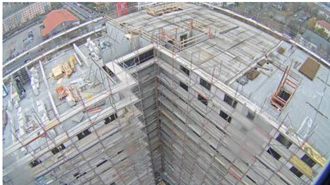
The student residence superstructure was built using crosswall construction. Image: PORR AG
