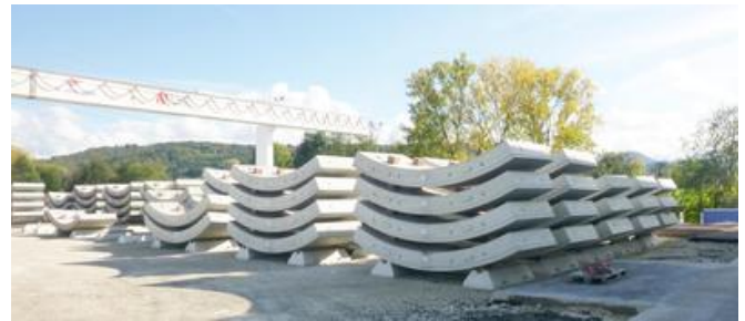
The segments are delivered by rail to an interim storage site in Frankfurt. Image: PORR AG
