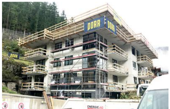
All the load-bearing walls and ceilings of the apartment hotel were made of reinforced concrete. Image: PORR AG
