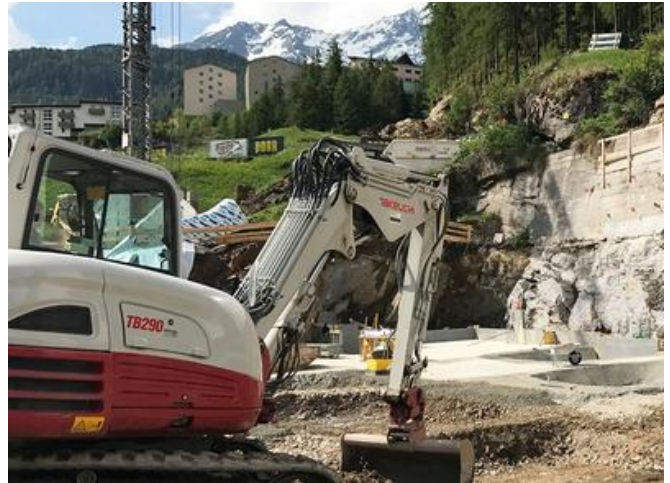
The construction pit was secured with jetcrete. Image: PORR AG
