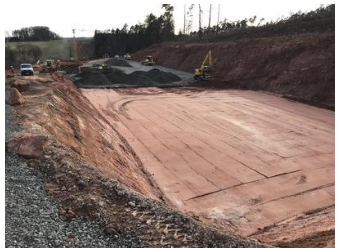
Around 25,000 m 3 of earth had to be excavated for the
