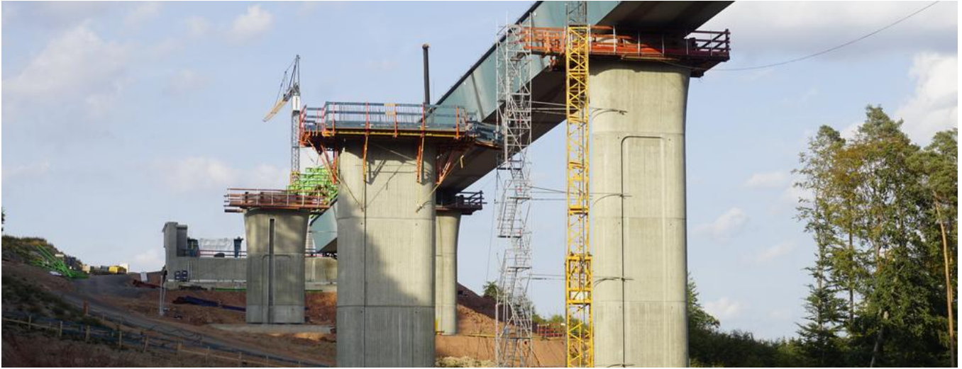
The columns have a height of just 30 m. Source: PORR
