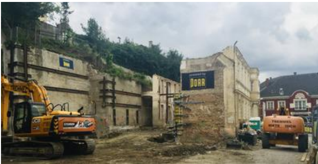
Considerable effort went into securing the church mound's retaining wall and the structured Gründerzeit façade. Source: PORR
