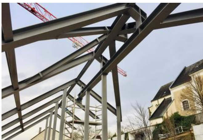
The new roof framework required a steel construction as the uppermost cornices of the old town hall featured a rooflight throughout. Source: PORR
