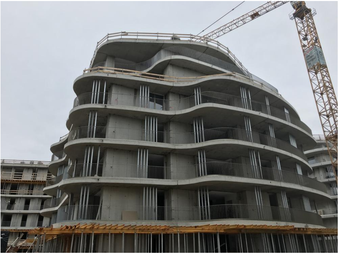
The completed project. Source: PORR
