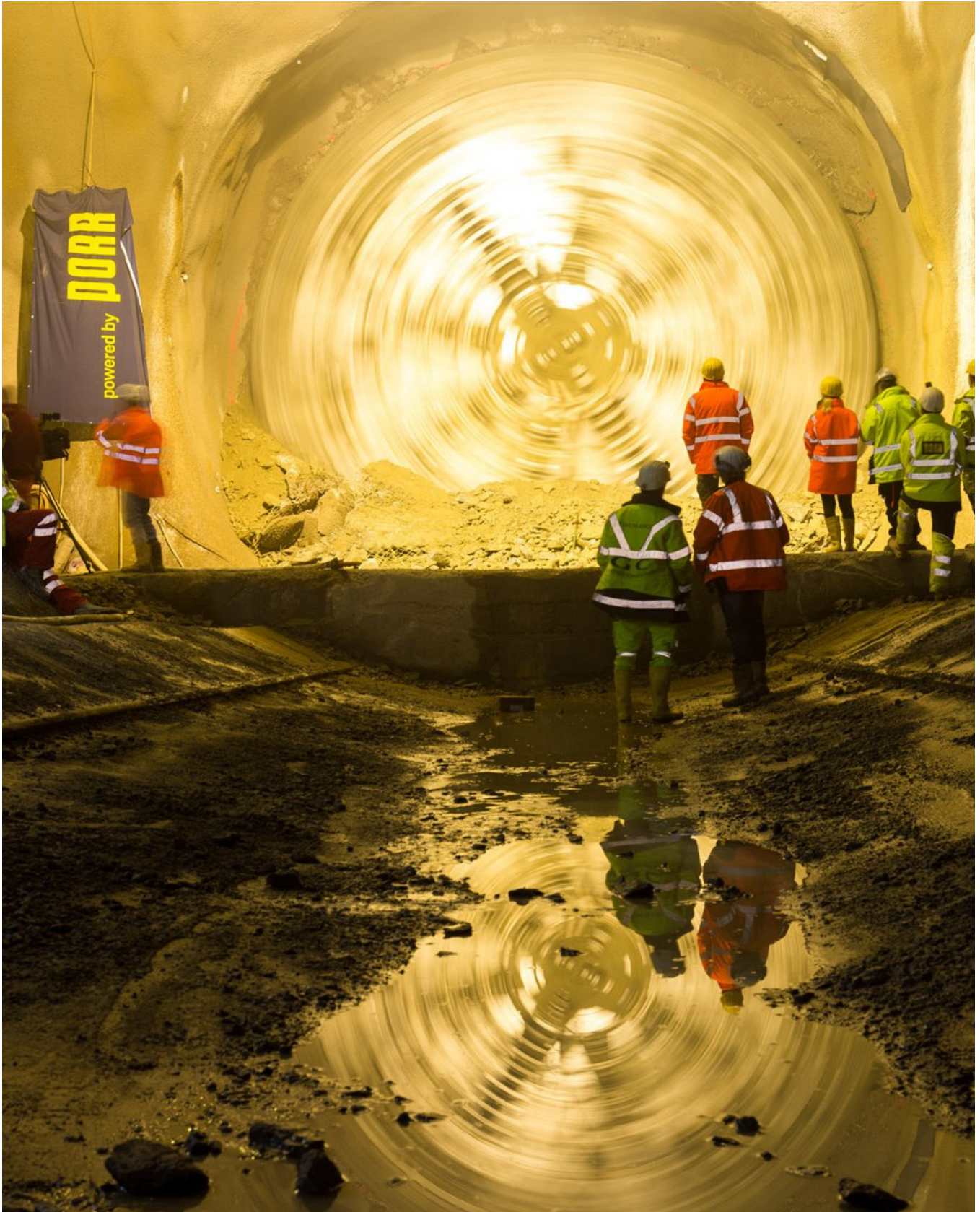
The lining segments in the north tunnel are constructed as a single-skin finish. Source: Harry Schiffer
