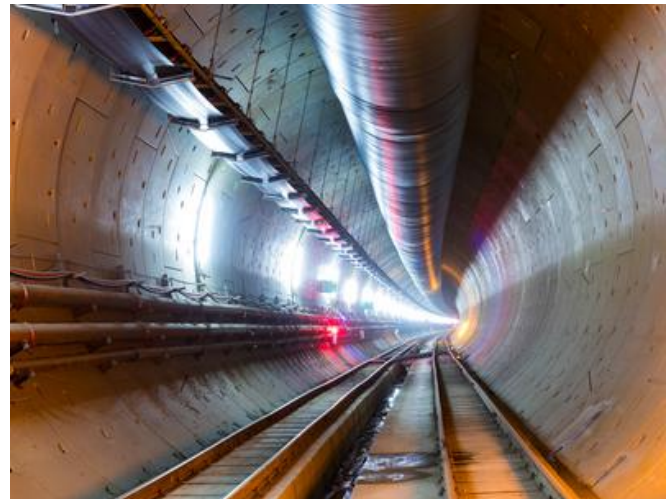
The north tunnel is mainly being bored using the “KORA tunnel boring machine”. Source: Harry Schiffer
