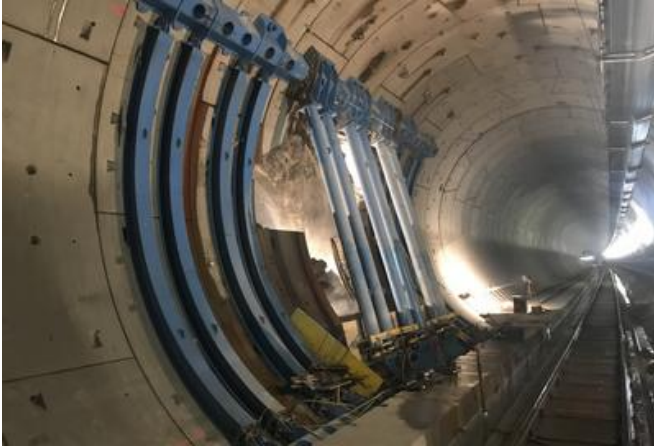
Before breaking through for the cross sections, the lining segments in the Neogene zone were shored up with steel reinforcement. Source: PORR AG
