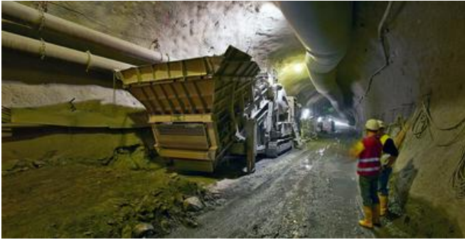
The excavated material from the drilling & blasting was processed on-site by a crusher and transported away via a conveyor system. Source: Toni Rappersberger
