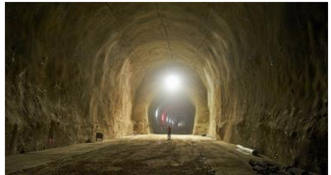
Dismantling cavern in the south tunnel, with a full-face cross-section of 170m 2 , looking towards Klagenfurt in the direction of the rail tunnel advance. Source: Toni Rappersberger
