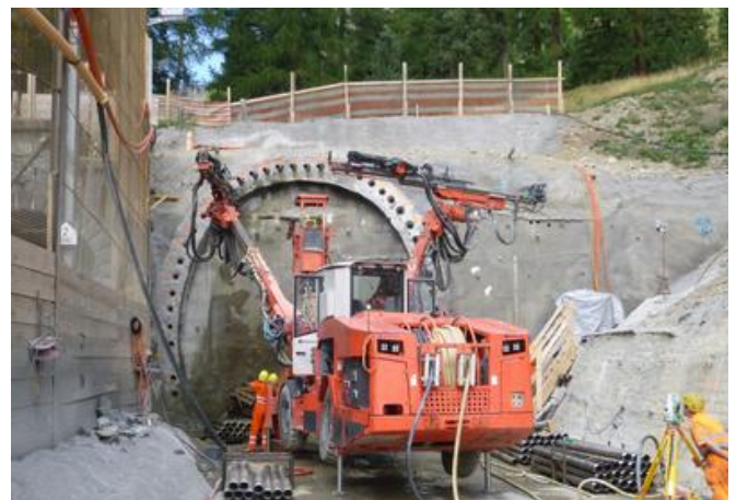
The railway line in Spinass continued operating during the pipe screen advance. Source: PORR
