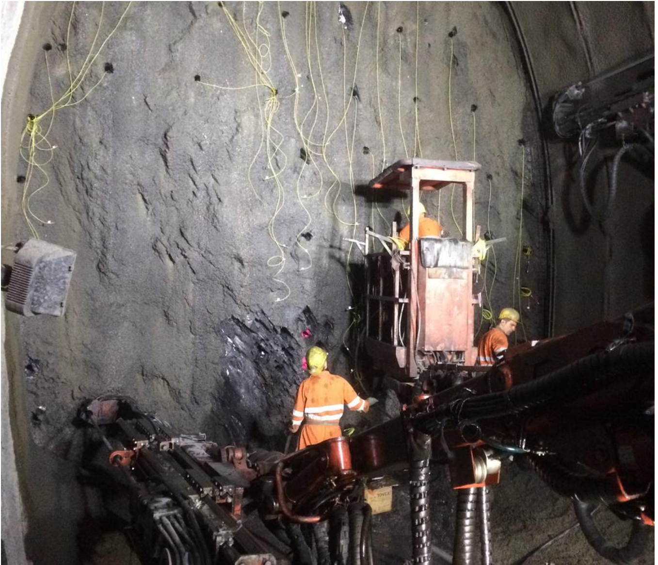
In the Allgäu schist section, it was possible to switch to drilling and blasting, but the dark fine slate proved to be very loose, with a tendency to form silt. Source: PORR
