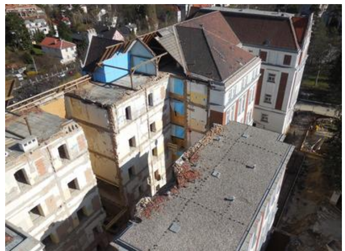
A view from the crane cab shows the vast scope of the structurally challenging demolition work. Source: PORR
