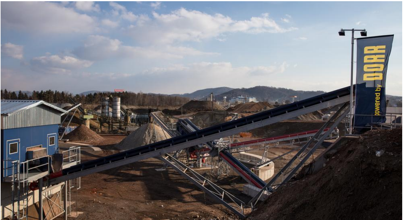
The Pirka recycling plant was constructed in just six months. Source: Daniel Ulbricht-Sundt
