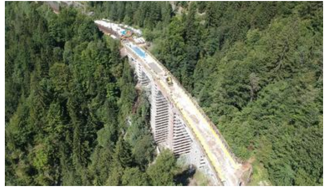
The entire frame had to be rehabilitated within a two-week track closure period in August. Source: PORR
