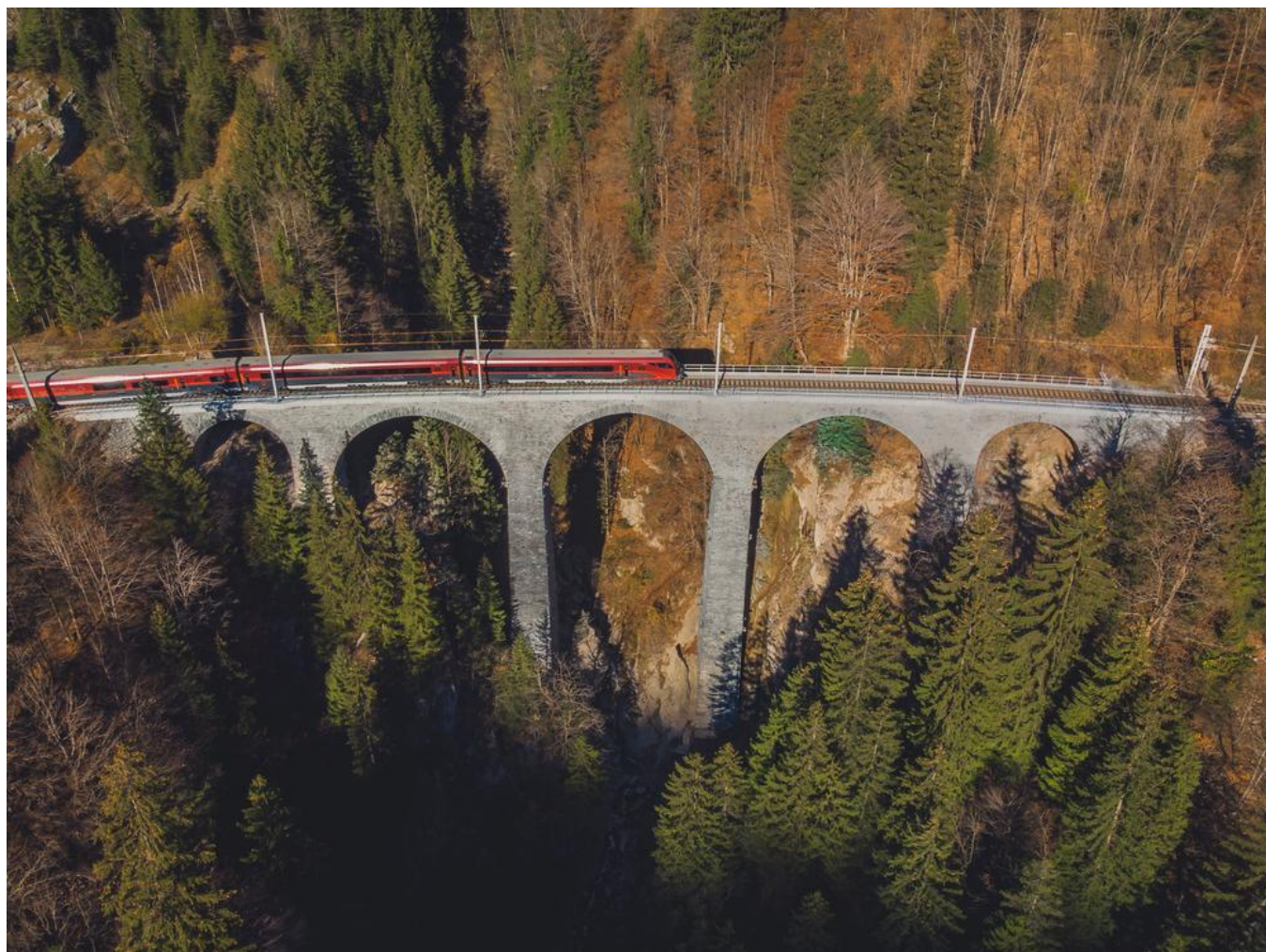
The project was handed over to the employer in October 2018. Source: ÖBB
