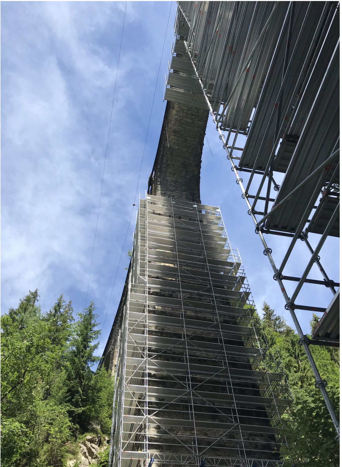
Using a rope crane to scaffold the pier. Source: PORR
