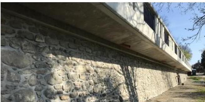
The bridge's foundation is made up of natural stone masonry. Source: PORR
