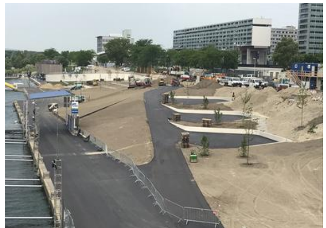
PORR erected several retaining walls featuring irregular curves along the embankment area. The largest retaining wall begins at the quay and ends at the top of the embankment (visible in the background). Source: PORR
