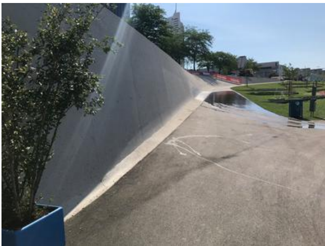
Custom-made formwork was needed to produce the exposed concrete surfaces. Source: PORR
