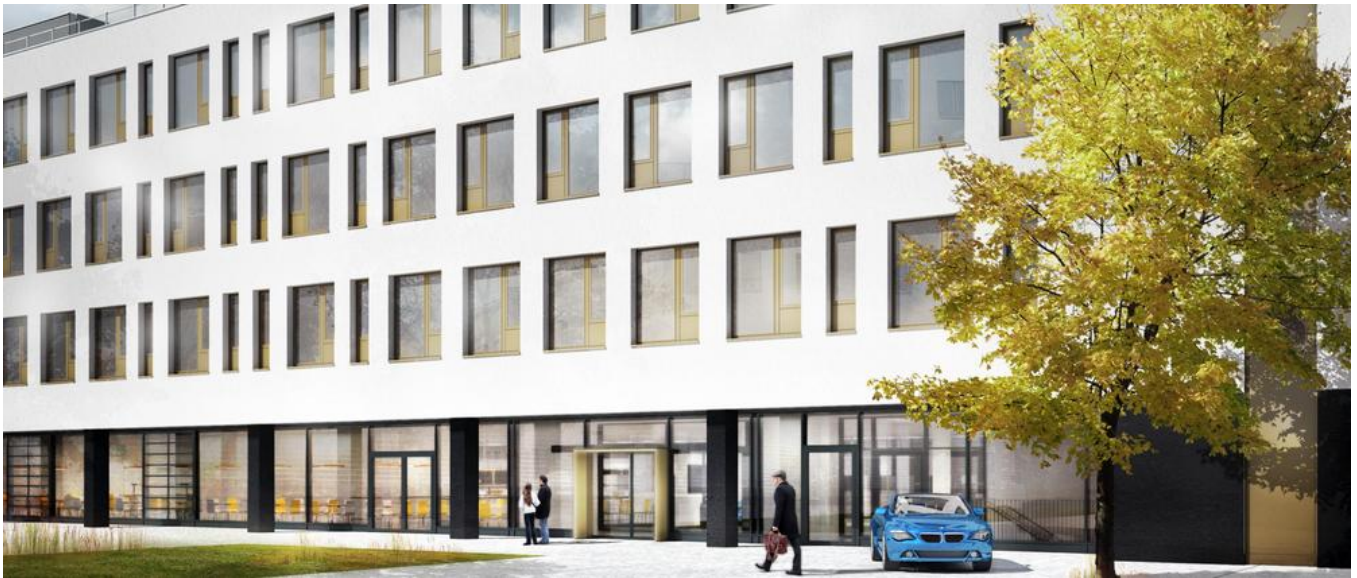
The area outside the main entrance, as well as the foyer, is intended to contain vehicle display areas. Source: PORR Design & Engineering
