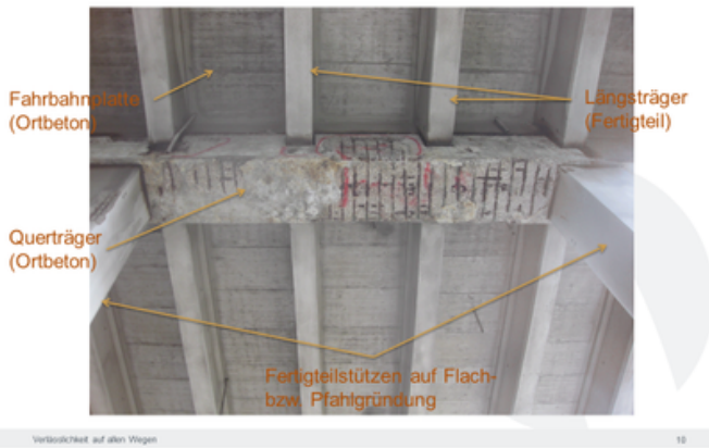
The steep increase in lorry traffic and prolonged use of road salt have resulted in irreparable damage. Source: PORR
