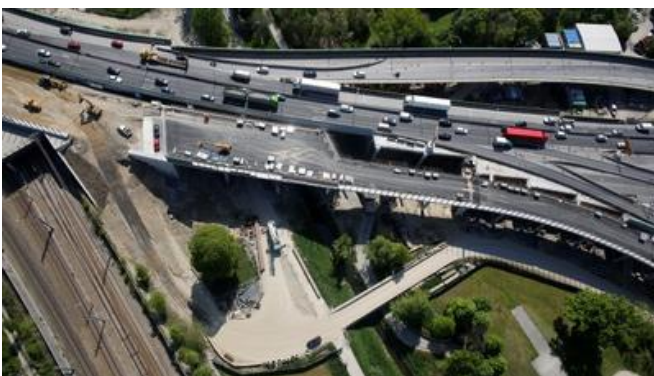
Several bridges were completely or partially rebuilt and an existing tunnel was backfilled. Source: PORR
