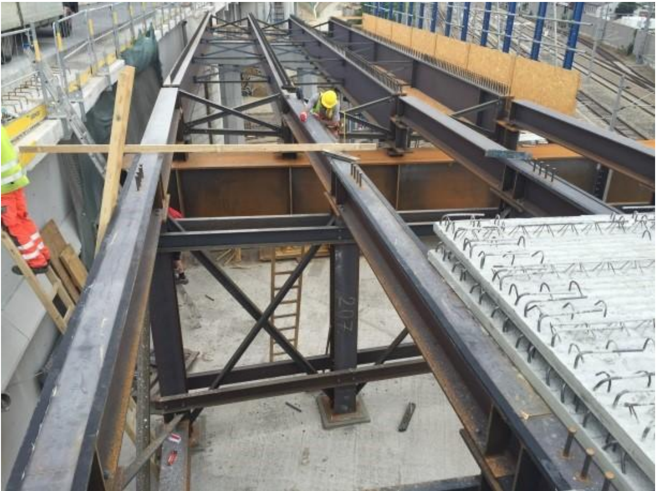
To create space for the construction site facilities and maintain ongoing traffic, the lanes were temporarily widened with the aid of composite steel bridges. Source: PORR
