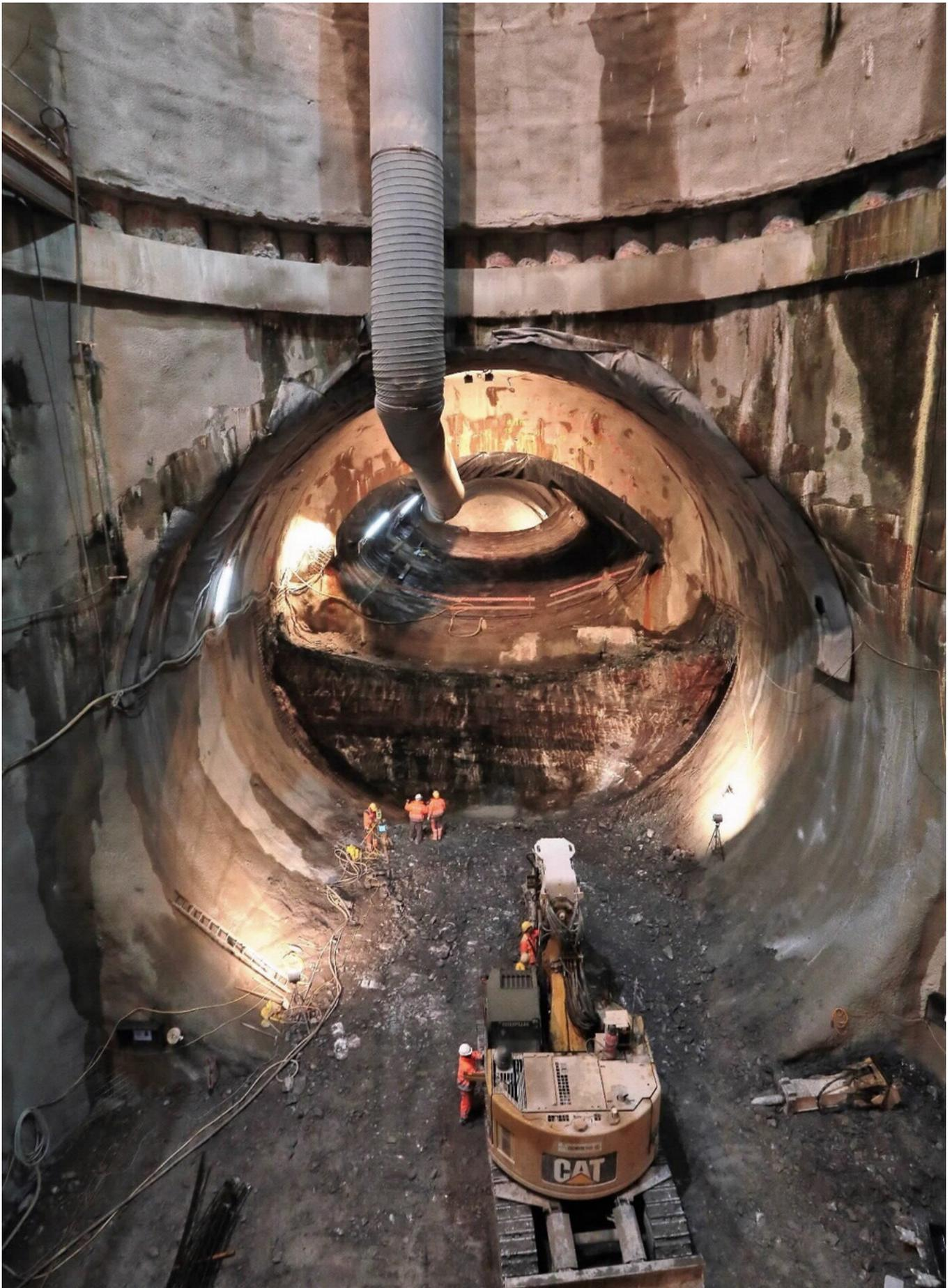
The only tunnel access for the twin-tube tunnel to the new underground station is via a 37m deep shaft and a 110m long access tunnel.
