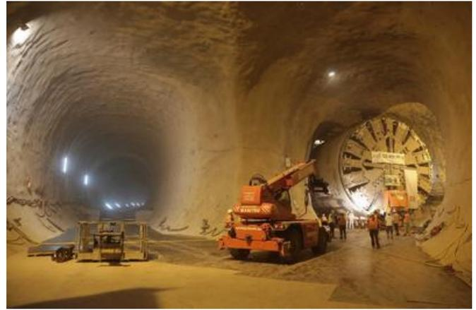
The rotation of the shield section through the turning cavern was particularly spectacular. Source: ATCOST21
