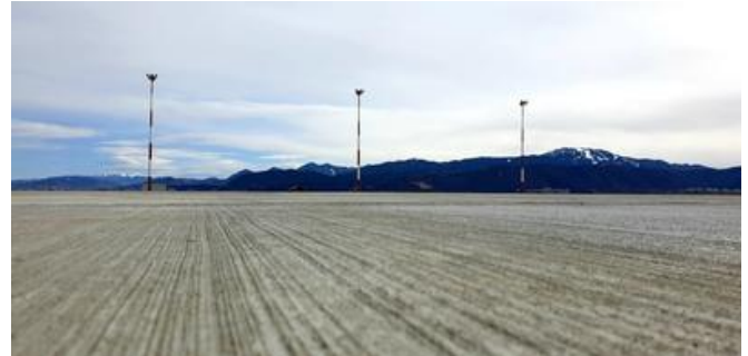
PORR built a high-mast lighting system at the edge of the platform. Source: PORR Construct
