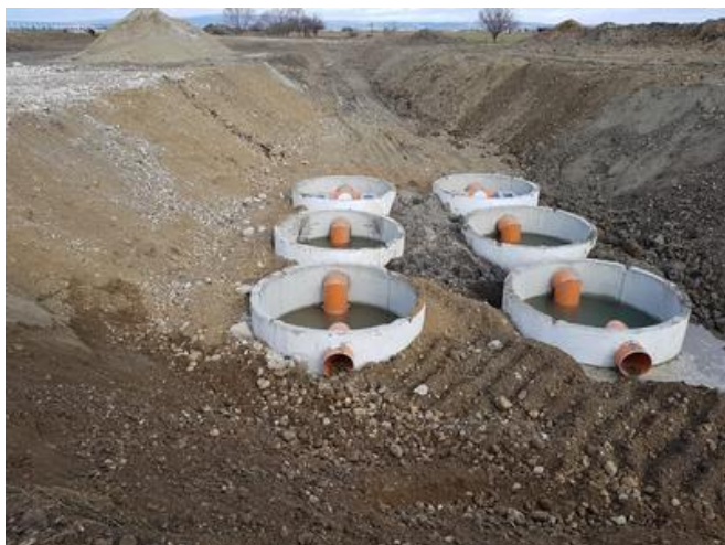
Water is cleaned in the two-stage oil separator system. Source: PORR Construct
