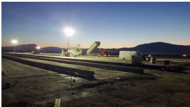
Solid steel girders were used as formwork for the concrete layer. Source: PORR Construct
