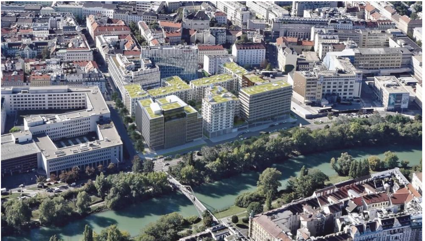
The Laendyard residential complex is part of the “Laendyard” project development area on the Danube Canal in Vienna. Source: Laende3
