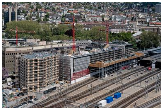
View across the tracks to the Gleisarena and protective tunnel. Source: PORR
