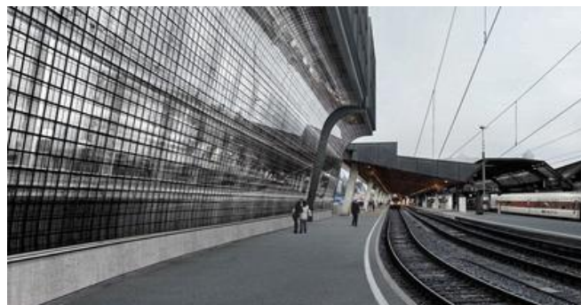
The spectacular curved glass brick facade of the Gleisarena was developed in-house by PORR. Source: PORR
