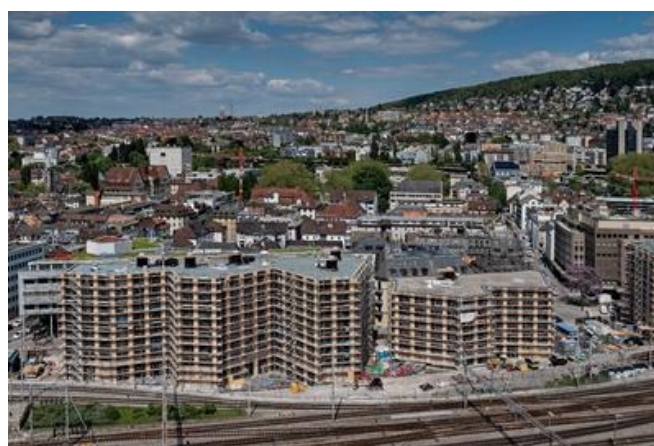
The Gleistribüne complex shortly before completion. Source: PORR
