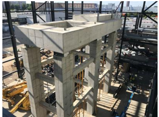
The completed turbine platform. Source: PORR/Fabian Hemauer
