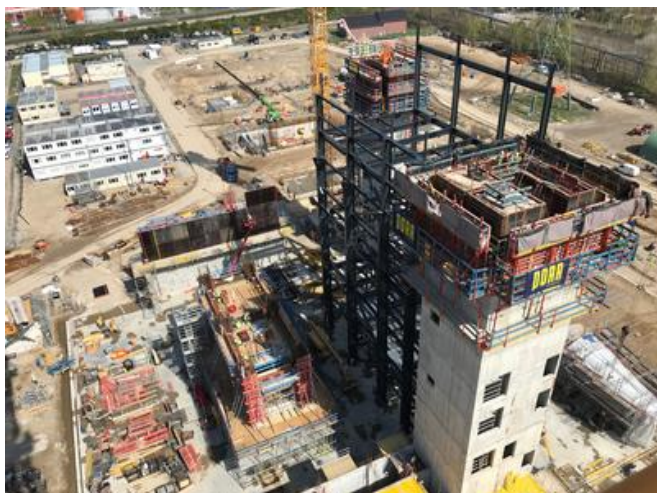
In an effort to meet weekly deadlines, the stairwells had to be heated and coated in frost protection mats over the weekends. Source: PORR/Fabian Hemauer
