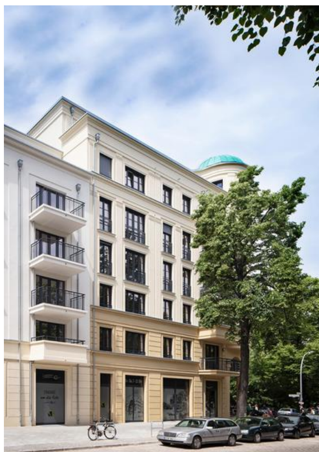
The copper roof dome makes the residential project a special eye-catcher. Source: PORR/Markus Löffelhardt
