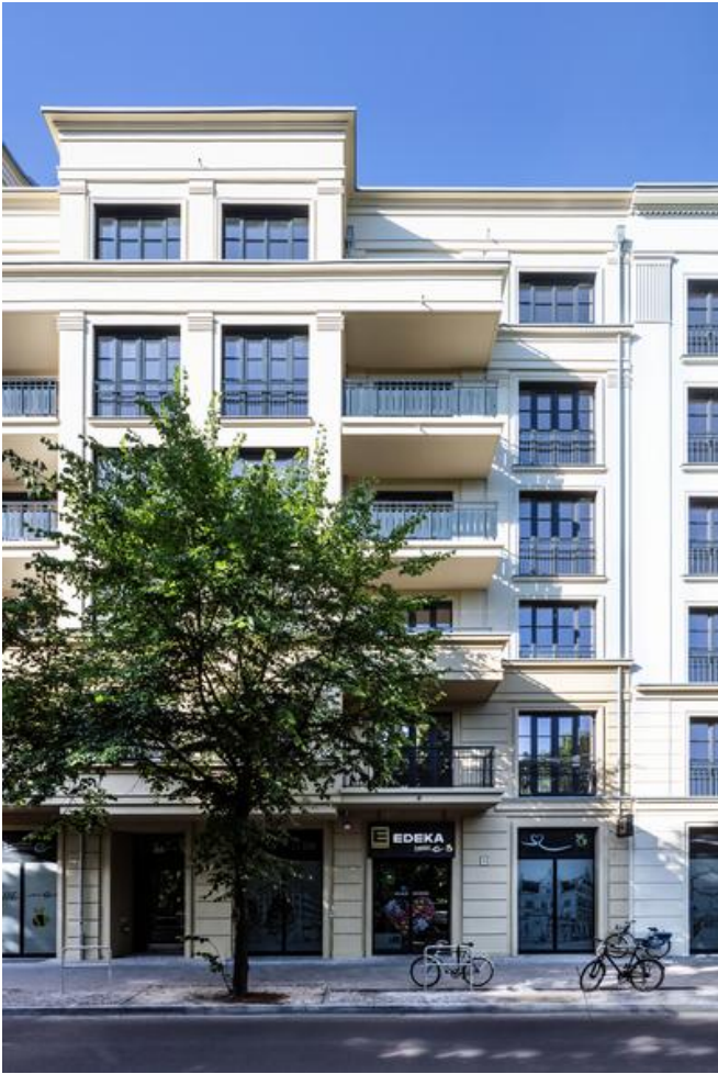
The elaborate façade design has differentiated structures depending on the equipment level. Source: PORR/Markus Löffelhardt
