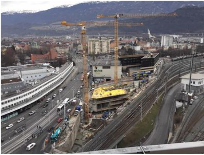
The tracks closest to the construction site were taken out of service for two months. During this time, PORR constructed the storeys from ground level up to third floor. Source: PORR Bau GmbH
