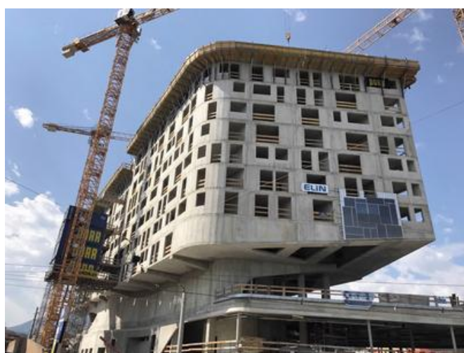
The projecting architecture makes PEMA 2 truly eye-catching. Source: PORR Bau GmbH
