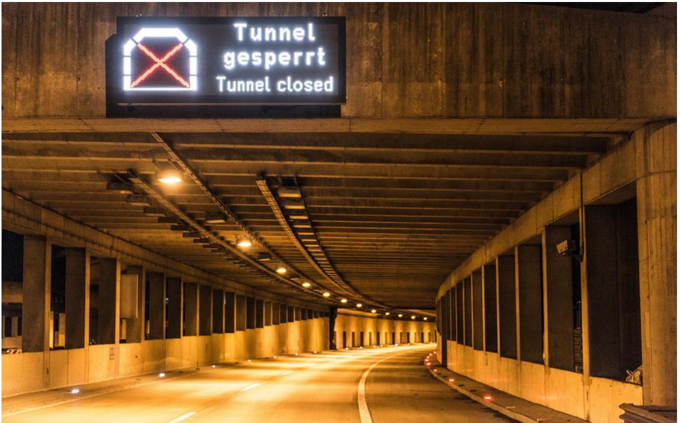
The night closure periods from 8 p.m. to 5 a.m. resulted in a net working period of only six hours. An entire round had to be completed within this time window. Source: Thomas Exel
