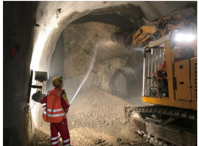
Work was carried out, using only an excavator, for the last few metres before reaching the west tunnel. Source: Thomas Exel
