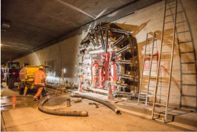
A total of 20 cross passages were constructed, five accessible by vehicle, 15 on foot. Source: Thomas Exel
