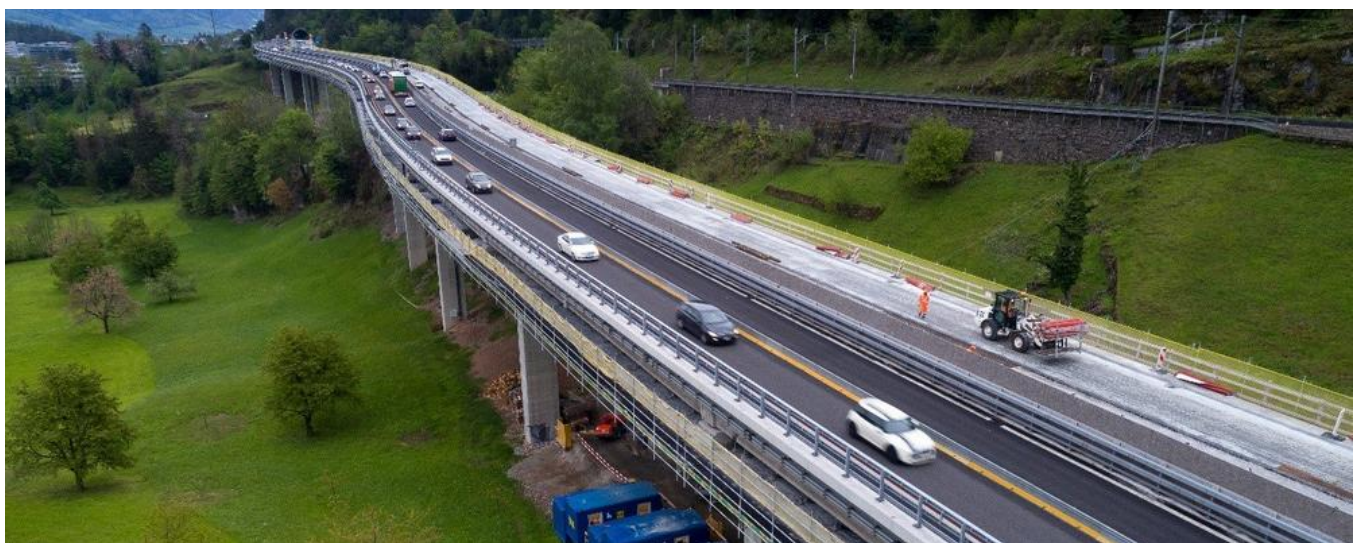
The Linden Bridge with scaffolding below the sides and new parapets. Source: PORR AG
