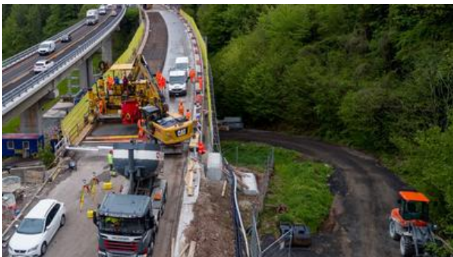
When temperatures during the day were high, work to apply the ultra-high performance concrete (UHPC) had to begin as early as 4am. Source: PORR AG
