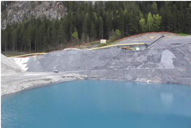
Aggregate material is collected from a side entrance and processed on site. Source: GKI Maria Stein consortium
