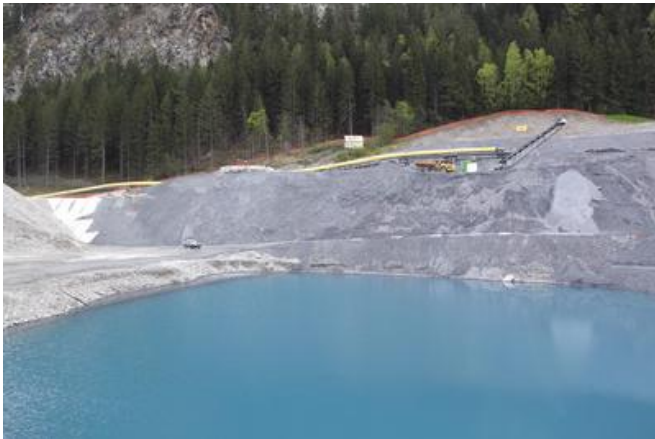
Aggregate material is collected from a side entrance and processed on site. Source: GKI Maria Stein consortium
