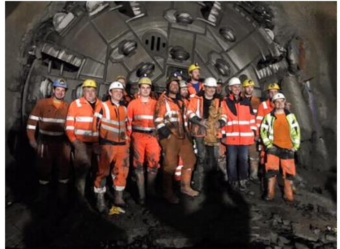
The northern section of the headrace tunnel was the first to be broken through, in April 2019. Source: GKI Maria Stein consortium
